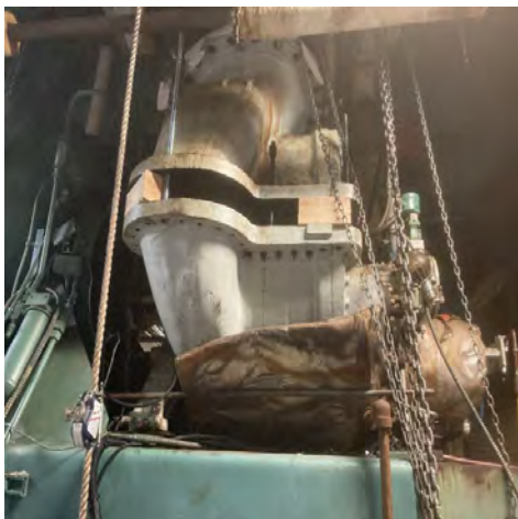
Turbine Cap Jacked, Splitline Separated
