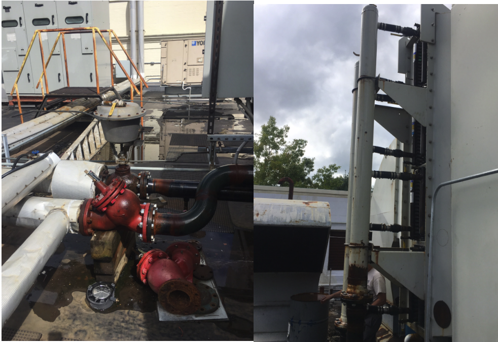
Image 7 - Image of turbine inlet air cooling coil and control valve (actuator disconnected)
