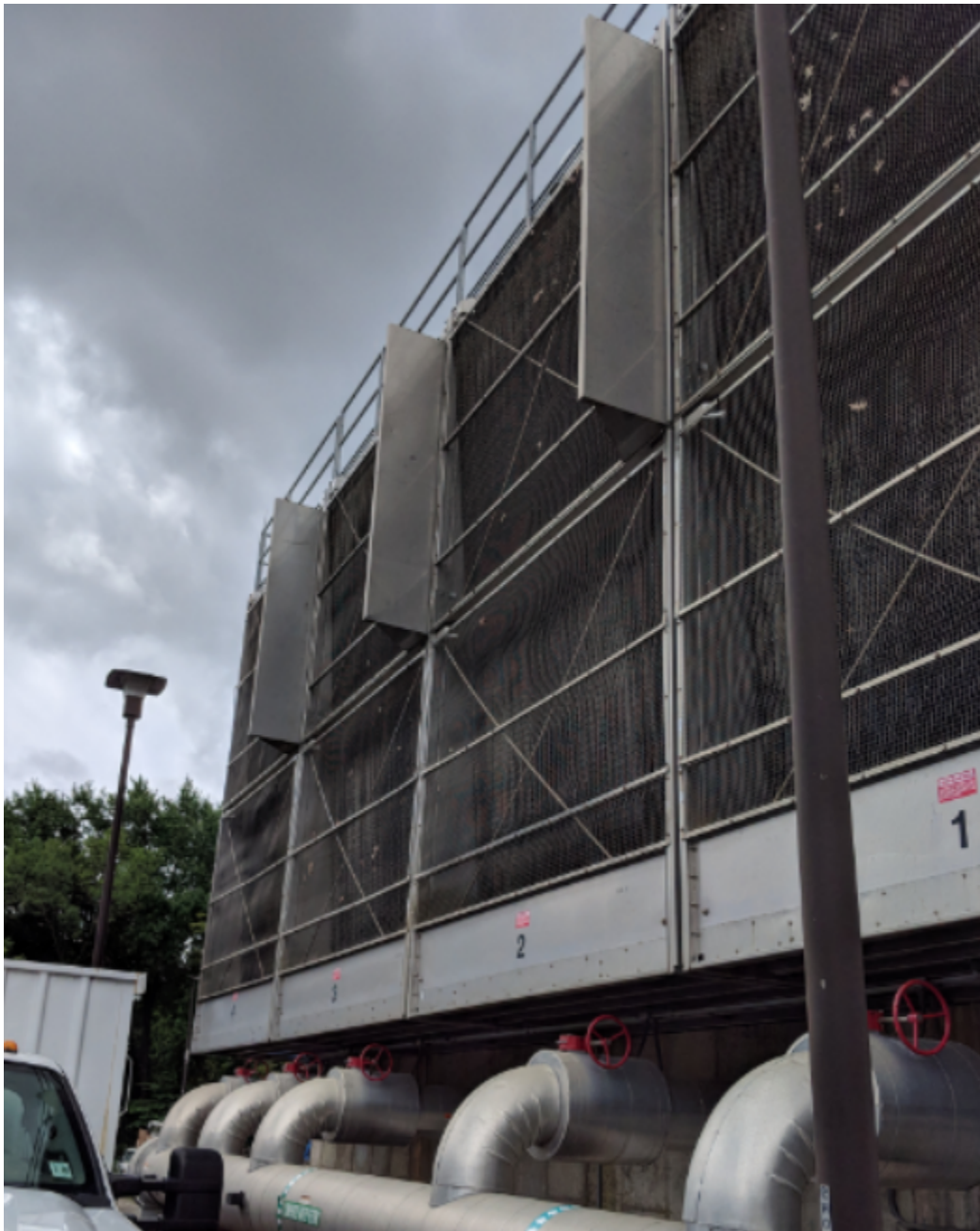
Image 11 – Chiller Plant Cooling Towers
