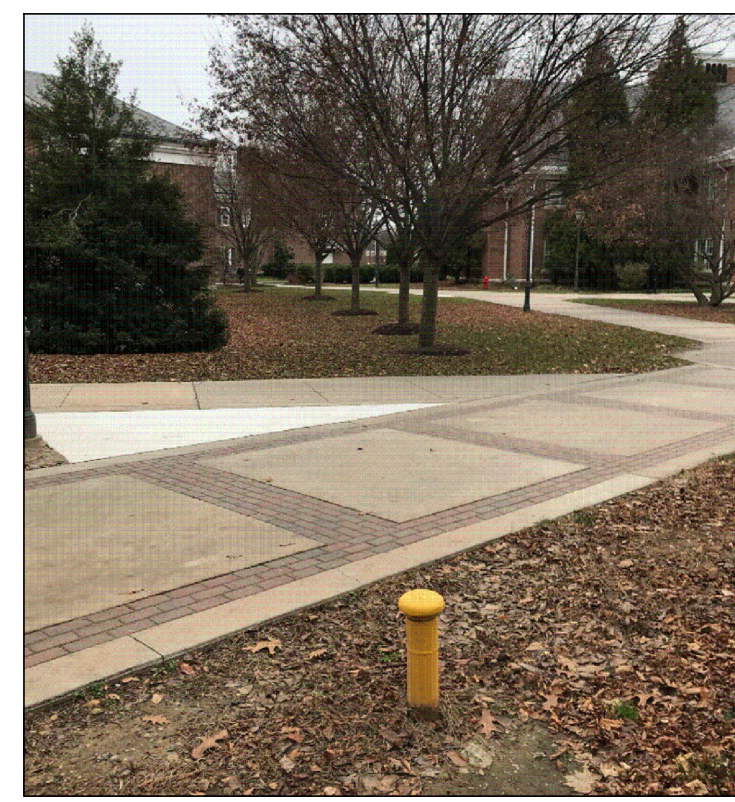
PHOTO B - MANHOLE 15A TO 16A Area For New Duct Bank Routing From Manhole 15A To Manhole 16A Includes Hardscapes Such As Brick And Concrete
