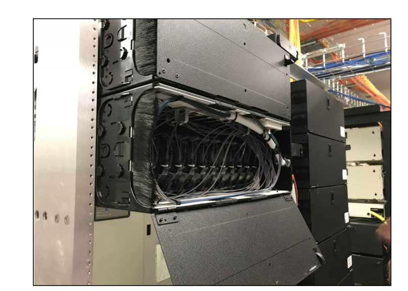
RACK MOUNTED CABINET
