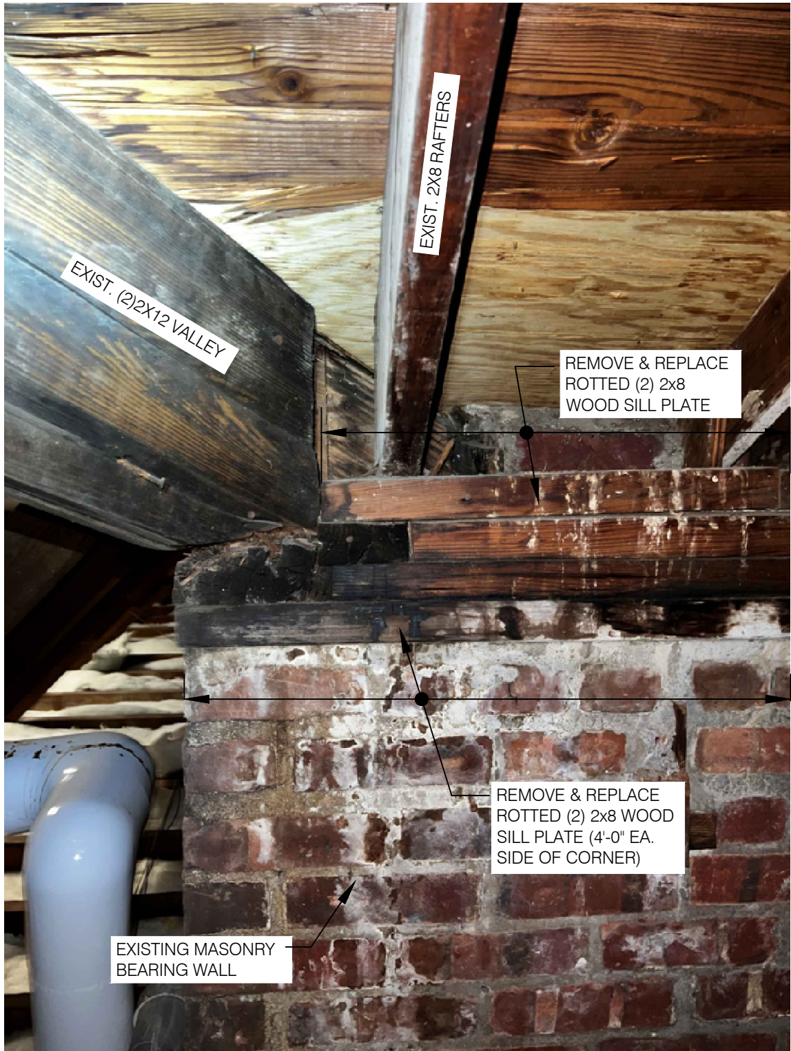
DETAIL B/104 ROOF VALLEY REPAIR NO SCALE
