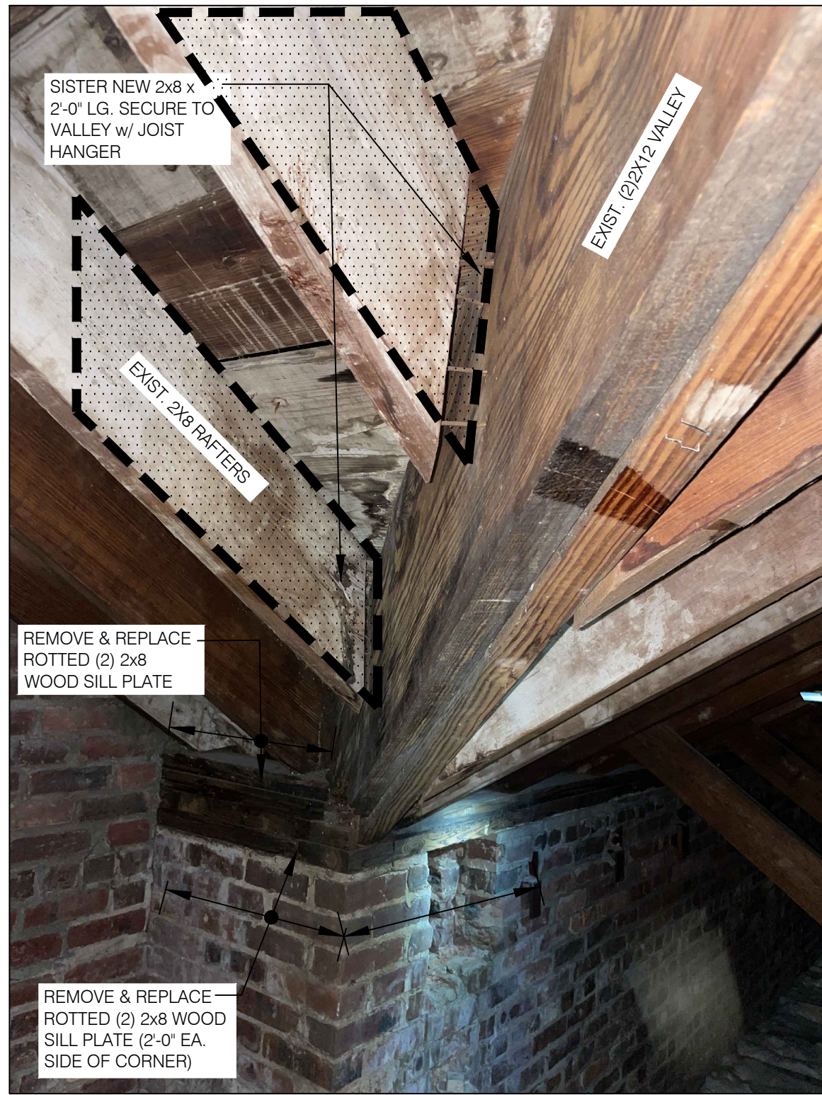
DETAIL A/104 ROOF VALLEY REPAIR NO SCALE
