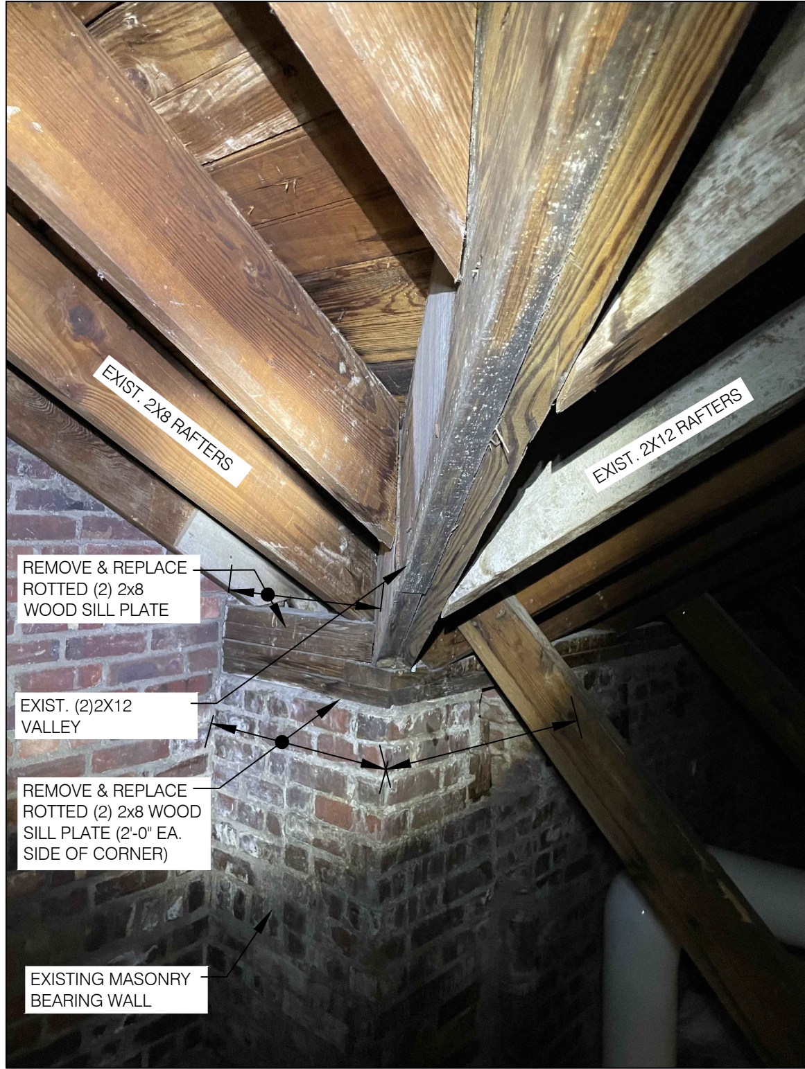
DETAIL A/104 ROOF VALLEY REPAIR NO SCALE
