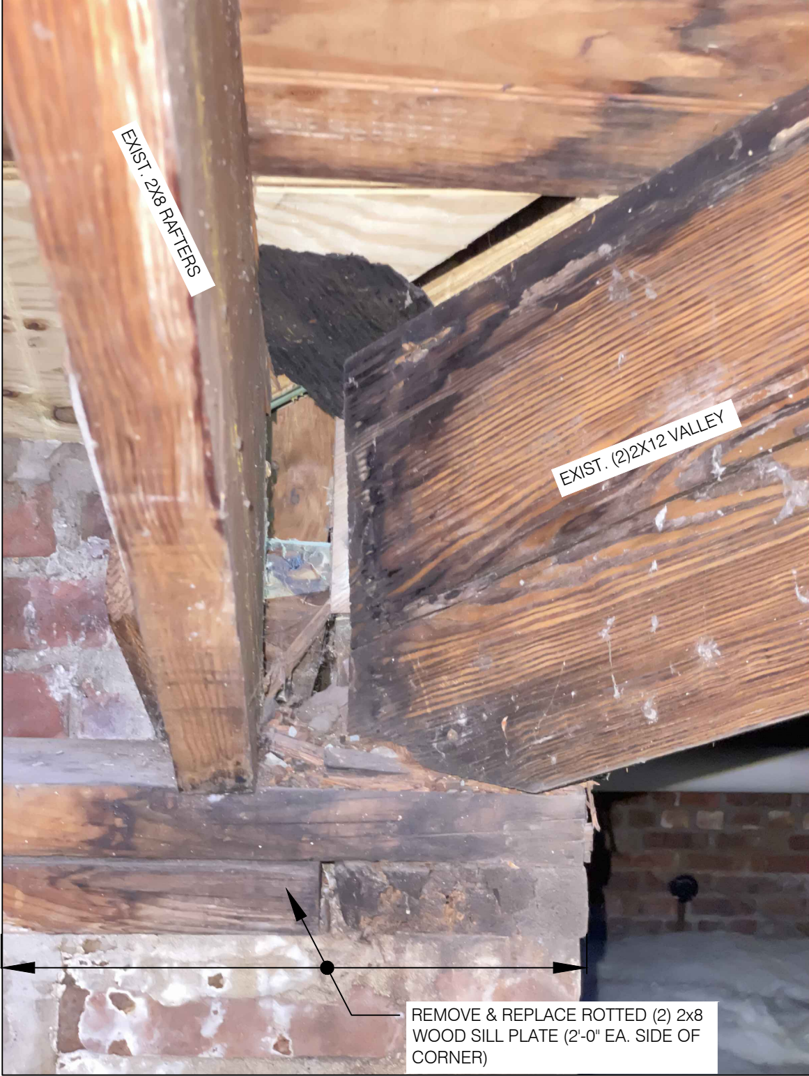
DETAIL C/104 ROOF VALLEY REPAIR NO SCALE
