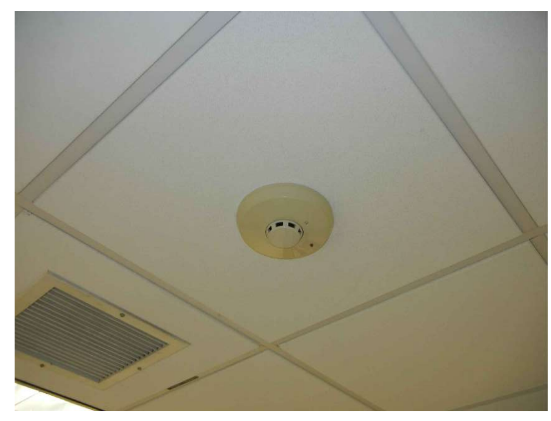
PHOTO B - EXISTING DROP CEILING Route Fiber Pathway Above Existing Drop Ceilings With The Corridor
