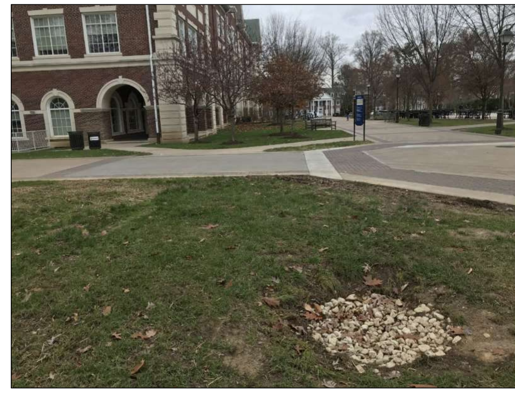
PHOTO D - OUTSIDE NEW LIBRARY Location For New Manhole And Duct Bank Routing From New Library To Green Hall. Route Includes Hardscapes Such As Brick And Concrete.
