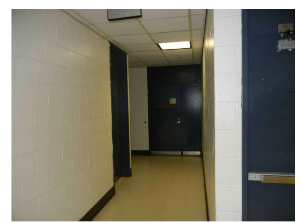
PHOTO B - BASEMENT CEILING Route Fiber Pathway Above Existing Basement Drop Ceiling
