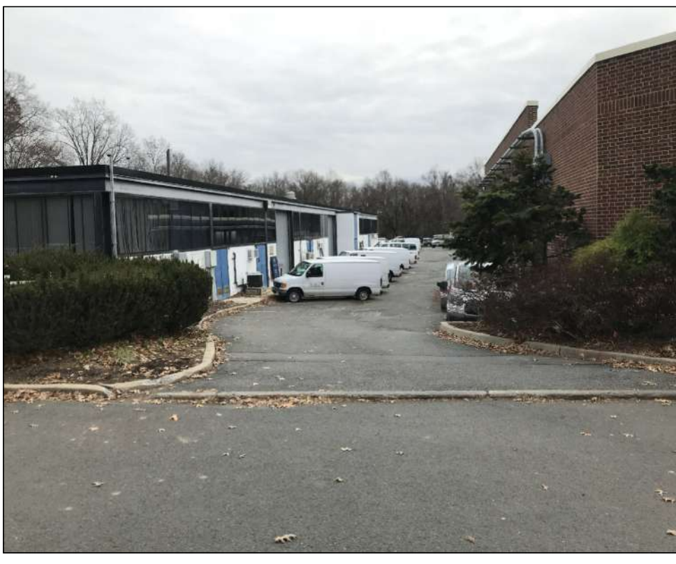
PHOTO A - MAINTENANCE BUILDING TO POWER HOUSE Location For New Duct Bank And Fiber Between The Maintenance Building And The Power House. Route Includes Hardscapes Such As Brick And Concrete.
