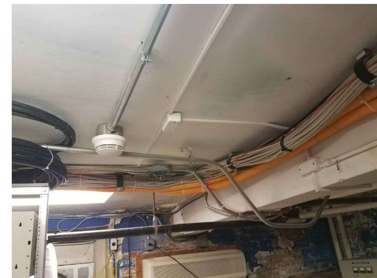
PHOTO B - BASEMENT CEILING Existing Ceiling Space In Basement MDF.
