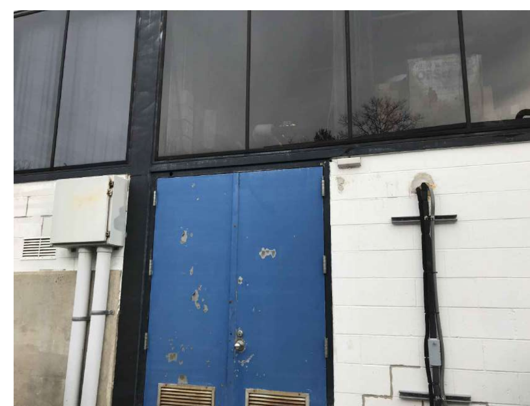
PHOTO D - EXISTING POINT OF ENTRY Location Of Existing Point Of Entry For Maintenance Building Pull Box Mounted On Building Exterior With Empty Conduit.
