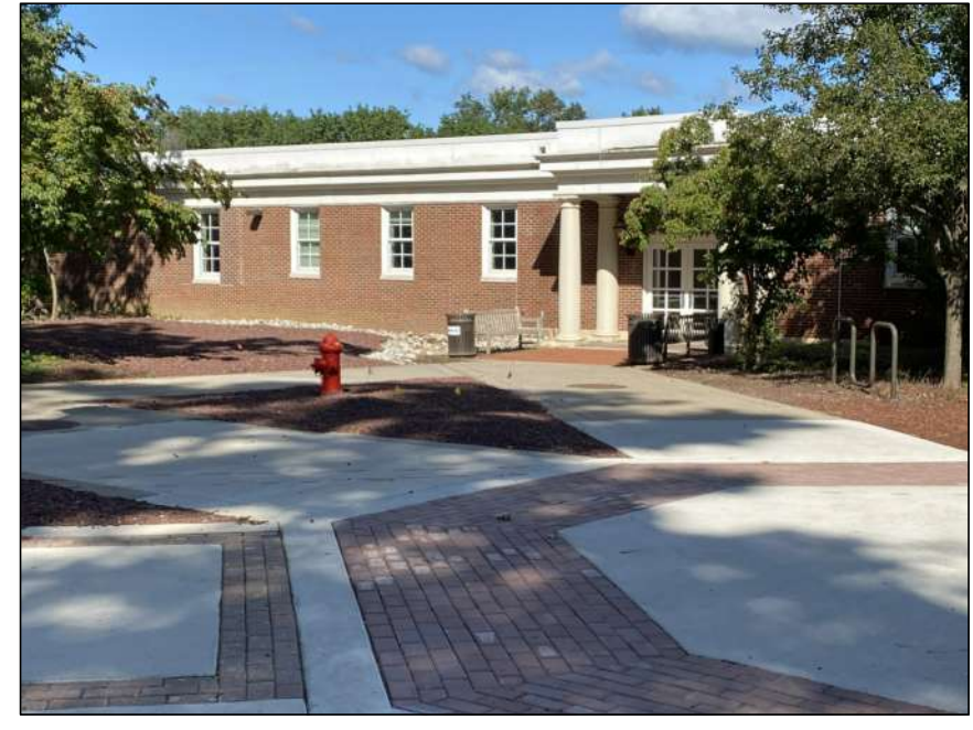
PHOTO A - ARMSTRONG HALL EXTERIOR Area Outside Armstrong Hall In Location Of Exterior Pull Box For Building Point Of Entry
