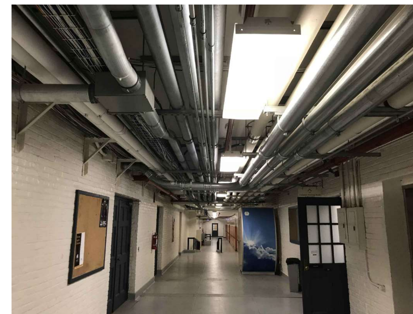
PHOTO A - BASEMENT CEILING New Fiber In Conduit To Be Run Along Basement Open Ceiling.
