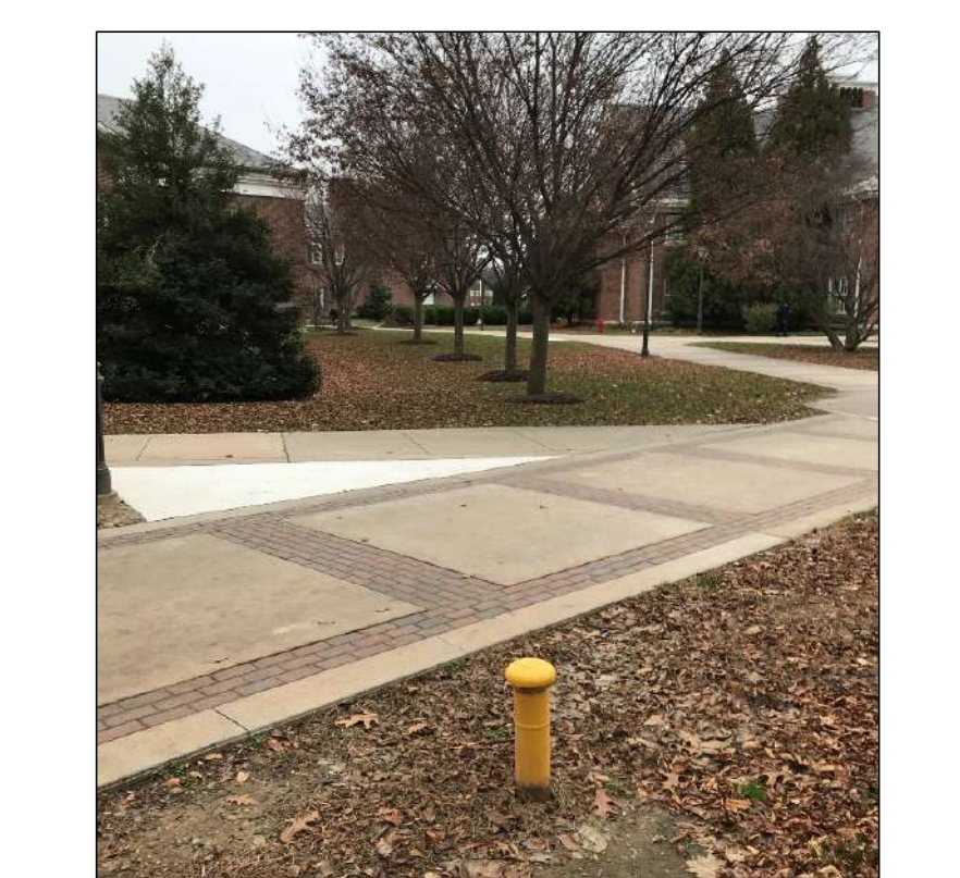
PHOTO B - MANHOLE 15A TO 16A Area For New Duct Bank Routing From Manhole 15A To Manhole 16A Includes Hardscapes Such As Brick And Concrete
