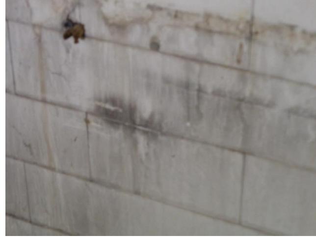
Photo 23. Suspect Mold Growth in Room 110.
