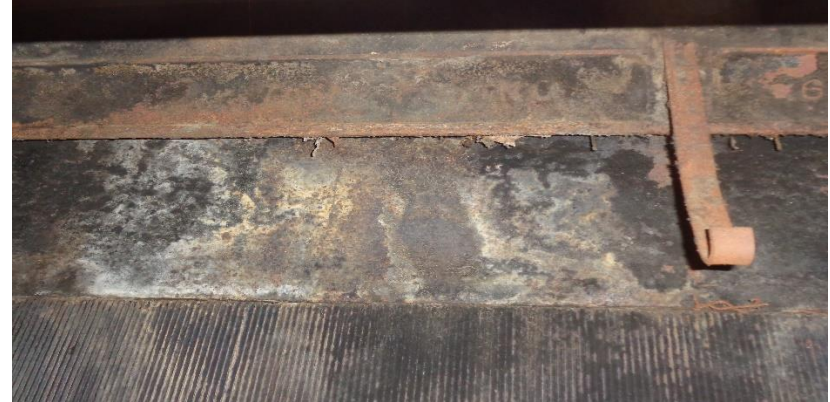
Photo 39a. Suspect Mold Growth inside the Fire Place in Room 108.
