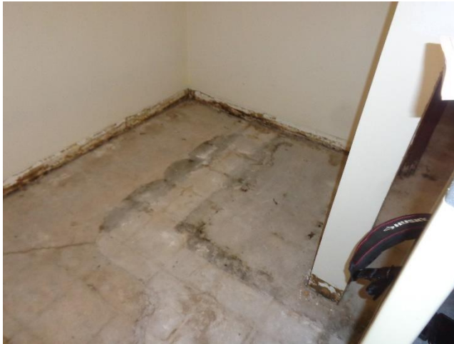
Photo 6. Suspect Mold Growth on the Concrete Floor of Room 002a.
