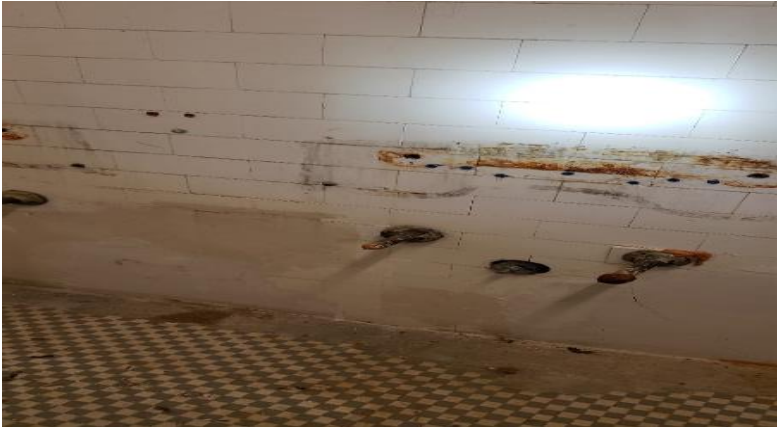
Photo 53. Suspect Mold Growth in Room 212.
