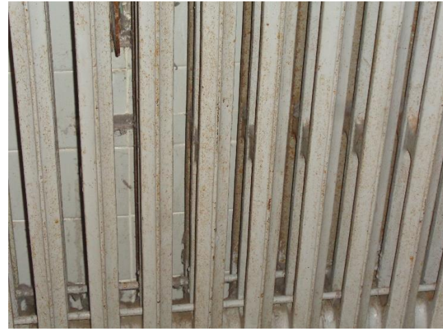
Photo 24a. Suspect Mold Growth on the Radiator in Hallway H101.
