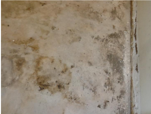
Photo 3. Suspect Mold Growth on the Concrete Floor of Room 003a.
