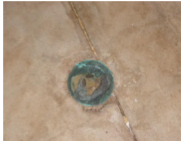
Photo 12a. Suspect Mold Growth on the Sealed Pipe Drain Located on the Southwest Floor of Room 017.
