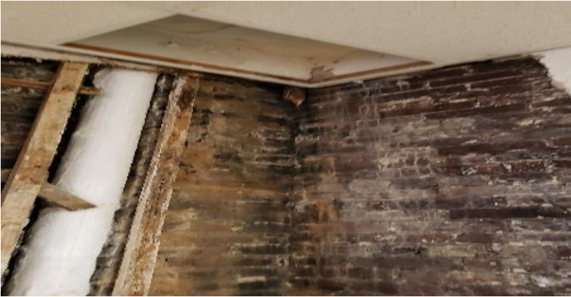
Photo 49. Northwest Corner Suspect Mold Growth from Ceiling to Floor in Room 208.
