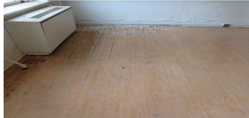
Photo 41a. Suspect Mold Growth on the Floor at the Southeast Corner of Room 201.
