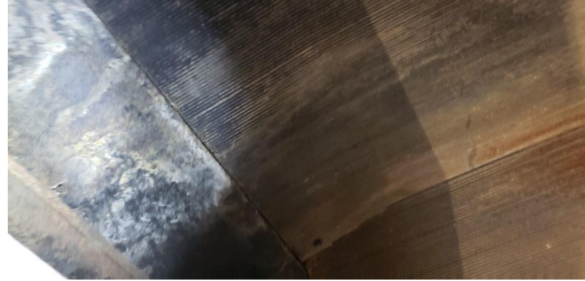
Photo 39. Suspect Mold Growth inside the Fire Place in Room 108.
