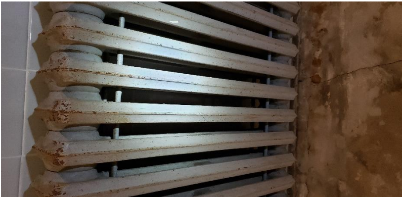
Photo 48. Suspect Mold Growth on the Radiator in Hallway H201. Ceiling in Room 206.
