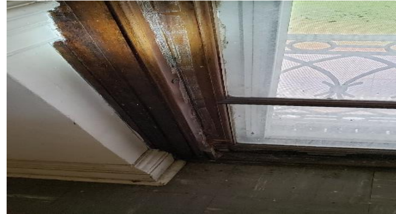
Photo 55. Suspect Mold Growth around the Window in Room 213.
