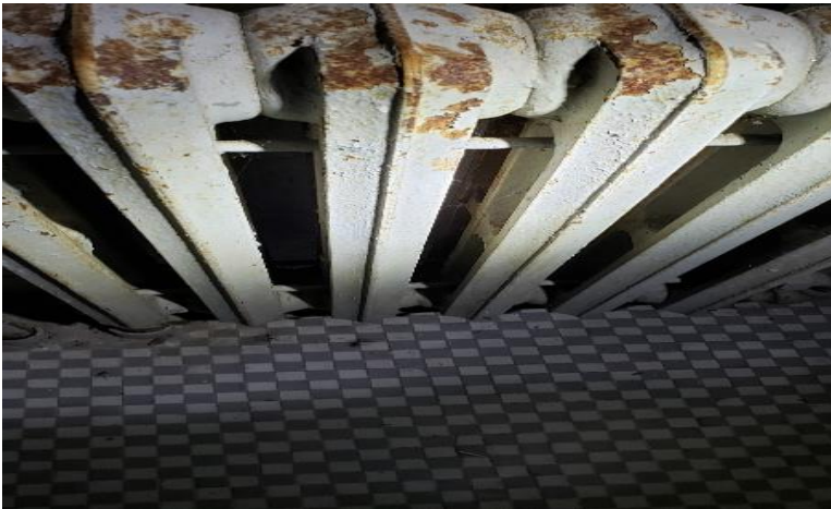
Photo 36. Suspect Mold Growth on the Radiator in Room 104.
