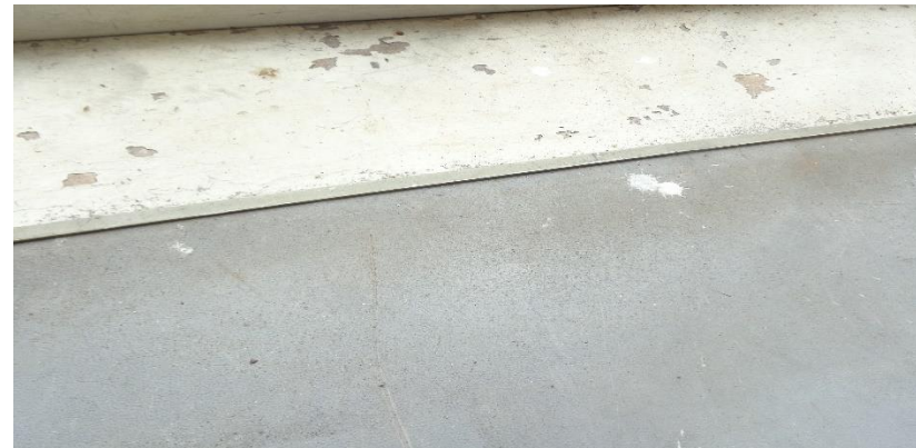
Photo 44a. Suspect Mold Growth on the Eastern Window of Room 203.
