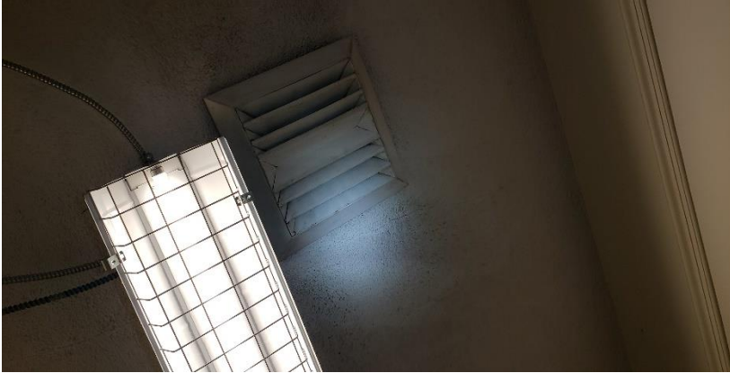
Photo 59. Suspect Mold Growth on the Vent by the Ramp near Rooms 213 and 214.
