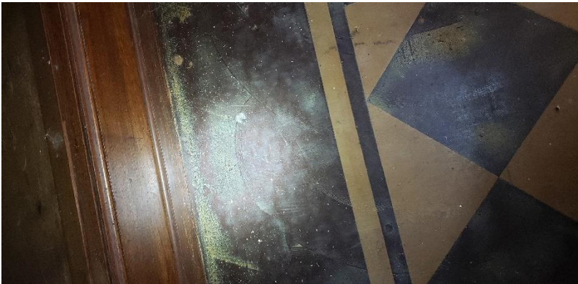
Photo 38. Suspect Mold Growth on the Ground along the Eastern Wall in Room 108.
