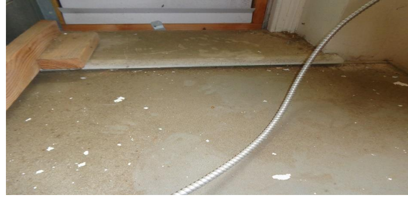
Photo 45a. Suspect Mold Growth in the Northeast Corner of Room 205.
