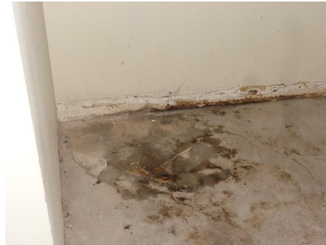
Photo 2a. Suspect Mold Growth on the Concrete Floor of Room 003a.
