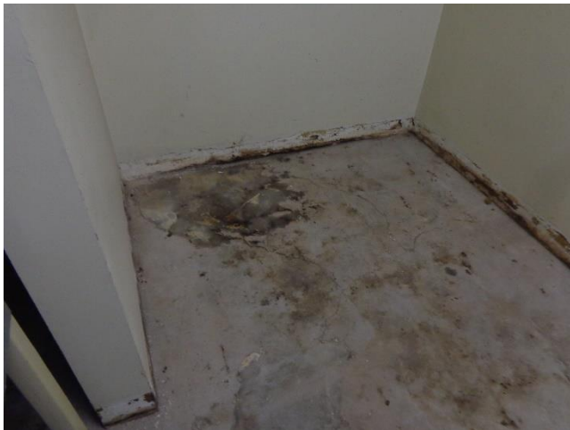
Photo 2. Suspect Mold Growth on the Concrete Floor of Room 003a.
