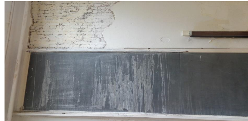
Photo 42a. Suspect Mold Growth on the South Wall in Room 201.
