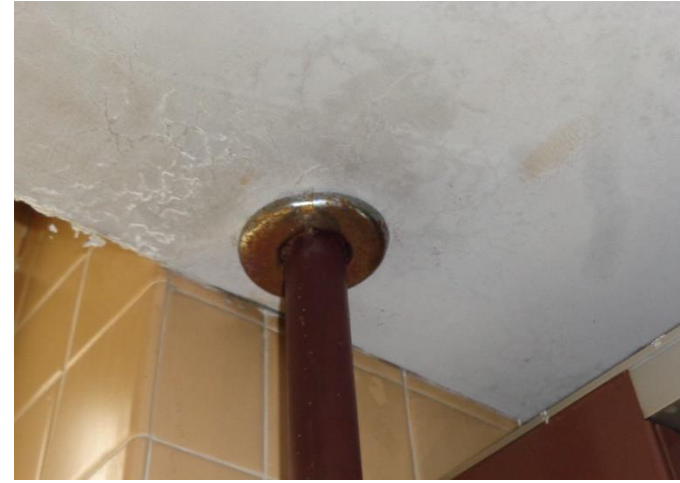
Photo 5. Suspect Mold Growth on the Eastern Ceiling in Room 002
