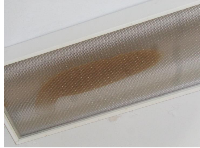
Photo 26a. Suspect Mold Growth on the Northern Light Fixtures of Room 112 has worsened.
