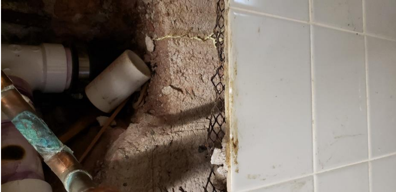
Photo 47. Suspect Mold Growth on the Water Fountain Wall in Hallway H201.
