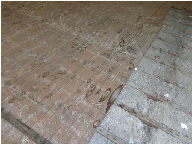
Photo 21. Suspect Mold Growth throughout the Floor of Room 109.
