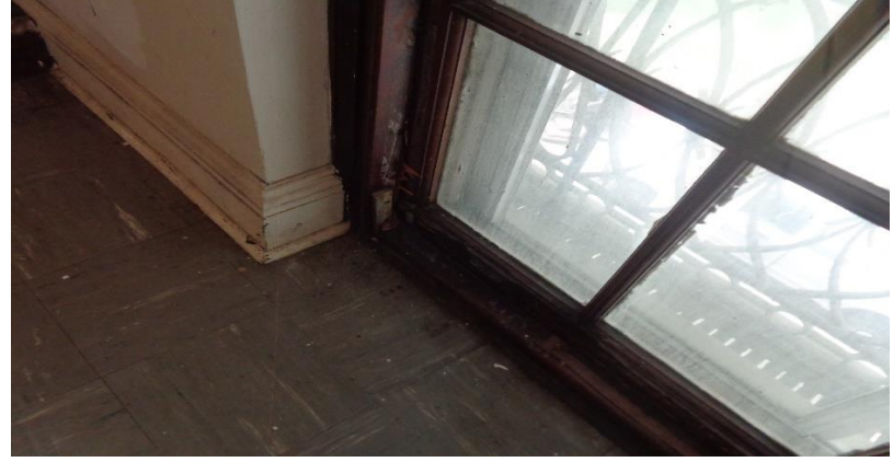
Photo 55a. Suspect Mold Growth around the Window in Room 213.
