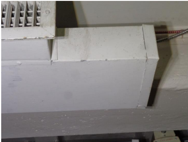
Photo 10. Suspect Mold Growth in the Vents across the Ceiling in Room 017.
