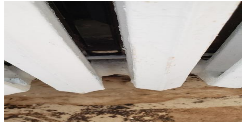
Photo 56. Suspect Mold Growth on the Radiator of Room 214.
