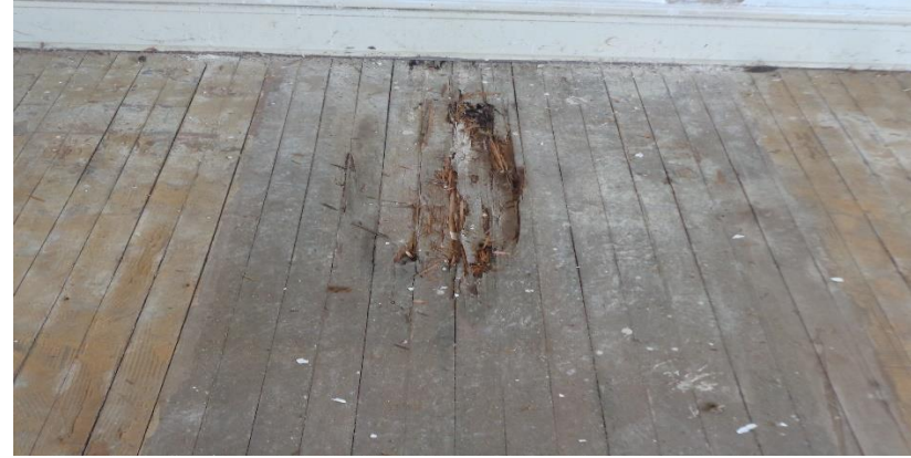
Photo 51a. Suspect Mold Growth on the floor beneath the Western Window in Room 210.
