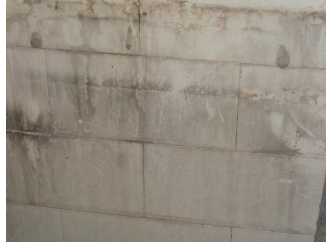
Photo 23a. Suspect Mold Growth in Room 110 has worsened
