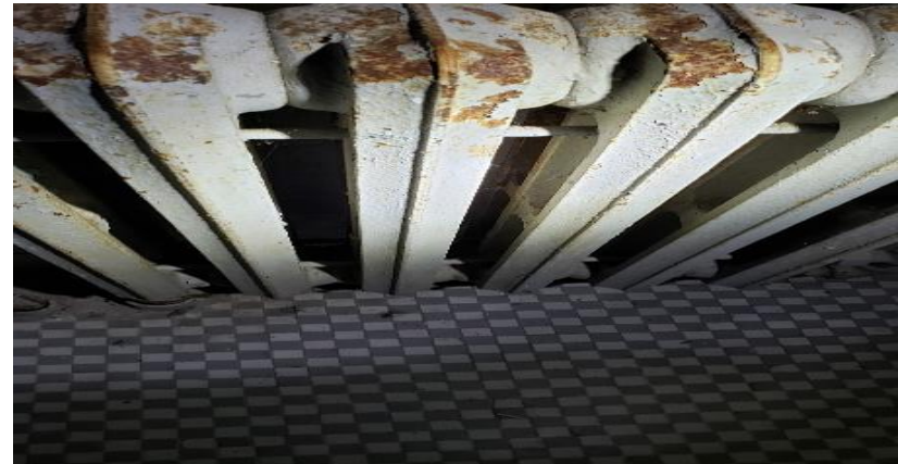
Photo 36. Suspect Mold Growth on the Radiator in Room 104.
