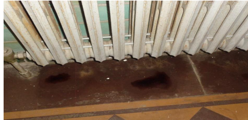
Photo 50a. Suspect Mold Growth on Radiator in Hallway H203.
