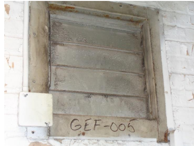
Photo 20a. Suspect Mold Growth on the Vent at the Southeast Corner of Room 016.
