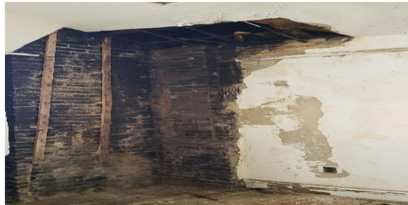
Photo 60. Suspect Mold Growth on the Southwest Corner in Room 218.
