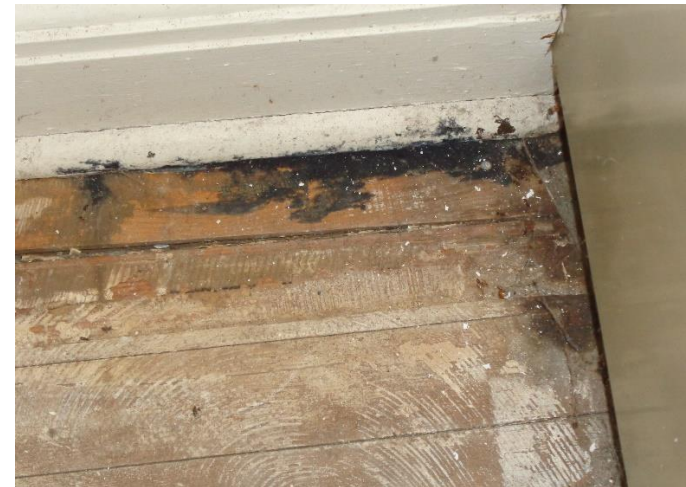
Photo 22a. Suspect Mold Growth in the Southwest side of Room 109.
