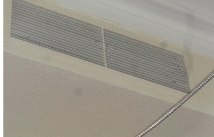
Photo 33a. Suspect Mold Growth on the Vents of Room 106.
