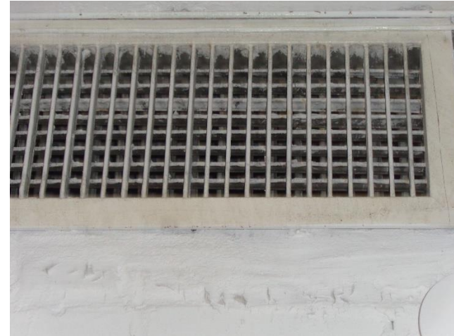
Photo 13a. Suspect Mold Growth in the Vents of Room 018.
