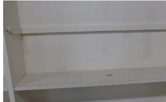
Photo 34a. Suspect Mold Growth on the Bookshelves in Room 102.
