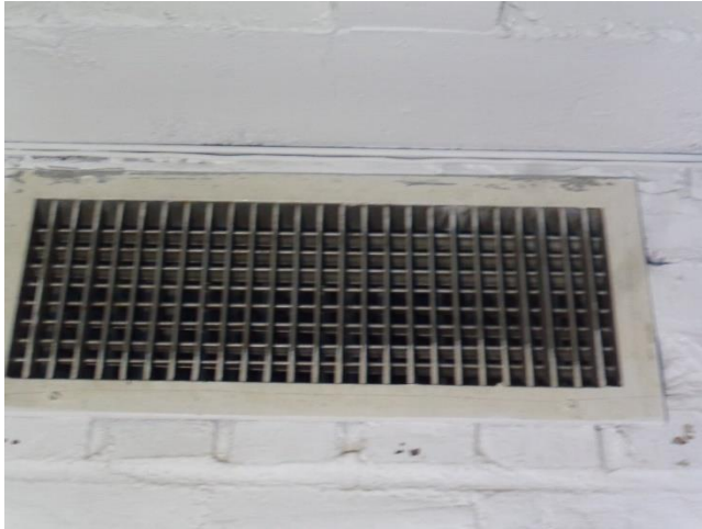
Photo 13. Suspect Mold Growth in the Vents of Room 018.
