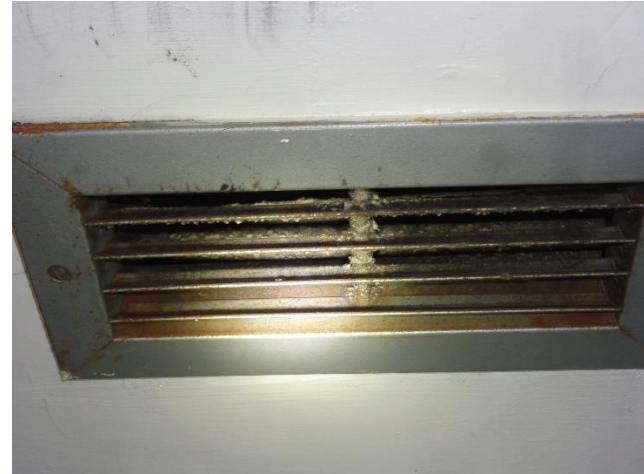
Photo 1a. Suspect Mold Growth in the Vents of Room 003.
