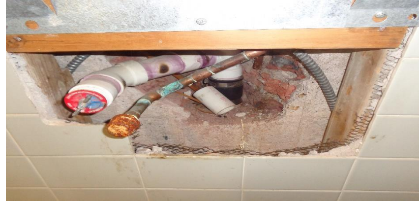
Photo 47a. Suspect Mold Growth on the Water Fountain Wall in Hallway H201.
