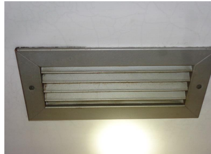
Photo 4a. Suspect Mold Growth in the Vents of Room 002.
