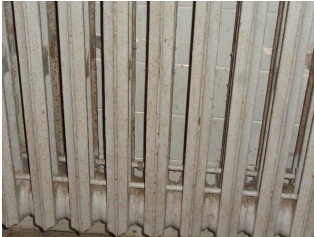
Photo 24. Suspect Mold Growth on the Radiator in Hallway H101.
