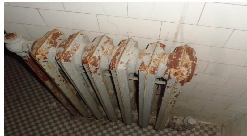
Photo 36a. Suspect Mold Growth on the Radiator in Room 104.
