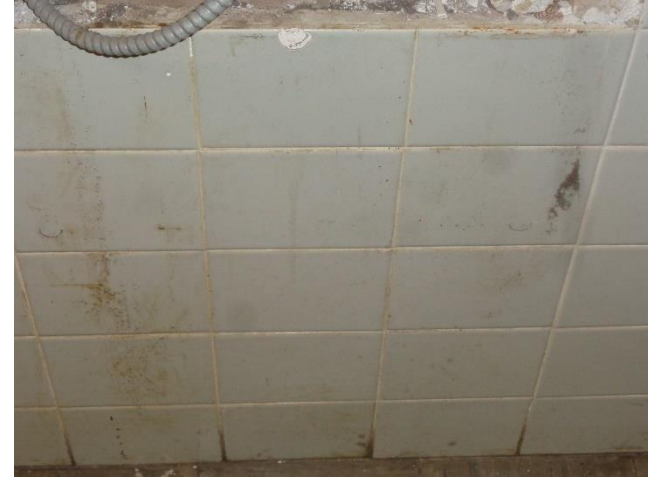
Photo 25a. Suspect Mold Growth where the Water Fountain used to be in Hallway H101.
