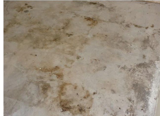
Photo 3a. Suspect Mold Growth on the Concrete Floor of Room 003a.
