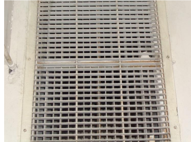
Photo 15a. Suspect Mold Growth Inside the Vents of Room 009.
