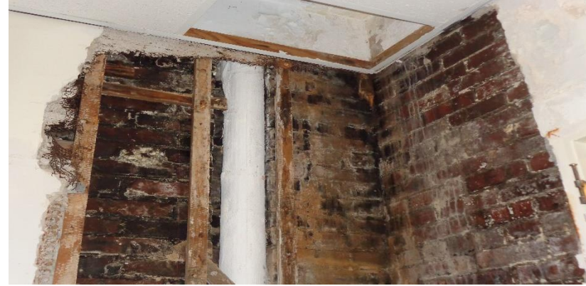
Photo 49a. Northwest Corner Suspect Mold Growth from Ceiling to Floor in Room 208.
