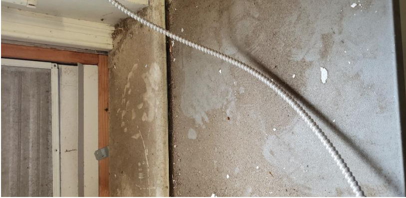
Photo 45. Suspect Mold Growth in the Northeast Corner of Room 205.
