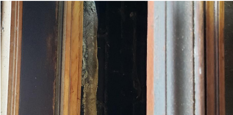
Photo 40. Window showing Suspect Mold Growth in Room 108a.
