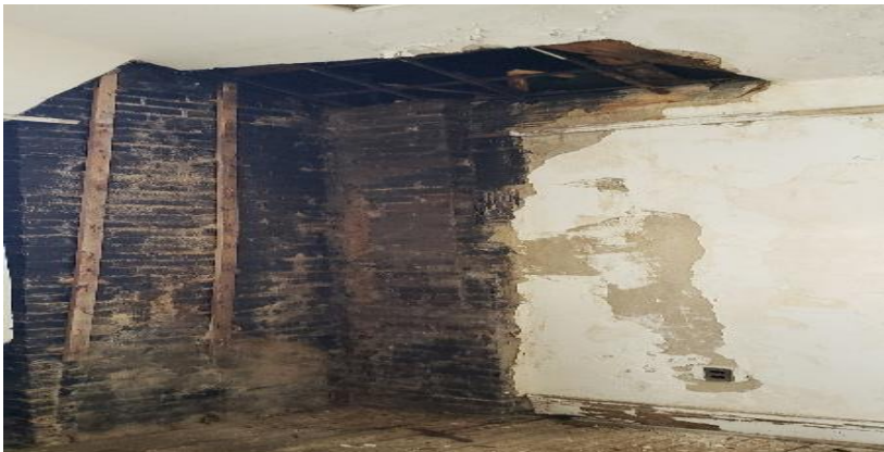
Photo 60. Suspect Mold Growth on the Southwest Corner in 218.
