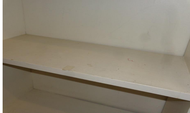
Photo 35a. Suspect Mold Growth on the Bookshelves in Room 102a no glove.
