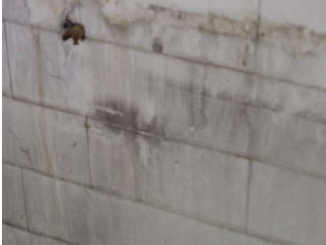
Photo 23. Suspect Mold Growth in Room 110.
