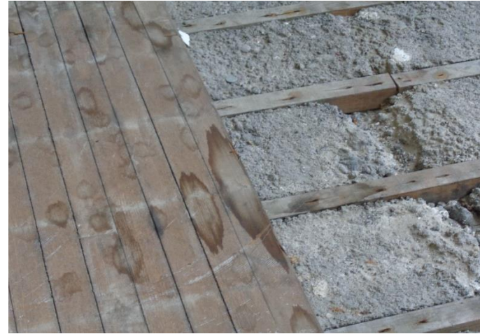
Photo 21. Suspect Mold Growth throughout the Floor of Room 109.
