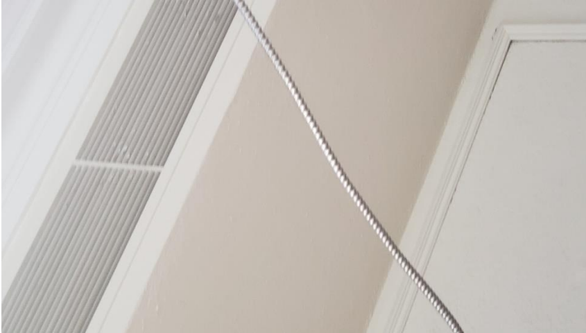
Photo 33. Suspect Mold Growth on the Vents of Room 106.
