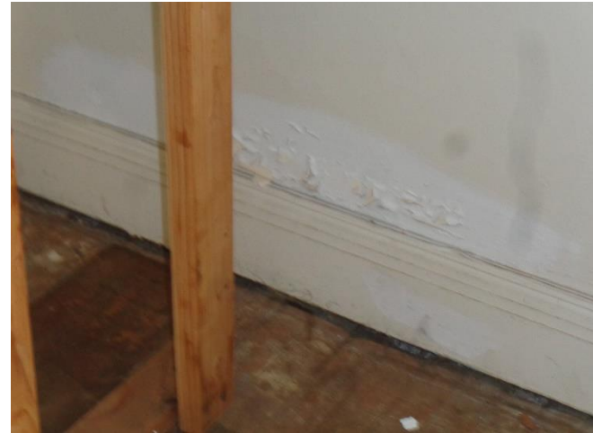
Photo 27a. Suspect Mold Growth below the Southern Window of Room 112.
