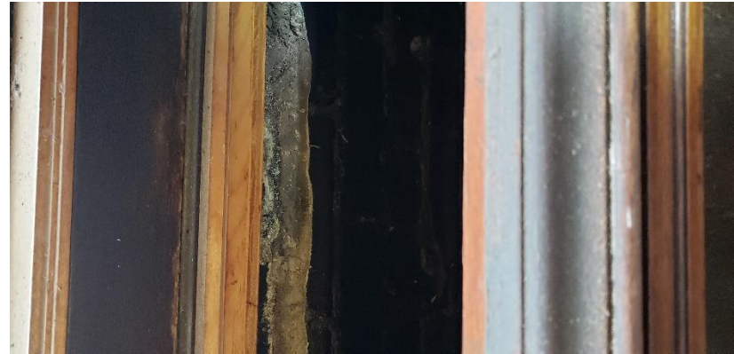
Photo 40. Window showing Suspect Mold Growth in Room 108a.
