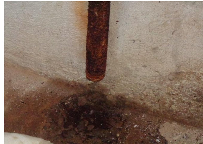
Photo 18. Suspect Mold Growth in the Pit Located at the Southwest Corner of Room 015 has more growth .
