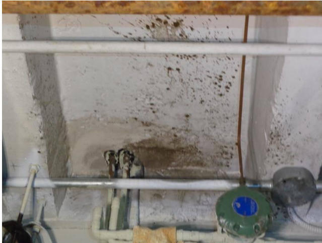
Photo 9. Suspect Mold Growth on the Ceiling of the Northern Wall in Room 017.
