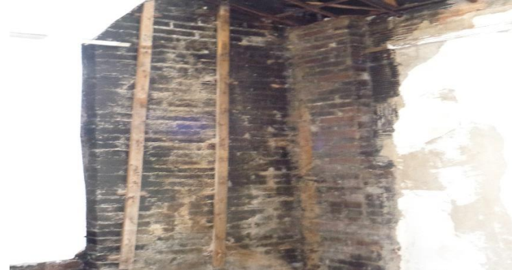
Photo 60a. Suspect Mold Growth on the Southwest Corner in 218.
