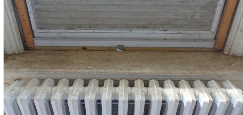
Photo 57a. Suspect Mold Growth on the Windows of Room 214.
