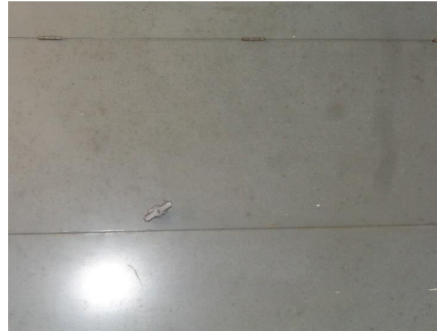
Photo 19a. Suspect Mold Growth on the Electrical Panel at the Southeast Corner of Room 016.
