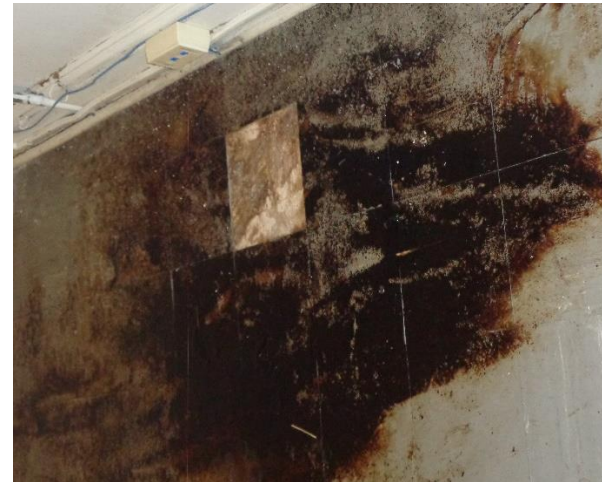
Photo 32a. Suspect Mold Growth on the Northeast Corner Floor in Room 107 has worsened.
