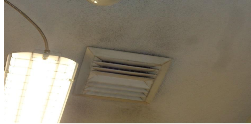
Photo 59. Suspect Mold Growth on the Vent by the Ramp near Rooms 213 and 214.
