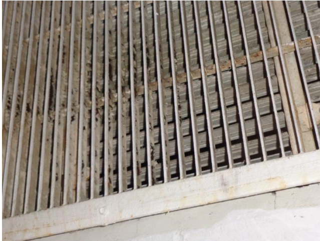
Photo 17. Suspect Mold Growth in the Vents of Room 011.
