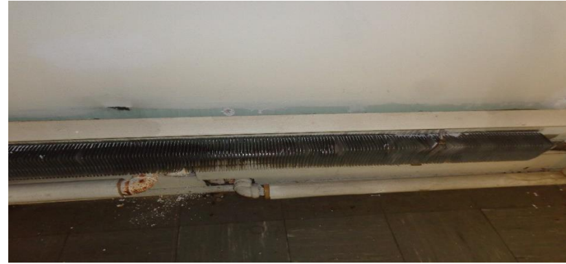
Photo 54a. Suspect Mold Growth on the Radiator in Room 213.
