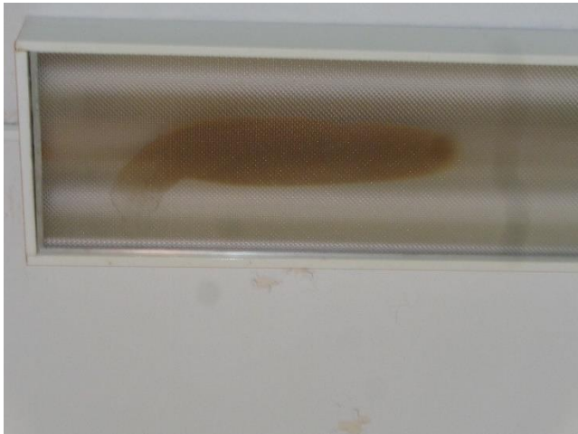
Photo 26. Suspect Mold Growth on the Northern Light Fixtures of Room 112.
