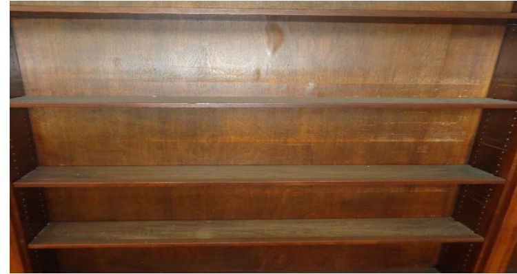
Photo 37a. Suspect Mold Growth on All Bookshelves in Room 108.
