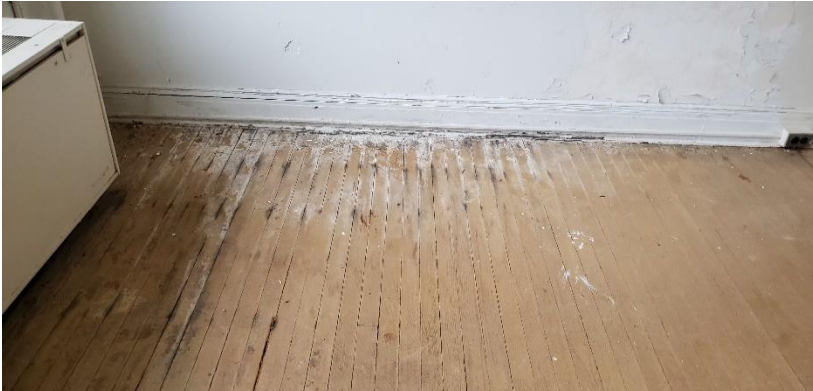
Photo 41. Suspect Mold Growth on the Floor at the Southeast Corner of Room 201.
