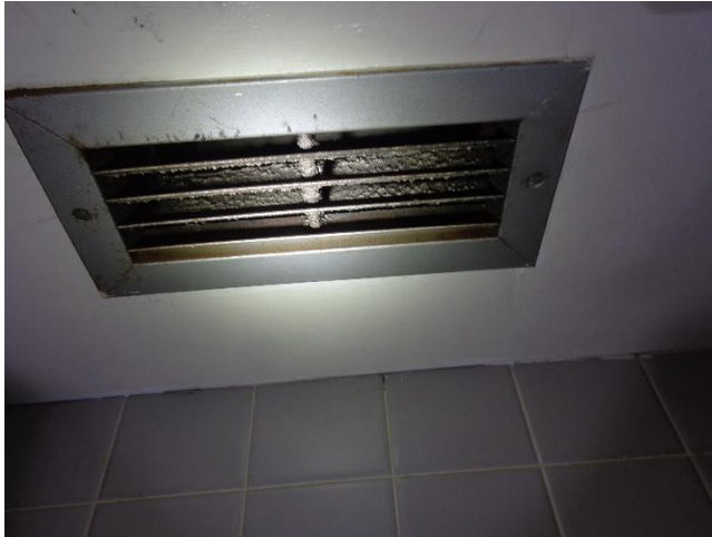
Photo 1. Suspect Mold Growth in the Vents of Room 003.
