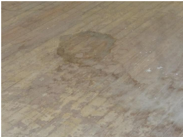
Photo 30. Suspect Mold Growth throughout the Floor of Room 113.
