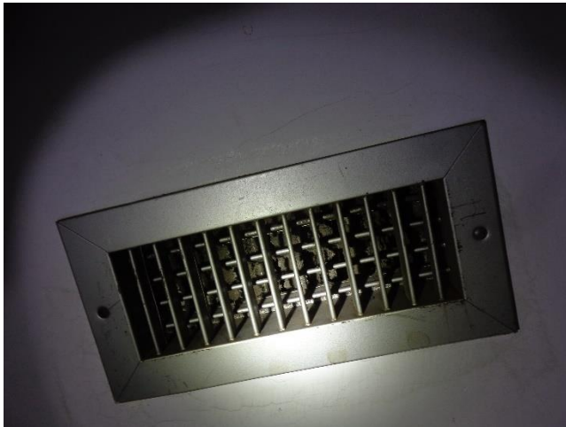
Photo 4. Suspect Mold Growth in the Vents of Room 002.
