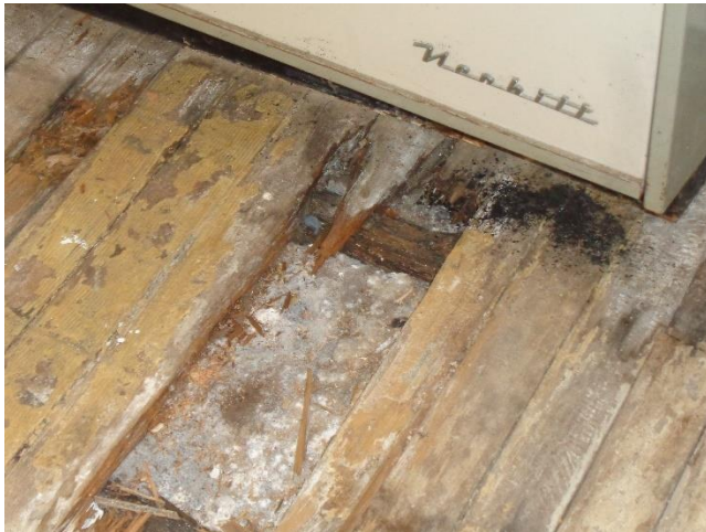
Photo 28. Suspect Mold Growth on the Floor of Room 112.
