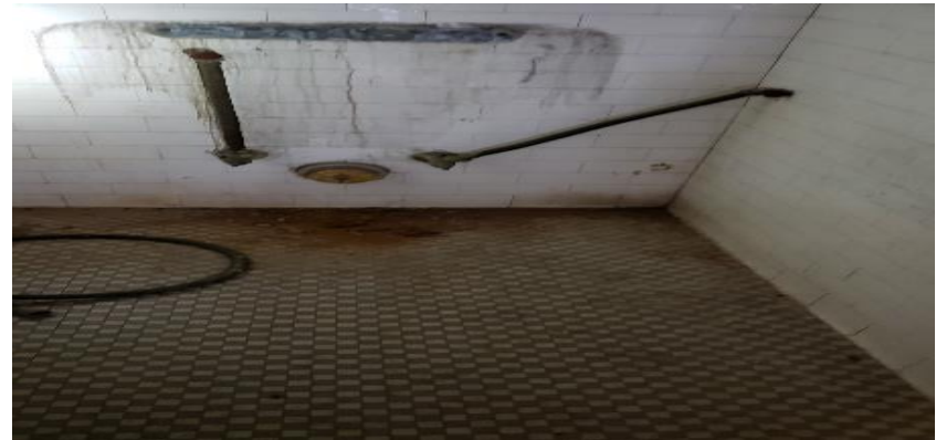
Photo 52. Suspect Mold Growth in Room 211.
