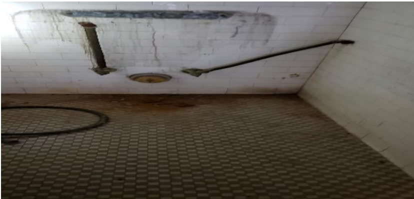
Photo 52. Suspect Mold Growth in Room 211.
