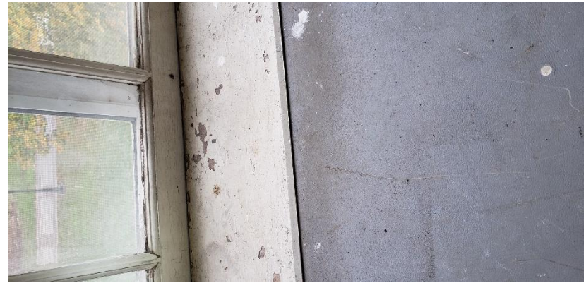
Photo 44. Suspect Mold Growth on the Eastern Window of Room 203.
