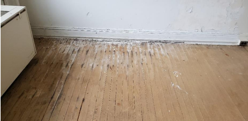
Photo 41. Suspect Mold Growth on the Floor at the Southeast Corner of Room 201.
