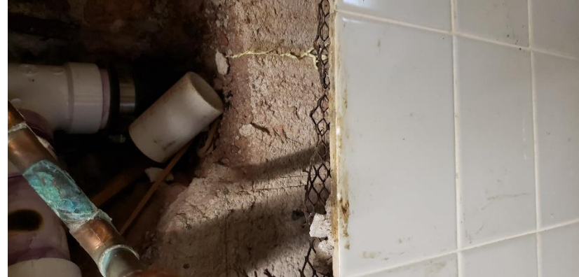
Photo 47. Suspect Mold Growth on the Water Fountain Wall in Hallway H201.
