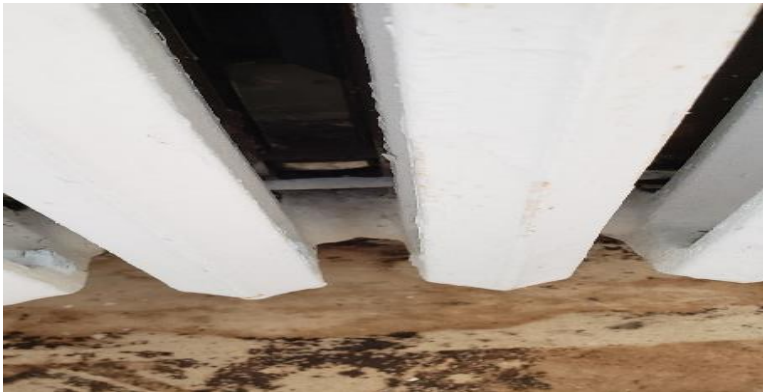
Photo 56. Suspect Mold Growth on the Radiator of Room 214.
