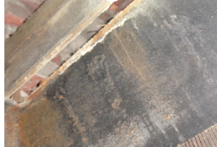
Photo 31a. Suspect Mold Growth inside the Fire Place in Room 105.
