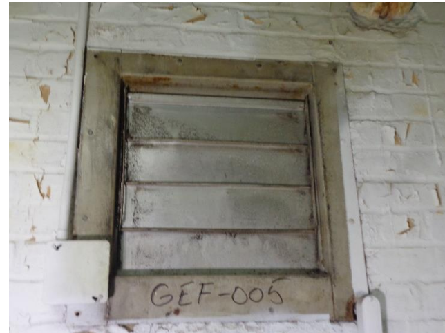
Photo 20. Suspect Mold Growth on the Vent at the Southeast Corner of Room 016.
