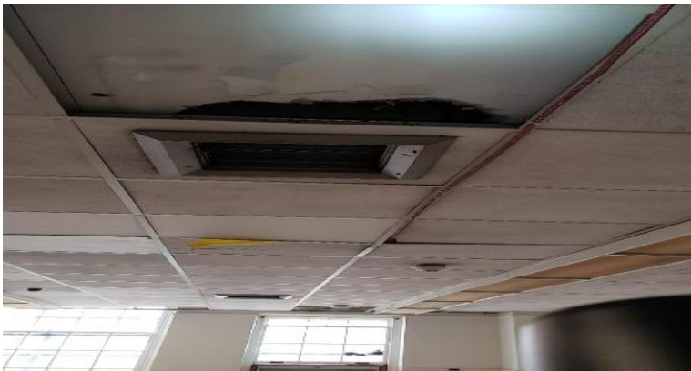
Photo 58. Suspect Mold Growth on the Vents in Room 214.
