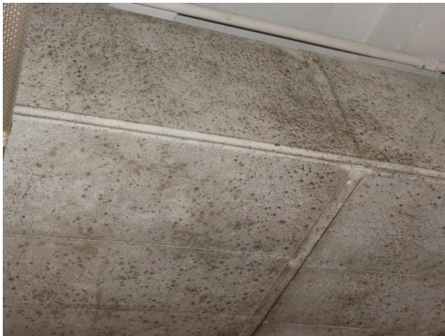
Photo 14. Suspect Mold Growth Surrounding the Vents of Room 009.
