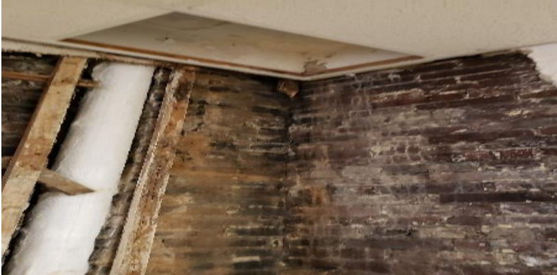
Photo 49. Northwest Corner Suspect Mold Growth from Ceiling to Floor in Room 208.
