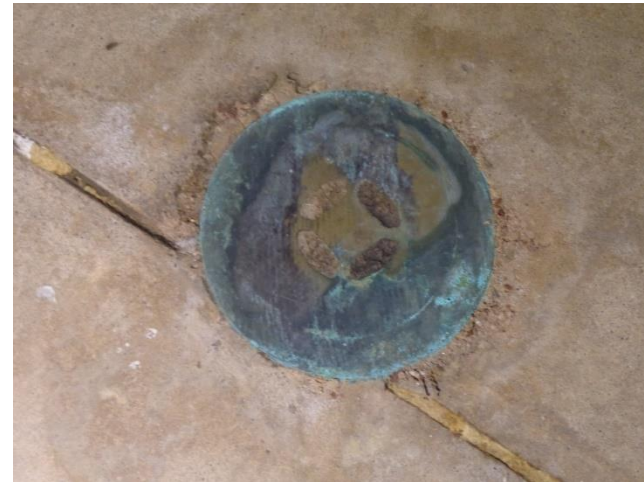
Photo 12. Suspect Mold Growth on the Sealed Pipe Drain Located on the Southwest Floor of Room 017.
