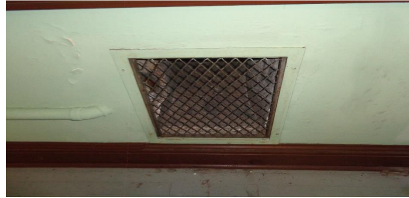
Photo 46a. Suspect Mold Growth on the Vents in Room 205.
