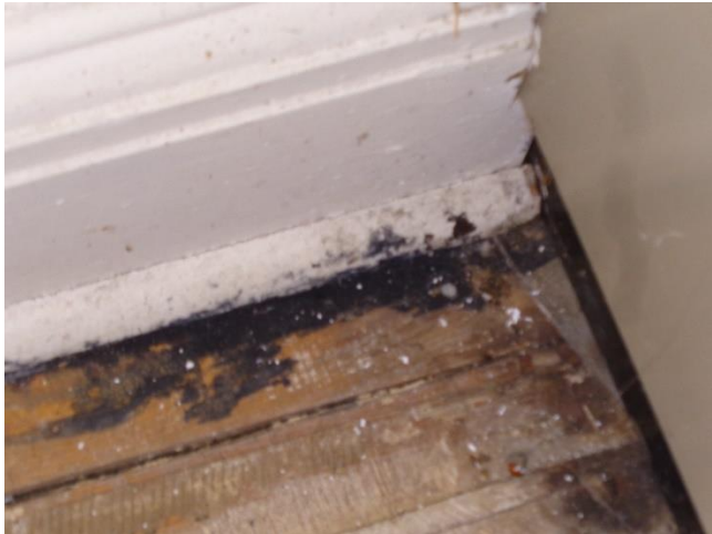
Photo 22. Suspect Mold Growth in the Southwest side of Room 109.
