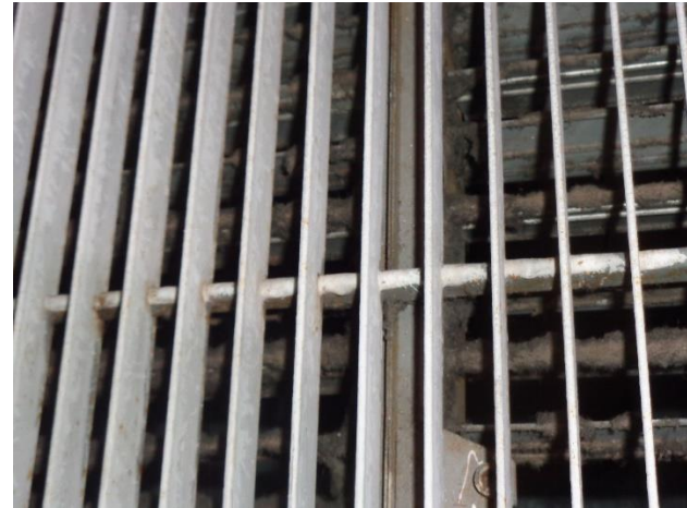
Photo 11a. Suspect Mold Growth in the Vent Located at the Southeastern Corner of Room 017.
