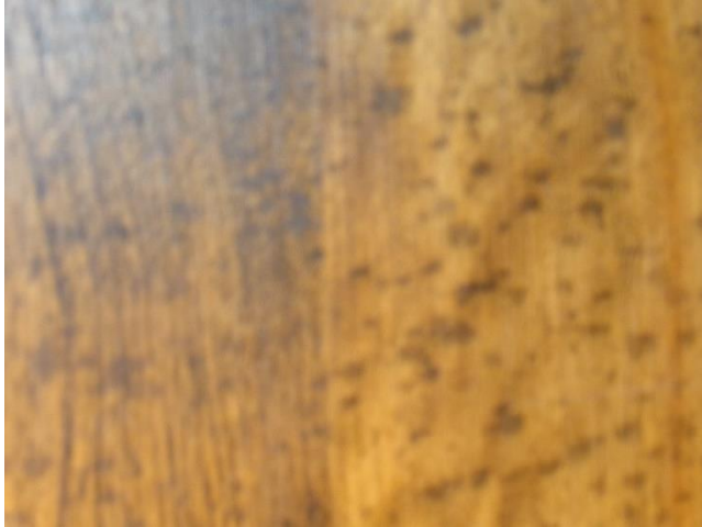
Photo 29. Suspect Mold Growth on the Door of Room 112.
