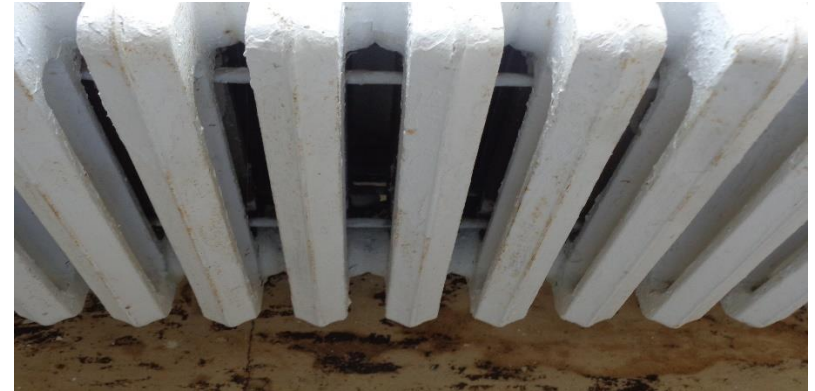
Photo 56a. Suspect Mold Growth on the Radiator of Room 214.
