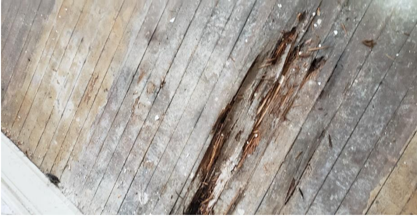
Photo 51. Suspect Mold Growth on the floor beneath the Western Window in Room 210.
