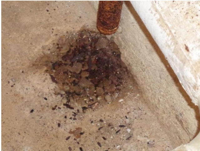
Photo 18. Suspect Mold Growth in the Pit Located at the Southwest Corner of Room 015.
