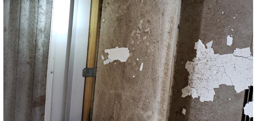
Photo 43. Suspect Mold Growth in the Southeast Corner of Room 202.
