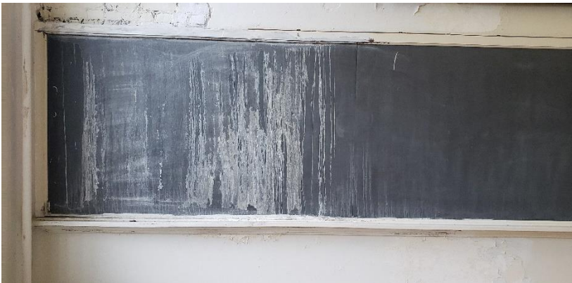
Photo 42. Suspect Mold Growth on the South Wall in Room 201.
