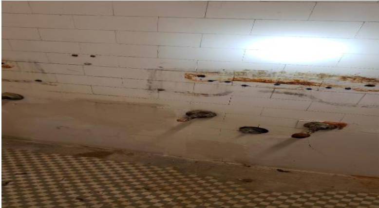
Photo 53. Suspect Mold Growth in Room 212.
