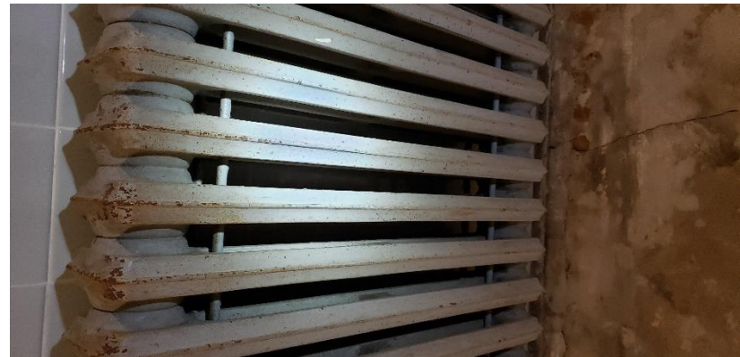
Photo 48. Suspect Mold Growth on the Radiator in Hallway H201. Ceiling in Room 206.
