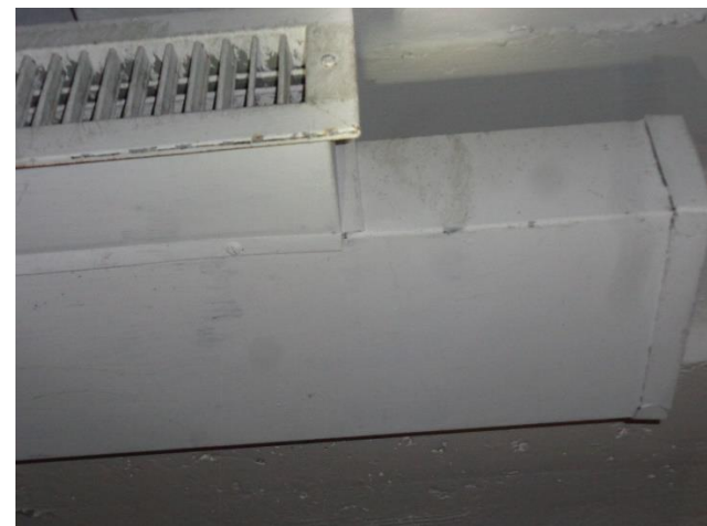
Photo 10a. Suspect Mold Growth in the Vents across the Ceiling in Room 017.
