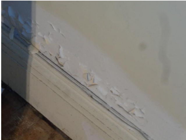
Photo 27. Suspect Mold Growth below the Southern Window of Room 112.
