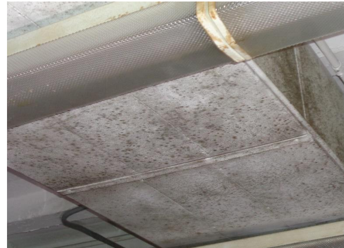
Photo 14a. Suspect Mold Growth Surrounding the Vents of Room 009 has worsened.
