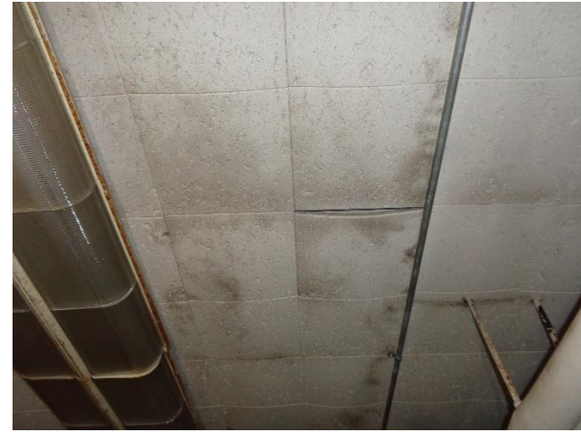
Photo 16. Ceiling Tiles throughout Room 011 Showing Suspect Mold Growth.
