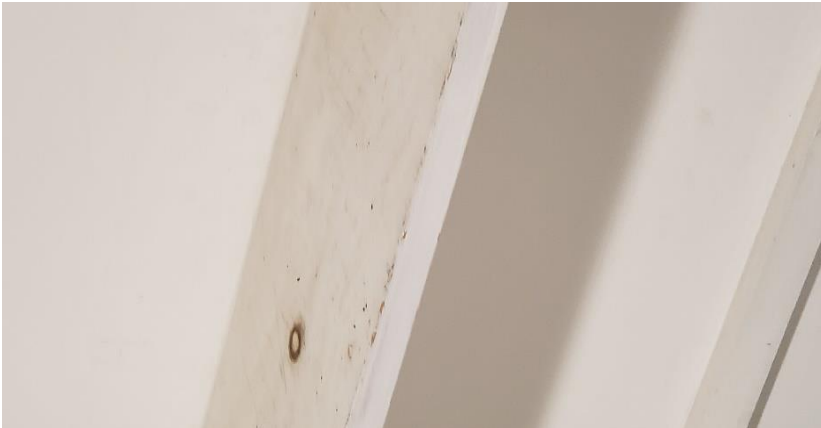
Photo 34. Suspect Mold Growth on the Bookshelves in Room 102.
