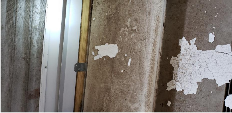
Photo 43. Suspect Mold Growth in the Southeast Corner of Room 202.
