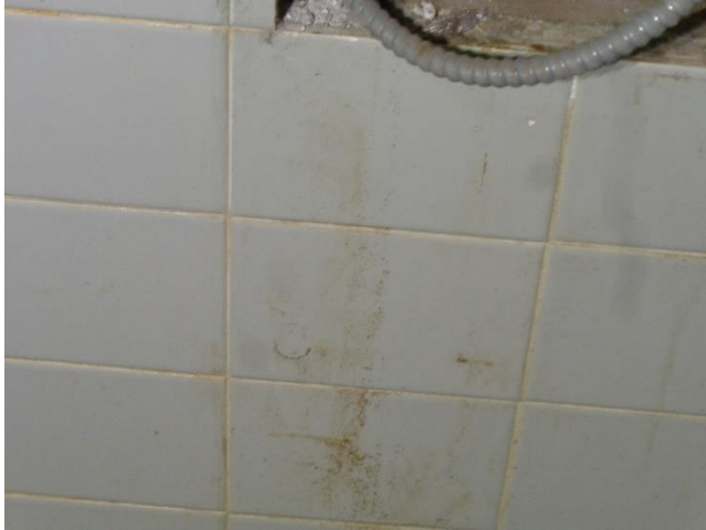
Photo 25. Suspect Mold Growth where the Water Fountain used to be in Hallway H101.
