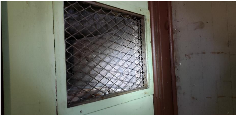
Photo 46. Suspect Mold Growth on the Vents in Room 205.
