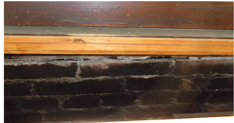
Photo 40a. Window showing Suspect Mold Growth in Room 108a.
