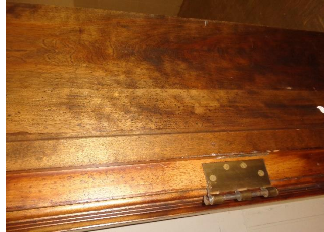
Photo 29a. Suspect Mold Growth on the Door of Room 112 has spread and worsened.
