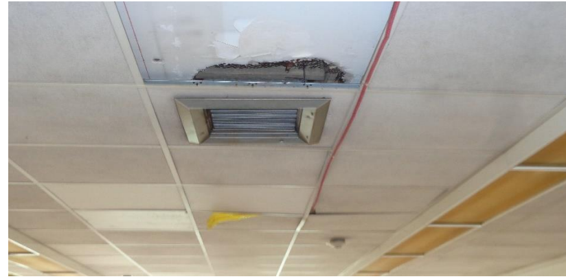
Photo 58. Suspect Mold Growth on the Vents in Room 214.
