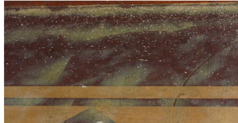
Photo 38a. Suspect Mold Growth on the Ground along the Eastern Wall in Room 108.
