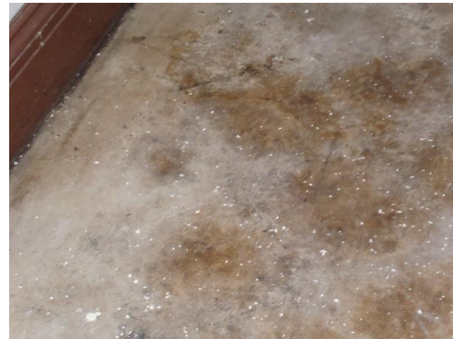
Photo 8. Suspect Mold Growth on the Floor of Room 008.
