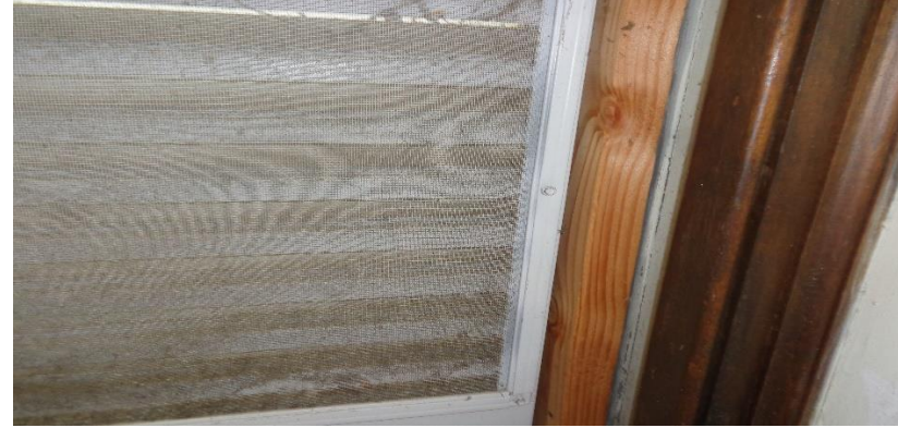
Photo 43a. Suspect Mold Growth in the Southeast Corner of Room 202.
