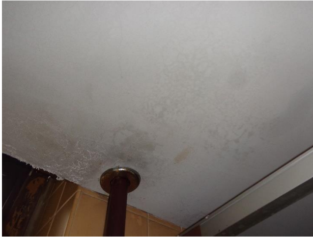
Photo 5. Suspect Mold Growth on the Eastern Ceiling in Room 002.
