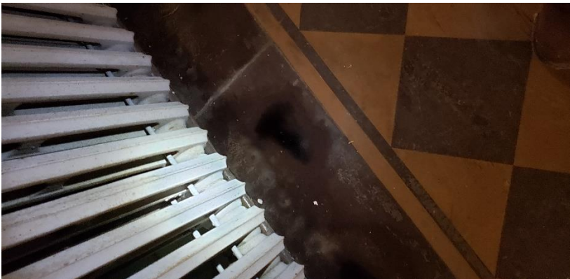
Photo 50. Suspect Mold Growth on Radiator in Hallway H203.
