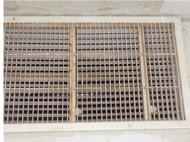
Photo 17a. Suspect Mold Growth in the Vents of Room 011.
