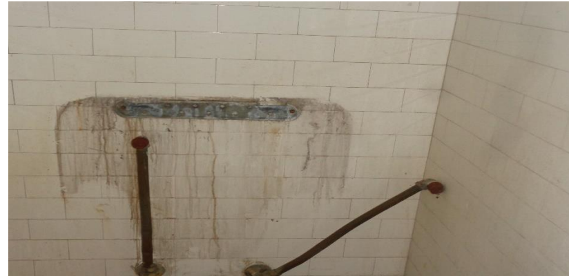
Photo 52a. Suspect Mold Growth in Room 211.
