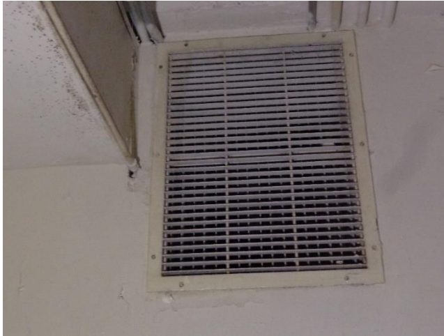
Photo 15. Suspect Mold Growth Inside the Vents of Room 009.
