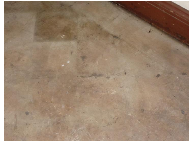
Photo 8a. Suspect Mold Growth on the Floor of Room 008.
