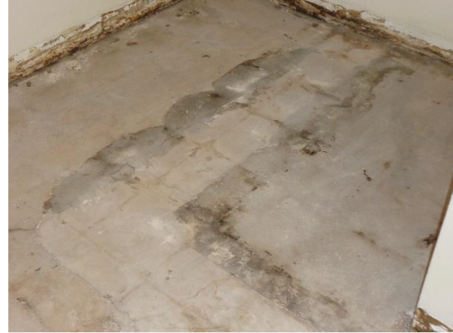
Photo 6a. Suspect Mold Growth on the Concrete Floor of Room 002a.
