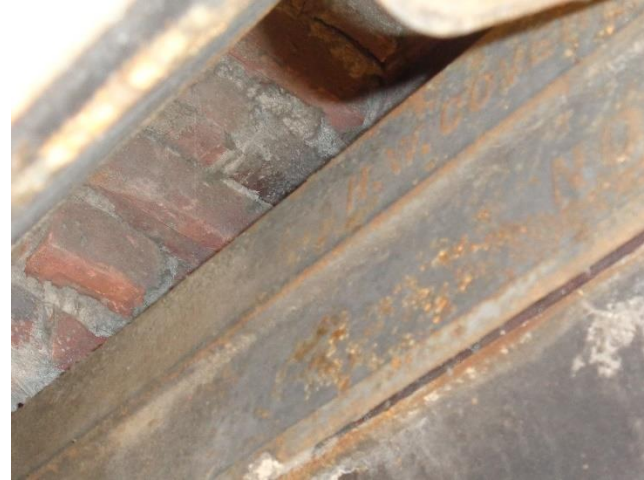
Photo 31. Suspect Mold Growth inside the Fire Place in Room 105.
