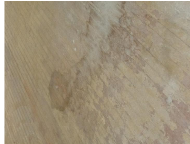
Photo 30a. Suspect Mold Growth throughout the Floor of Room 113 has worsened.
