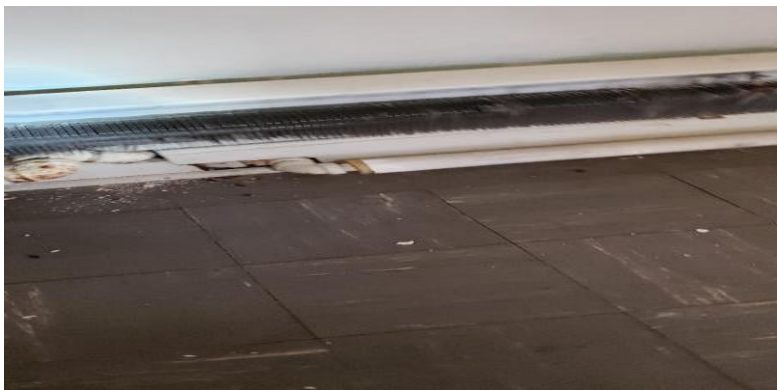
Photo 54. Suspect Mold Growth on the Radiator in Room 213.
