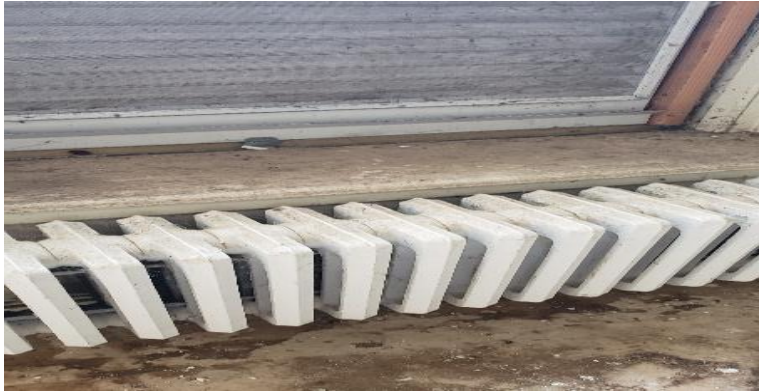
Photo 57. Suspect Mold Growth on the Windows of Room 214.
