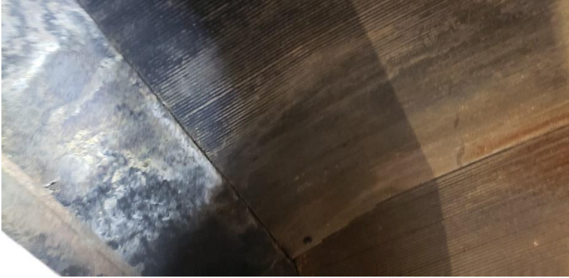
Photo 39. Suspect Mold Growth inside the Fire Place in Room 108.
