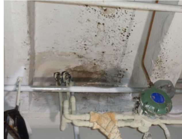
Photo 9. Suspect Mold Growth on the Ceiling of the Northern Wall in Room 017.
