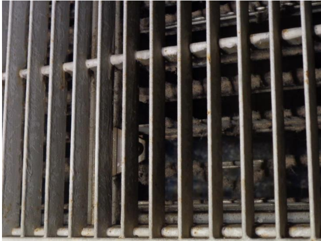
Photo 11. Suspect Mold Growth in the Vent Located at the Southeastern Corner of Room 017.
