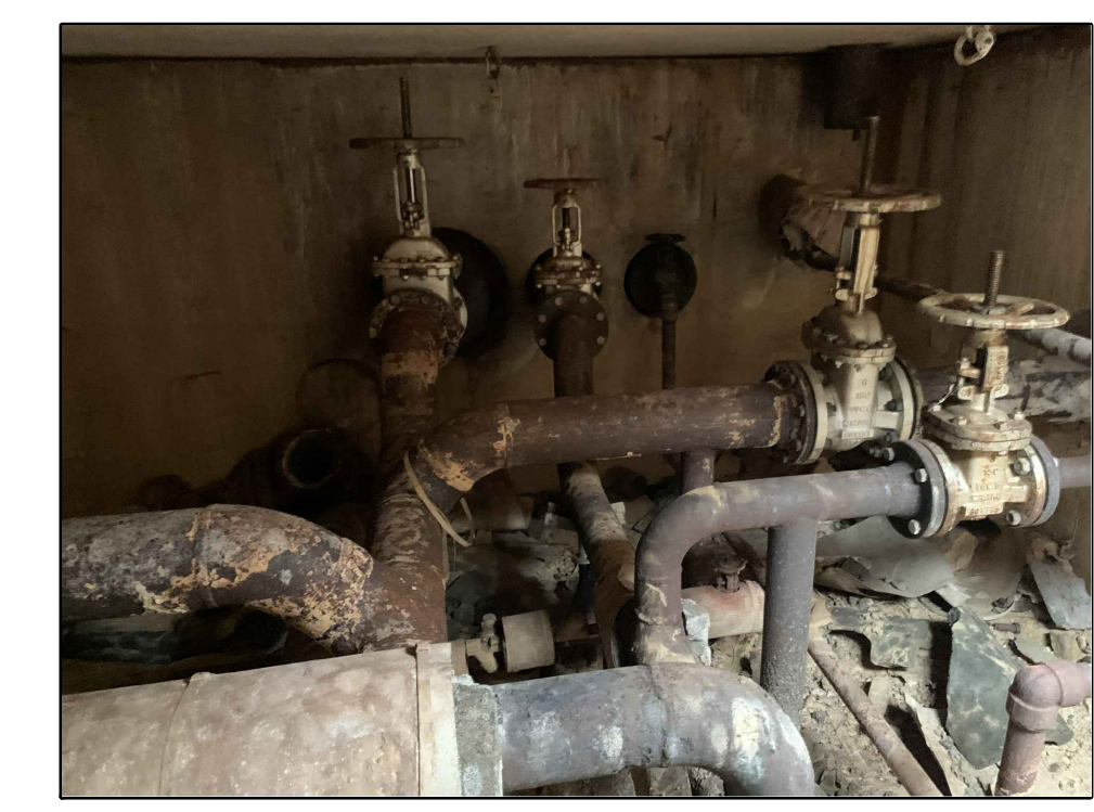
PHOTO D Piping To Armstrong Hall To Be Replaced.
