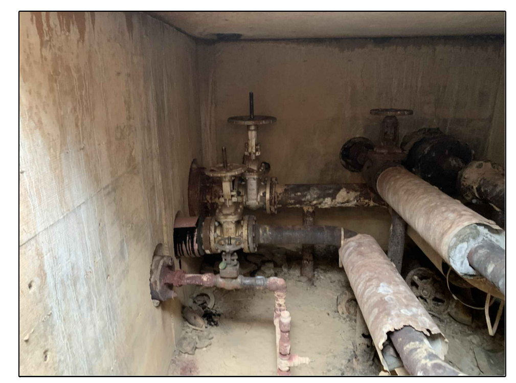
PHOTO B Existing Piping And Valves To Remain
