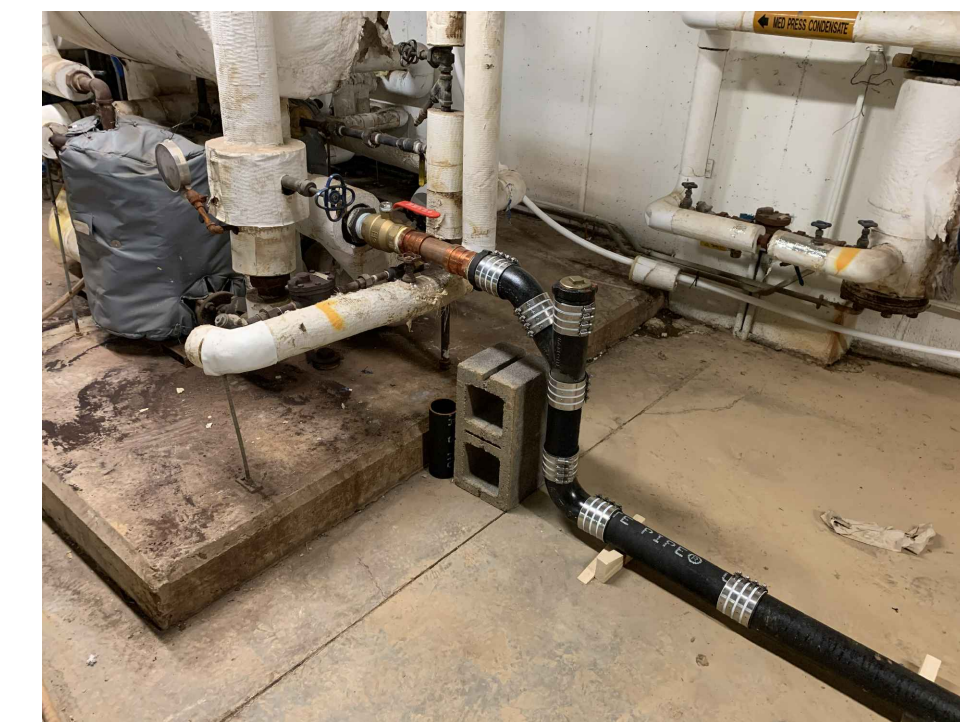
PHOTO F Temporary Piping And Fittings To Be Disconnected And Turned Over To TCNJ. Cap To Be Placed On Valve Discharge And Insulated.
