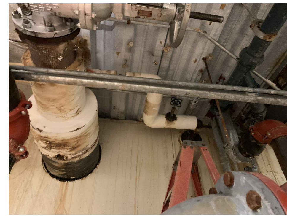
PHOTO A High Pressure Condensate Valve To Be Replaced
