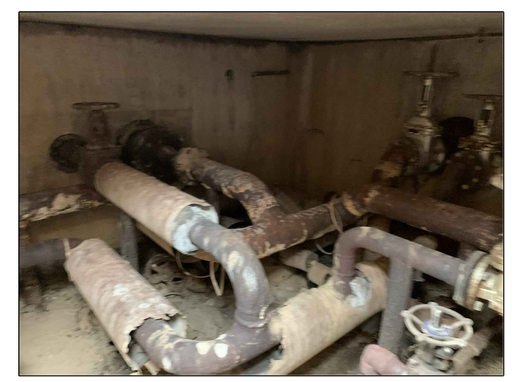
PHOTO A Existing Piping To Be Reinsulated.
