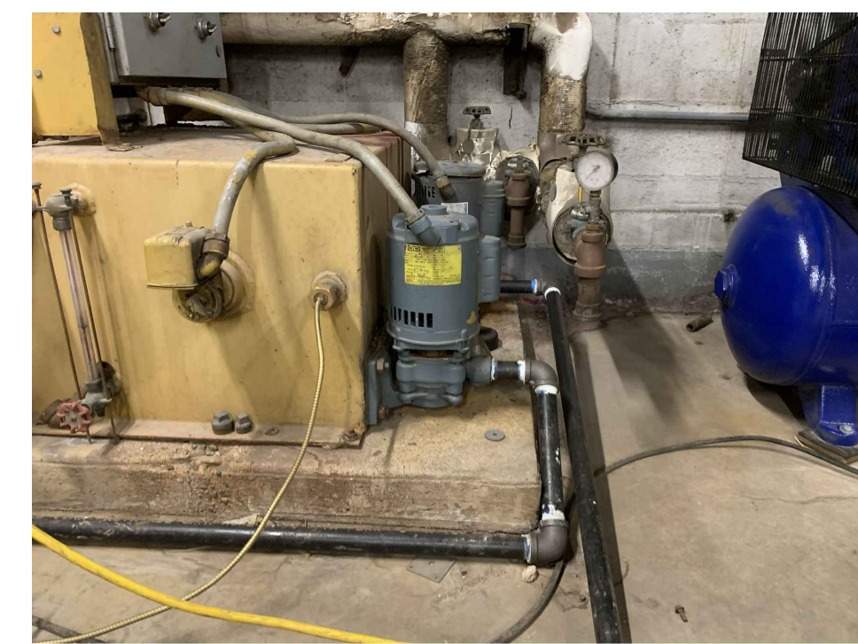
PHOTO C Temporary Piping From Condensate Receiver Pump Discharge To Be Removed. Permanent Piping To Be Reconnected.
