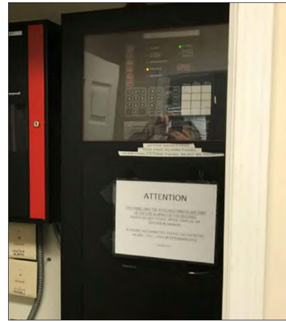
PHOTO B - SIEMENS FIRE ALARM CONTROL PANEL Siemens MXL Addressable Fire Alarm Control Panel With Exposed Conduit Located In Building Office
