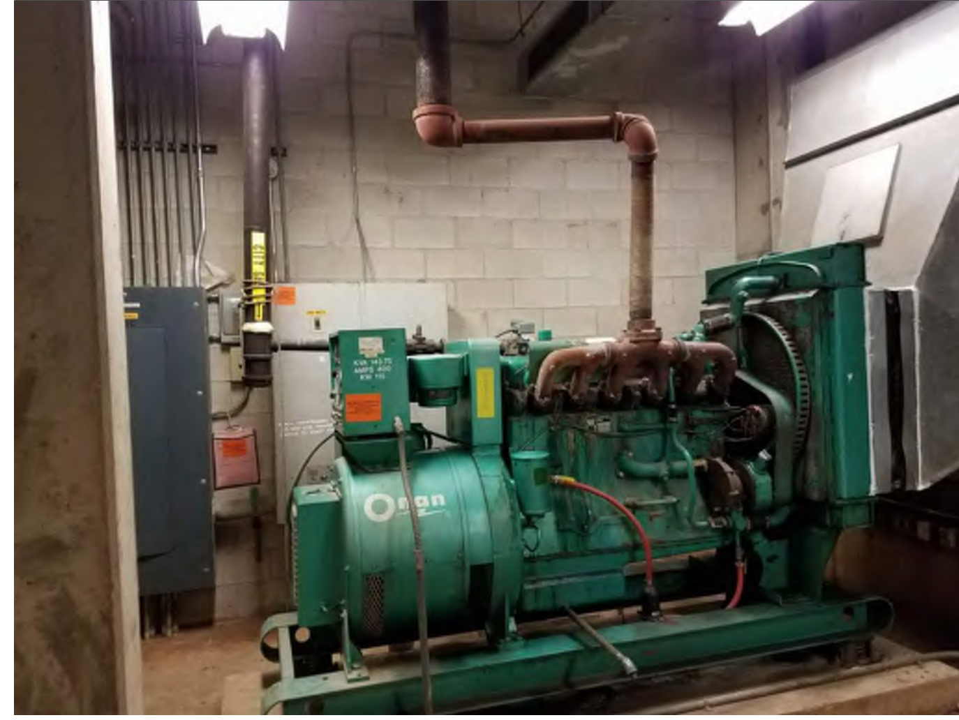
Existing Gas Generator
