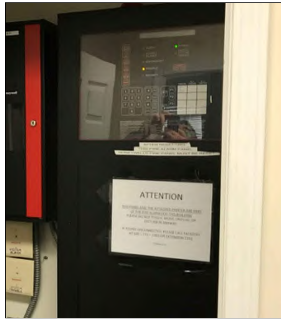
PHOTO A - SIEMENS FIRE ALARM CONTROL PANEL Siemens MXL Addressable Fire Alarm Control Panel Located Within Electrical Room
