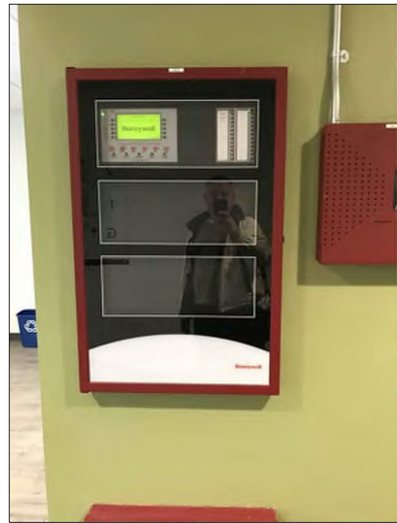
PHOTO A - HONEYWELL FIRE ALARM CONTROL PANEL Honeywell XLS 3000 Addressable Fire Alarm Control Panel Located Within Lower Level Corridor
