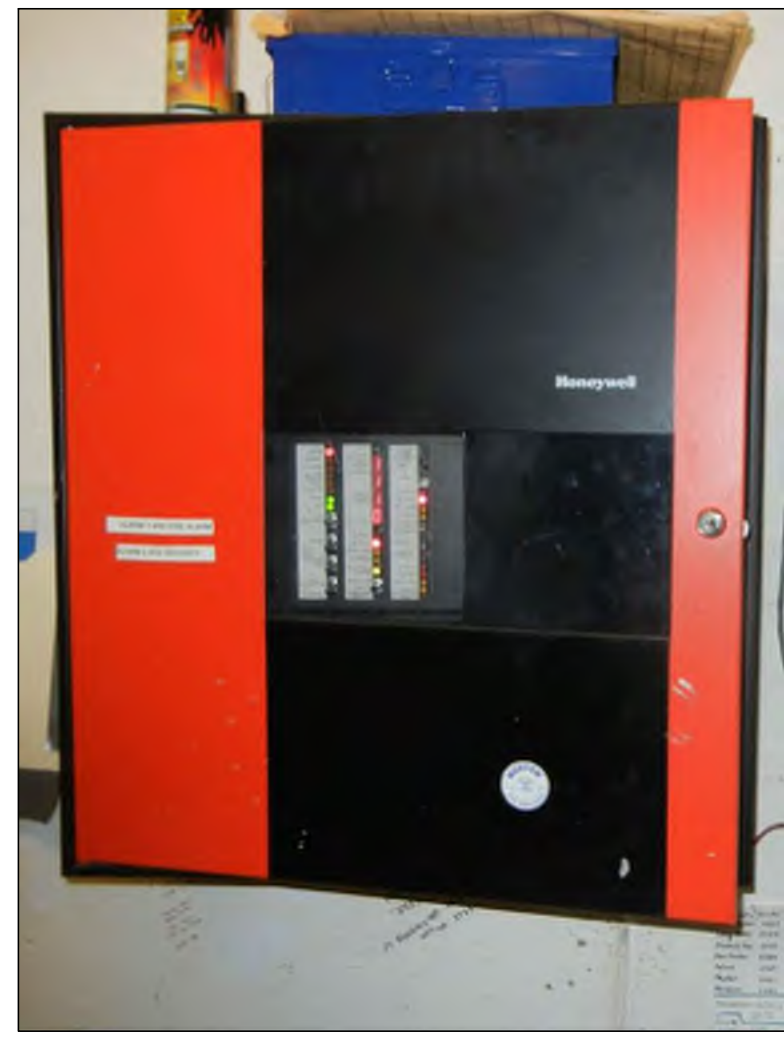
PHOTO A - INTERMEDIARY FIRE ALARM CONTROL PANEL Honeywell FS90 Intermediary Fire Alarm Control Panel Located Within Electrical Room
