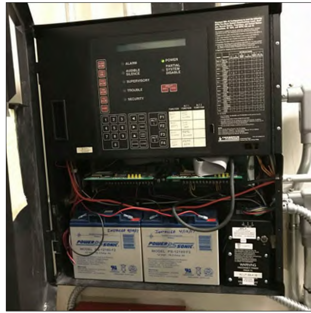
PHOTO A - SIEMENS FIRE ALARM CONTROL PANEL Existing Siemens MXL Addressable Fire Alarm Control Panel With Exposed Conduit Located Within Lower Level Electrical Room
