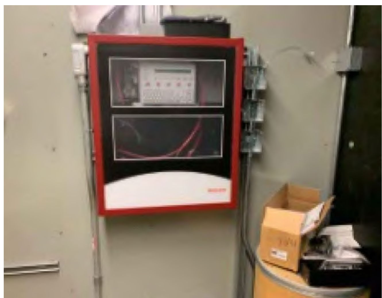
PHOTO A - HONEYWELL FIRE ALARM CONTROL PANEL Fire Alarm Control Panel Located Within Switchgear Building
