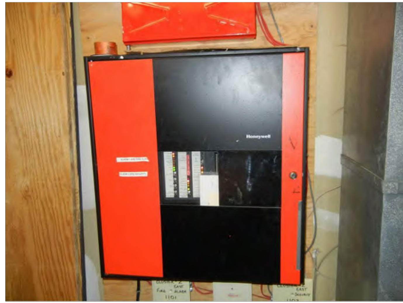
PHOTO A - INTERMEDIARY FIRE ALARM CONTROL PANEL Honeywell Intermediary Fire Alarm Control Panel With Exposed Conduit Located In Office Building Mechanical Room
