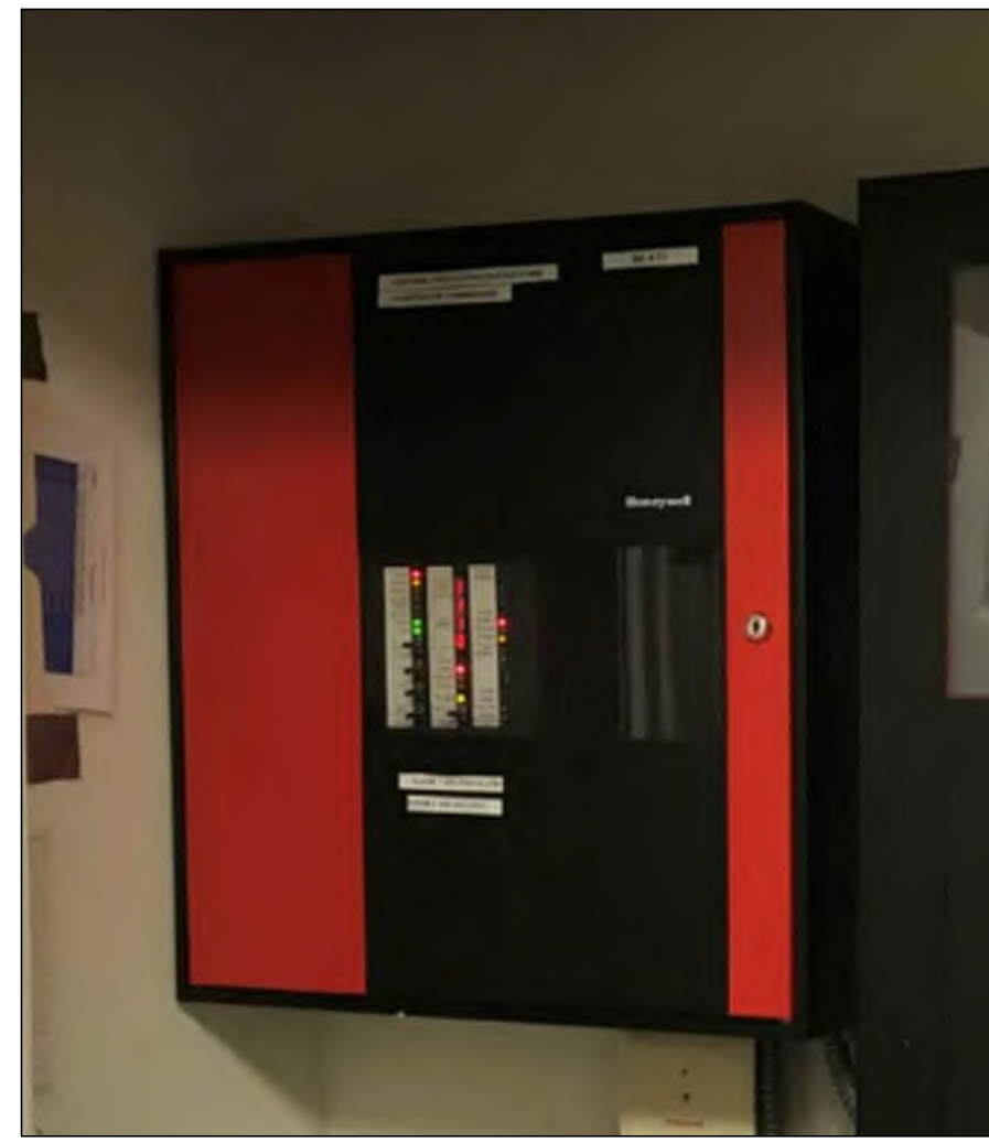
PHOTO B - INTERMEDIARY FIRE ALARM CONTROL PANEL Honeywell FS90 Intermediary Fire Alarm Control Panel Located Within Electrical Room
