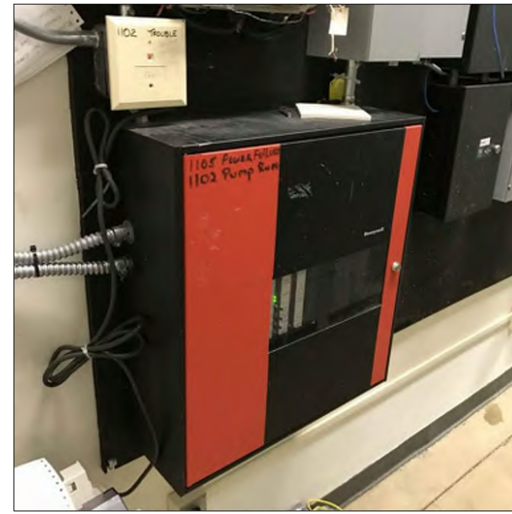
PHOTO B - INTERMEDIARY FIRE ALARM CONTROL PANEL Existing Honeywell FS90 Intermediary Fire Alarm Control Panel With Exposed Conduit Located Within Lower Level Electrical Room
