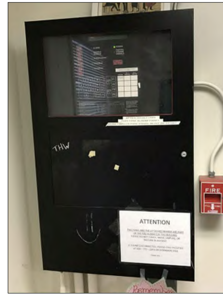
PHOTO B - SIEMENS FIRE ALARM CONTROL PANEL Siemens MXL Addressable Fire Alarm Control Panel Located Within Office Lobby
