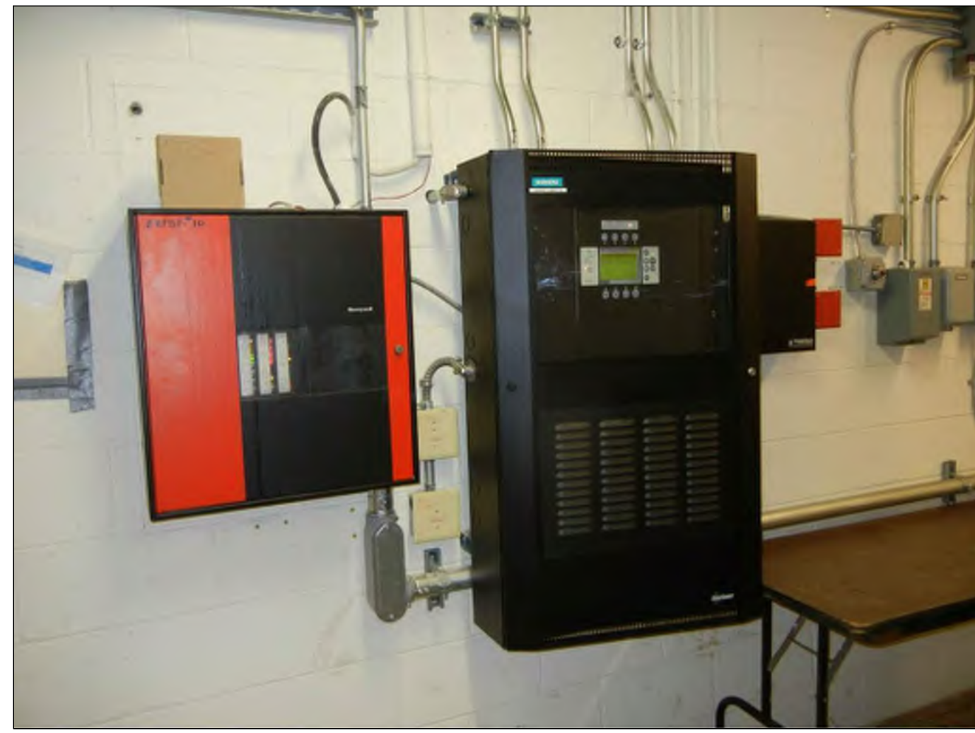
PHOTO A - SIEMENS FIRE ALARM CONTROL PANEL
