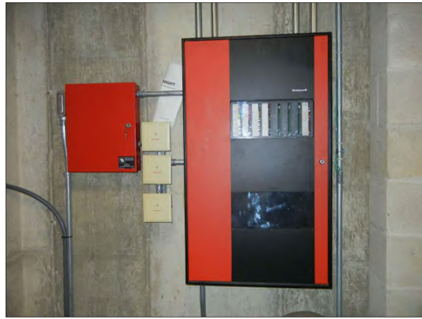
PHOTO A - HONEYWELL FIRE ALARM CONTROL PANEL Existing Honeywell FS90 Addressable Fire Alarm Control Panel With Exposed Conduit Located In Lower Level Electrical Room
