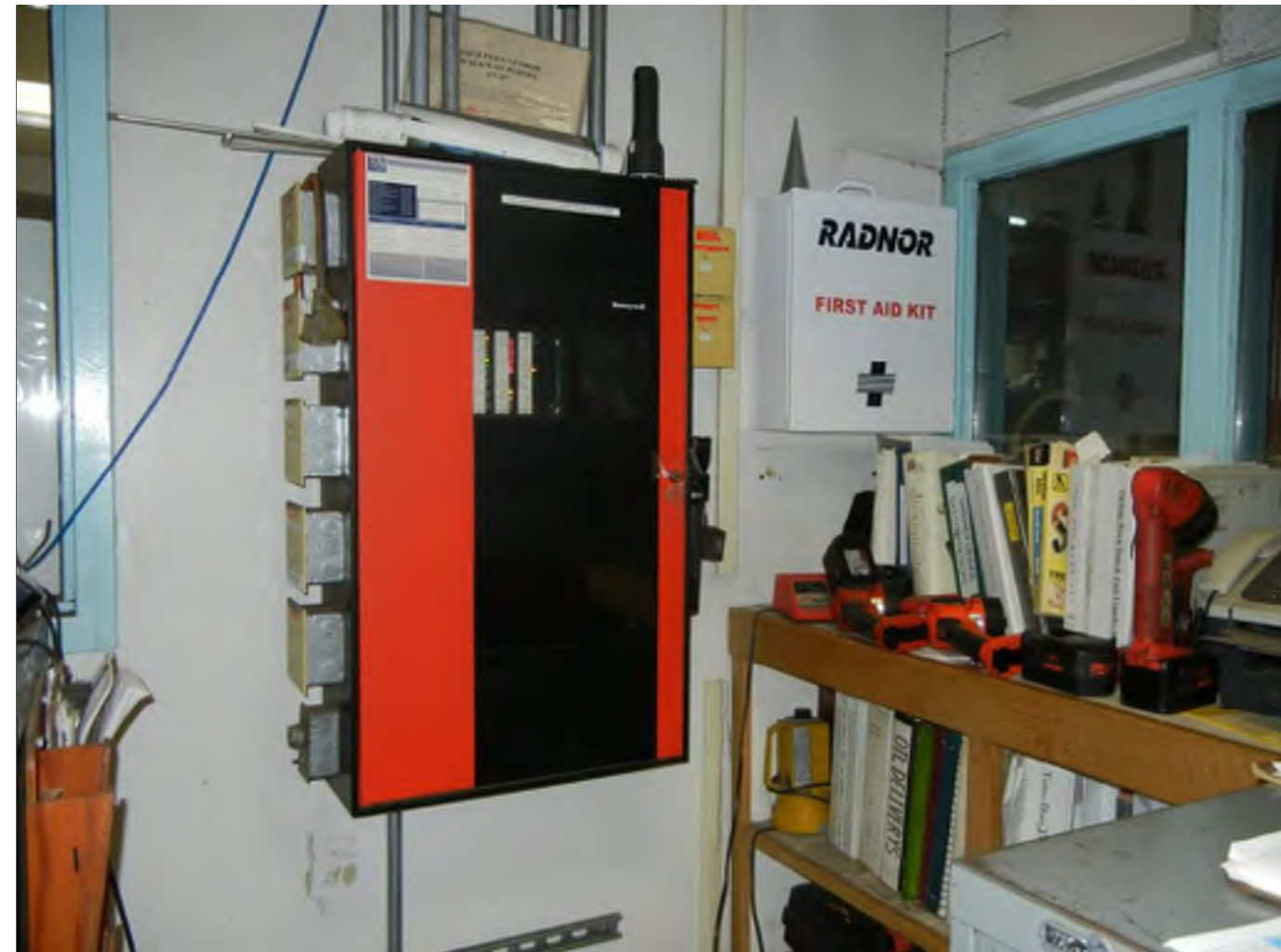
PHOTO A - HONEYWELL FIRE ALARM CONTROL PANEL Honeywell FS90 Addressable Fire Alarm Control Panel With Exposed Conduit Located Within Lower Level Electrical Room
