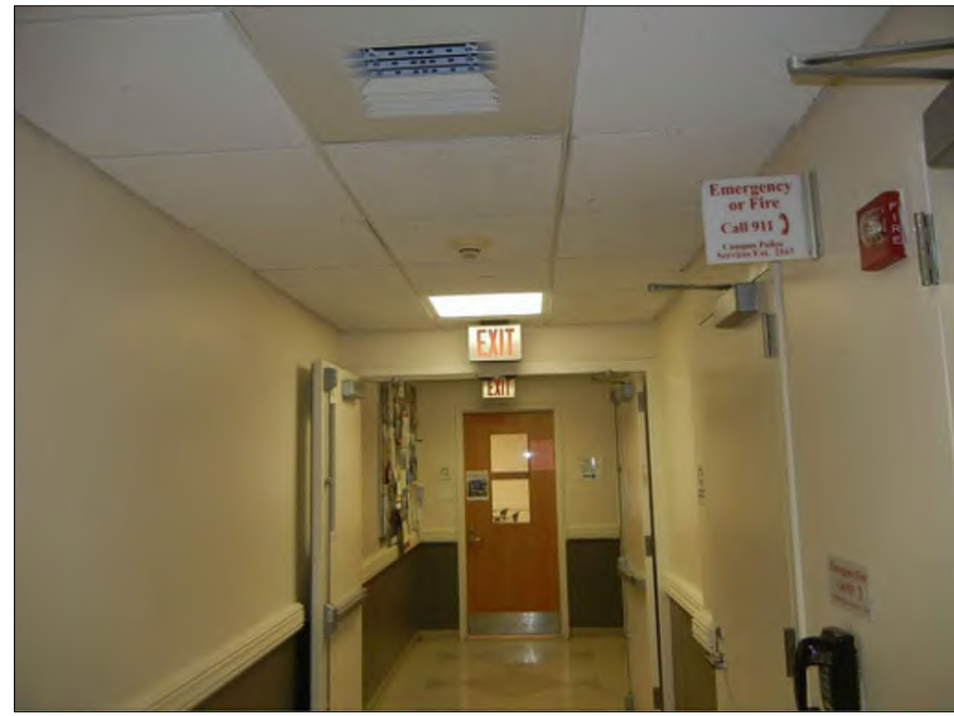
SIEMENS FIRE ALARM DEVICES
