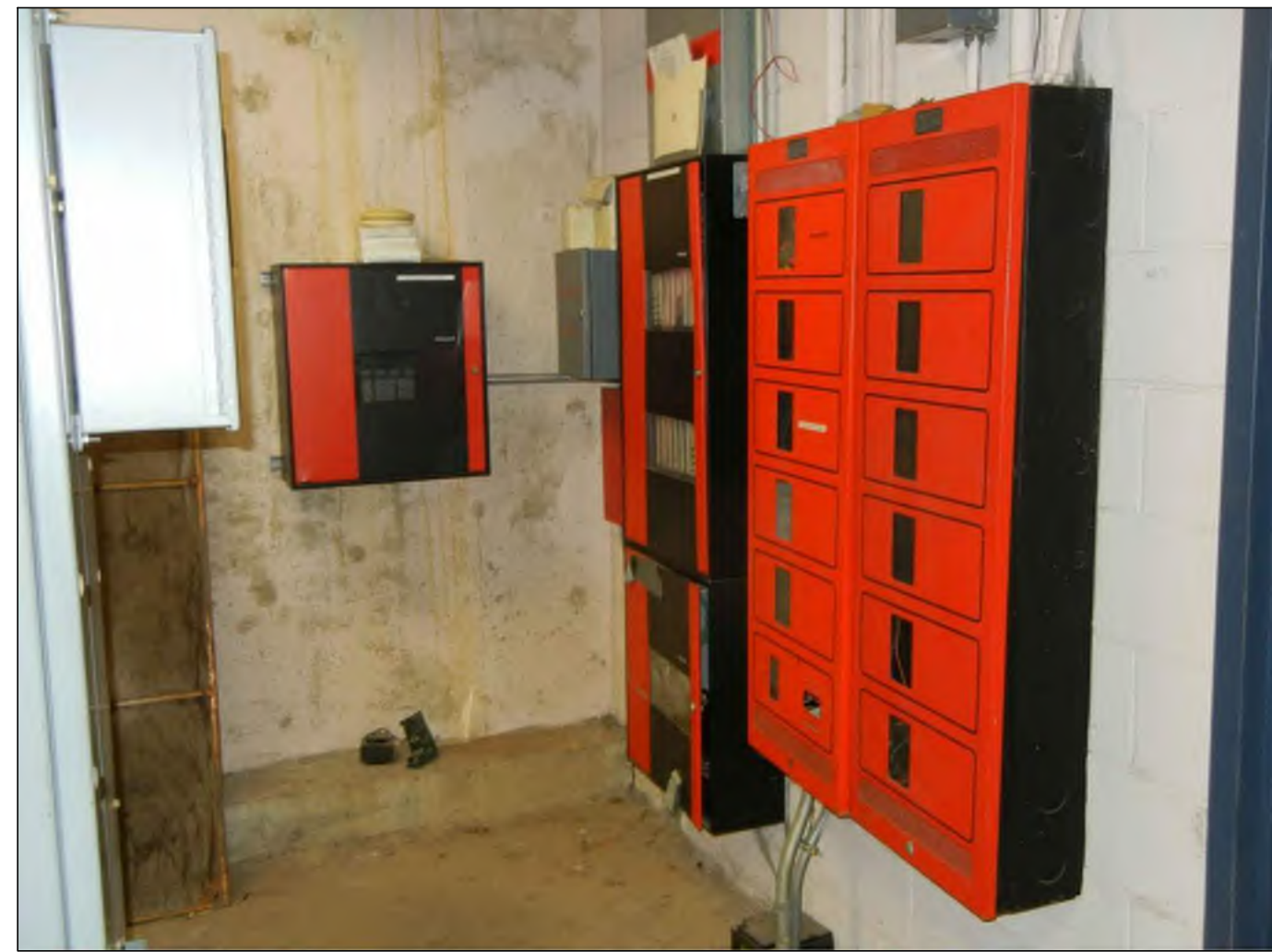
PHOTO A - HONEYWELL FIRE ALARM CONTROL PANEL Honeywell FS90 Addressable Fire Alarm Control Panel And Honeywell Remote Fire Alarm Annunciator With Exposed Conduit Located Within Lower Level Electrical Room
