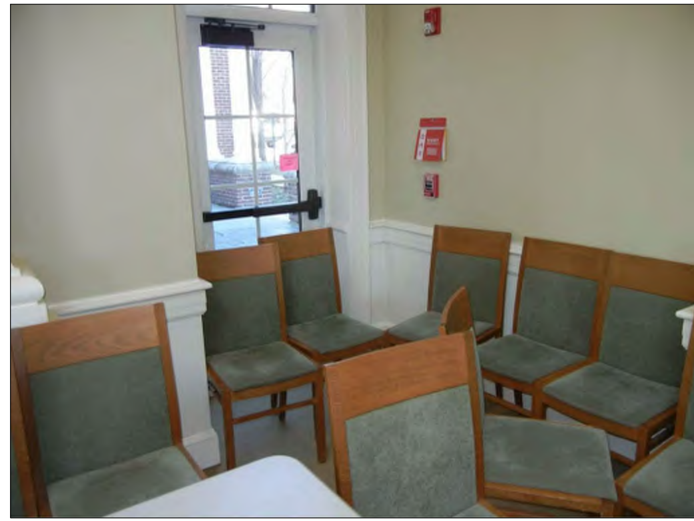
HONEYWELL FIRE ALARM DEVICES Existing Honeywell Addressable Fire Alarm Devices Located Throughout The Building
