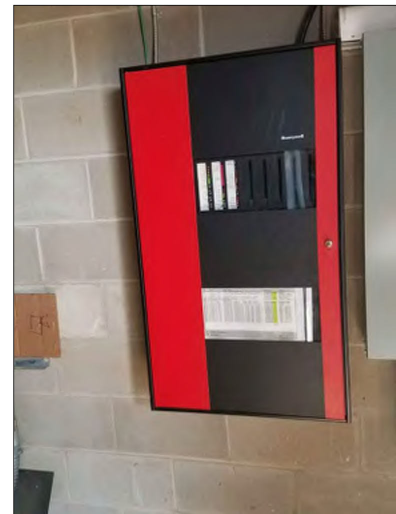
PHOTO A - INTERMEDIARY FIRE ALARM CONTROL PANEL Honeywell FS90 Intermediary Fire Alarm Control Panel Located Within Electrical Room To Be Replaced.
