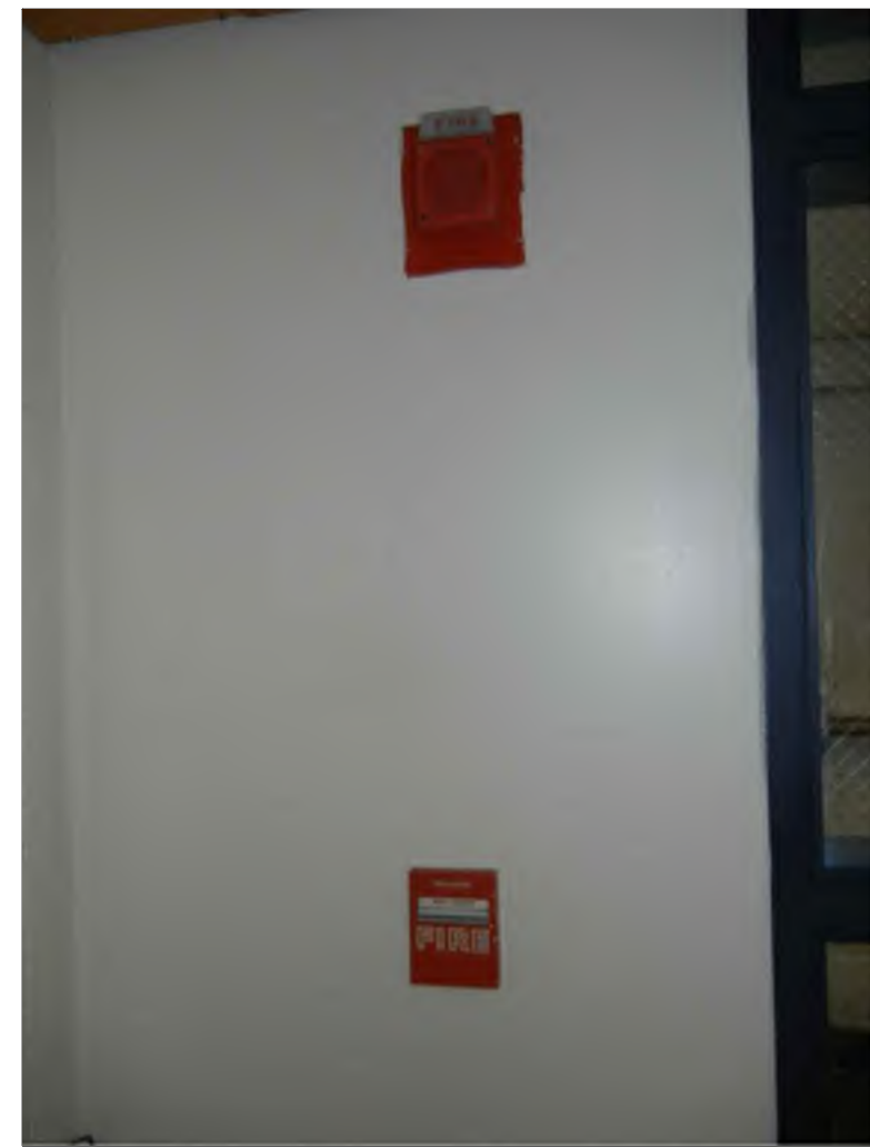
HONEYWELL FIRE ALARM DEVICES Existing Honeywell Addressable Fire Alarm Devices Located Throughout The Building
