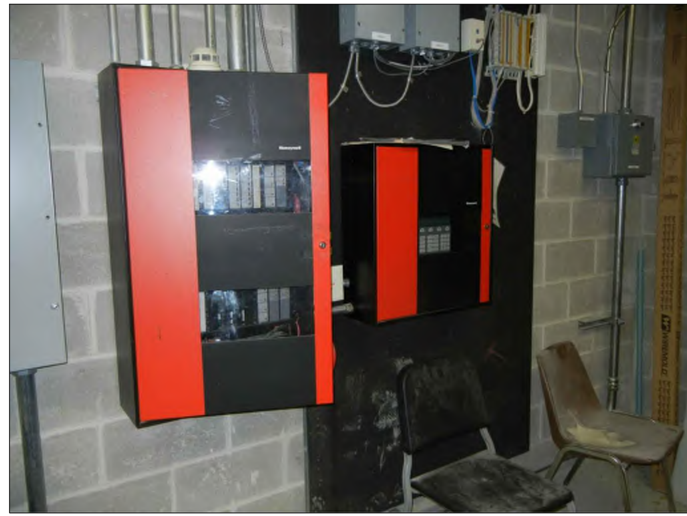
PHOTO A - HONEYWELL FIRE ALARM CONTROL PANEL
