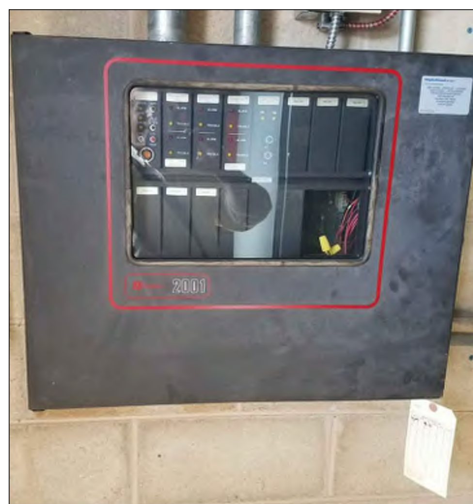
PHOTO B - SIMPLEX FIRE ALARM CONTROL PANEL Simplex 2001 Fire Alarm Control Panel Located Within Electrical Room
