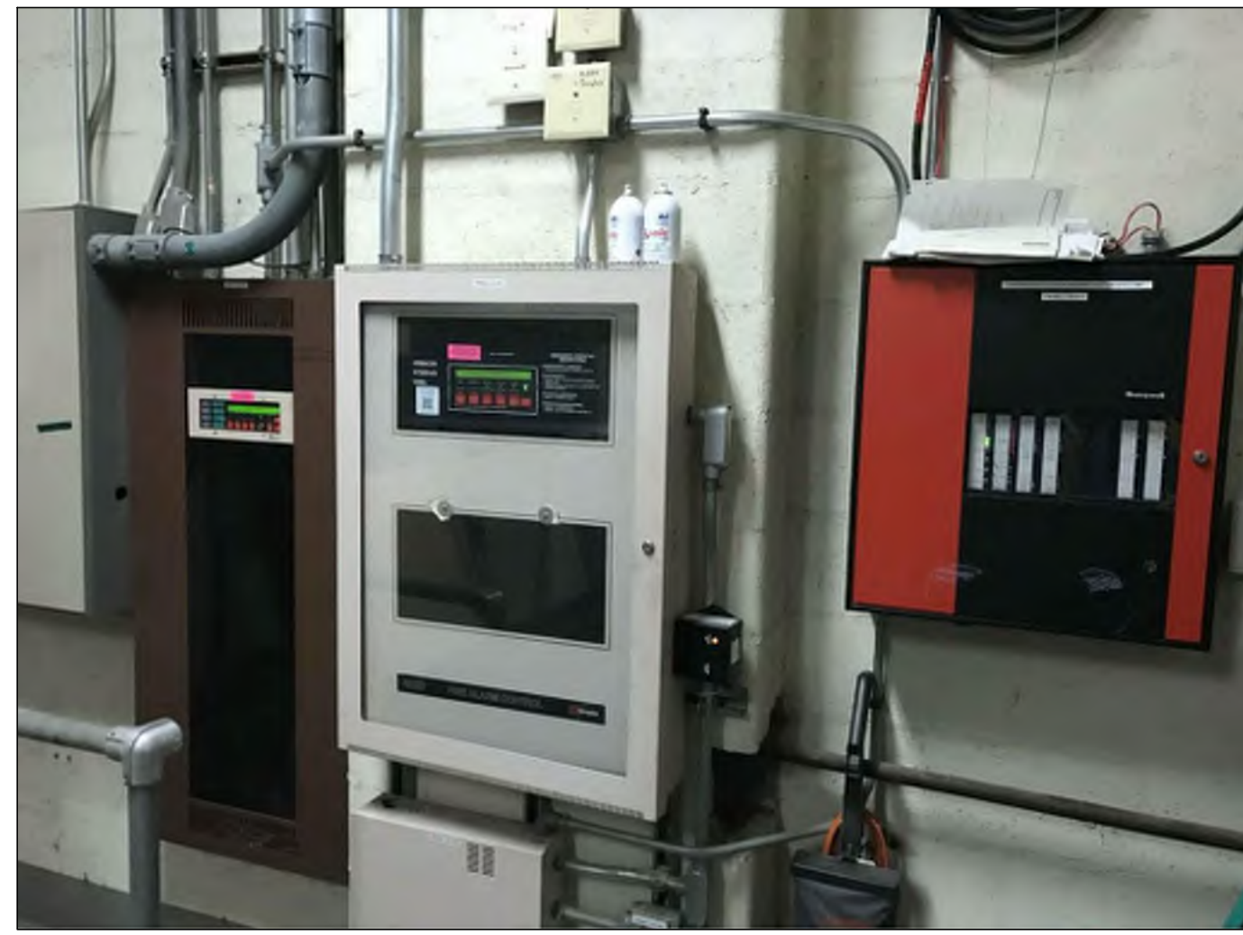
PHOTO A - SIMPLEX FIRE ALARM CONTROL PANEL
