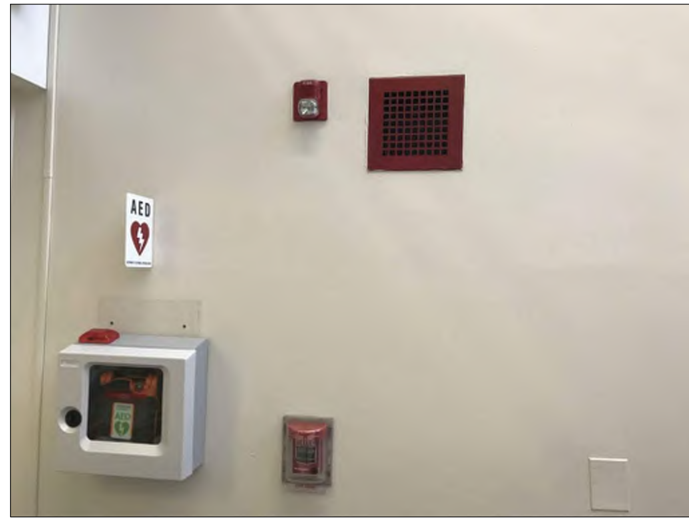
SIMPLEX FIRE ALARM DEVICES
