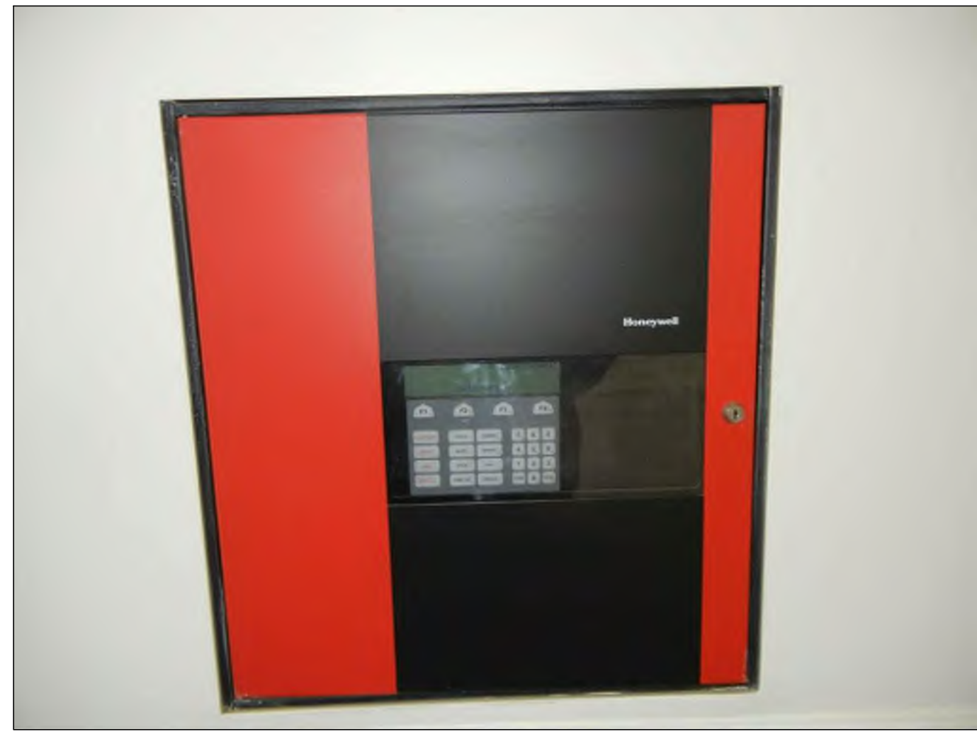
PHOTO A - HONEYWELL FIRE ALARM CONTROL PANEL Honeywell FS90 Addressable Fire Alarm Control Panel Located Within Mechanical Room
