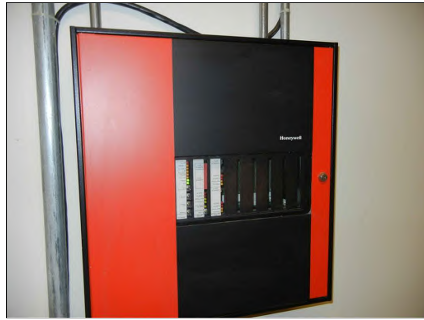
PHOTO B - HONEYWELL FIRE ALARM CONTROL PANEL Existing Honeywell Intermediary Fire Alarm Control Panel With Exposed Conduit Located In The Lower Level Telecom Room
