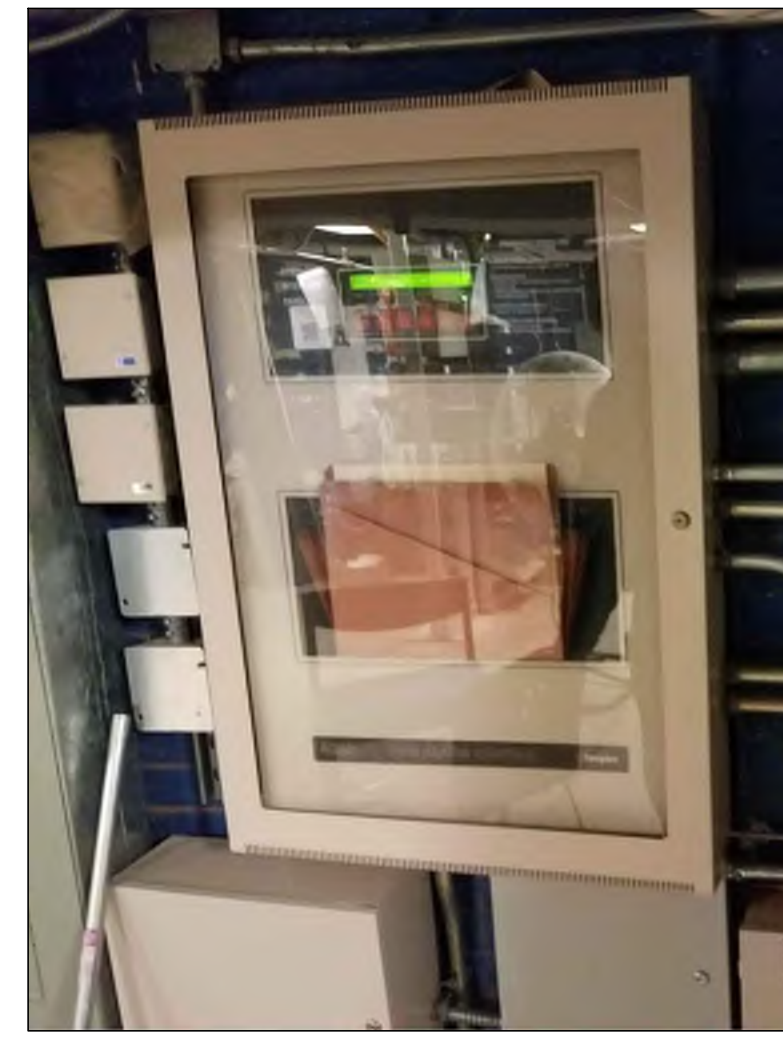
PHOTO B - SIMPLEX FIRE ALARM CONTROL PANEL Simplex 4020 Addressable Fire Alarm Control Panel With Exposed Conduit Located Within Basement Electrical Room.
