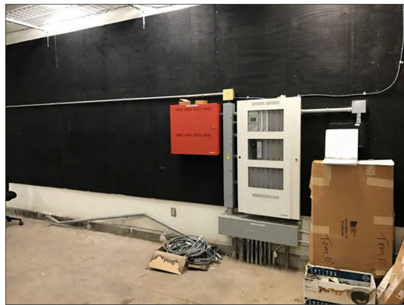
PHOTO A - HONEYWELL FIRE ALARM CONTROL PANEL Honeywell XLS1000 Addressable Fire Alarm Control Panel And Booster Panel With Exposed Conduit Located Within Lower Level Electrical Room
