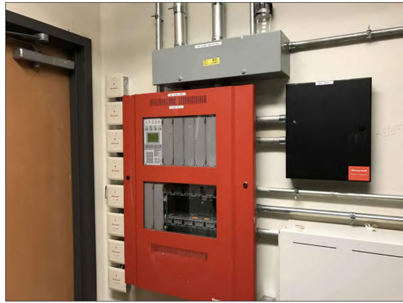
PHOTO A - HONEYWELL FIRE ALARM CONTROL PANEL Honeywell XLS 1000 Addressable Fire Alarm Control Panel With Exposed Conduit Located Within First Floor Electrical Room
