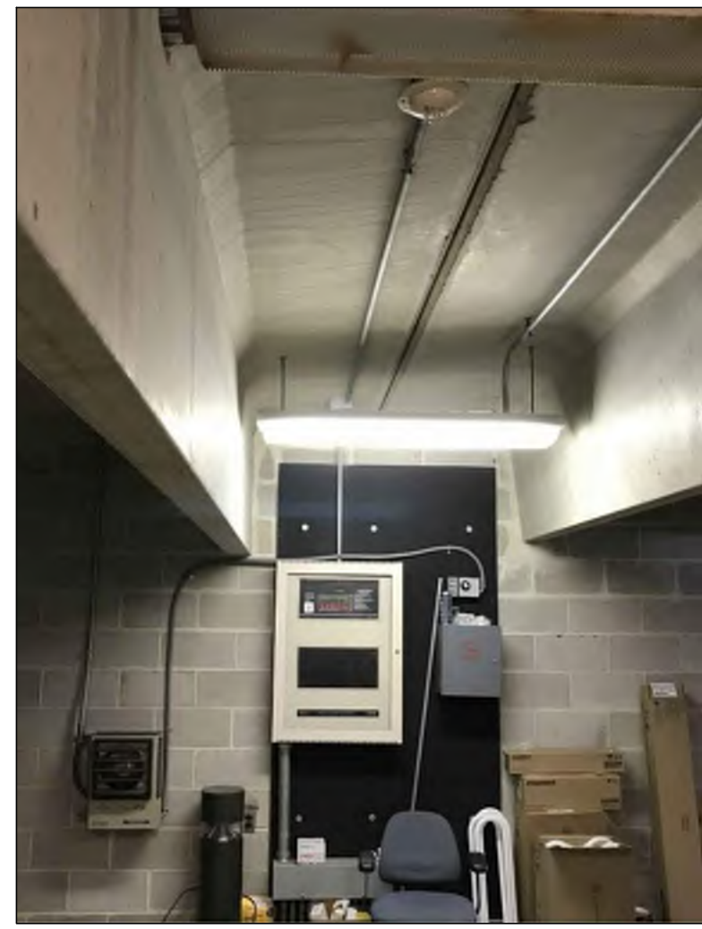
PHOTO A - SIMPLEX FIRE ALARM CONTROL PANEL Simplex 4020 Addressable Fire Alarm Control Panel And Booster Panel With Exposed Conduit Located Within First Floor Electrical Room
