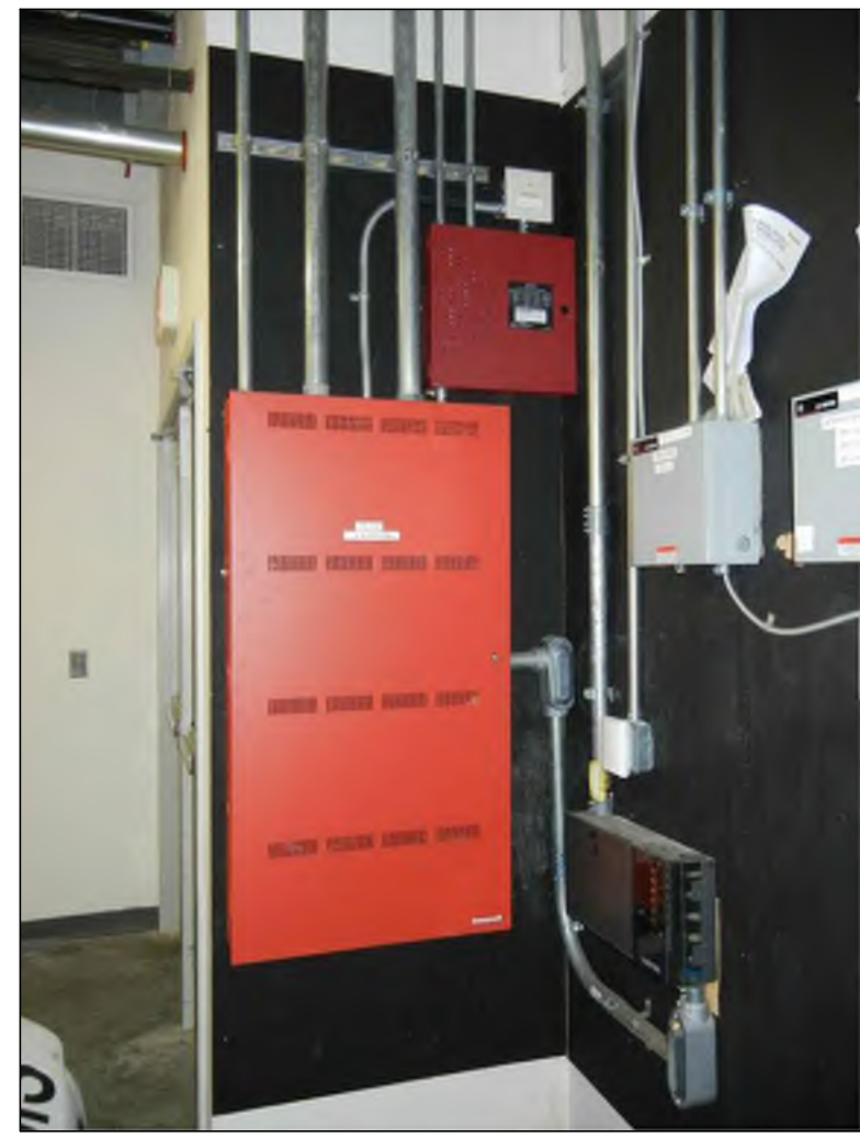
PHOTO A - HONEYWELL FIRE ALARM CONTROL PANEL Honeywell XLS 1000 Addressable Fire Alarm Control Panel and Booster Panel With Exposed Conduit Located Within Lower Level Electrical Room
