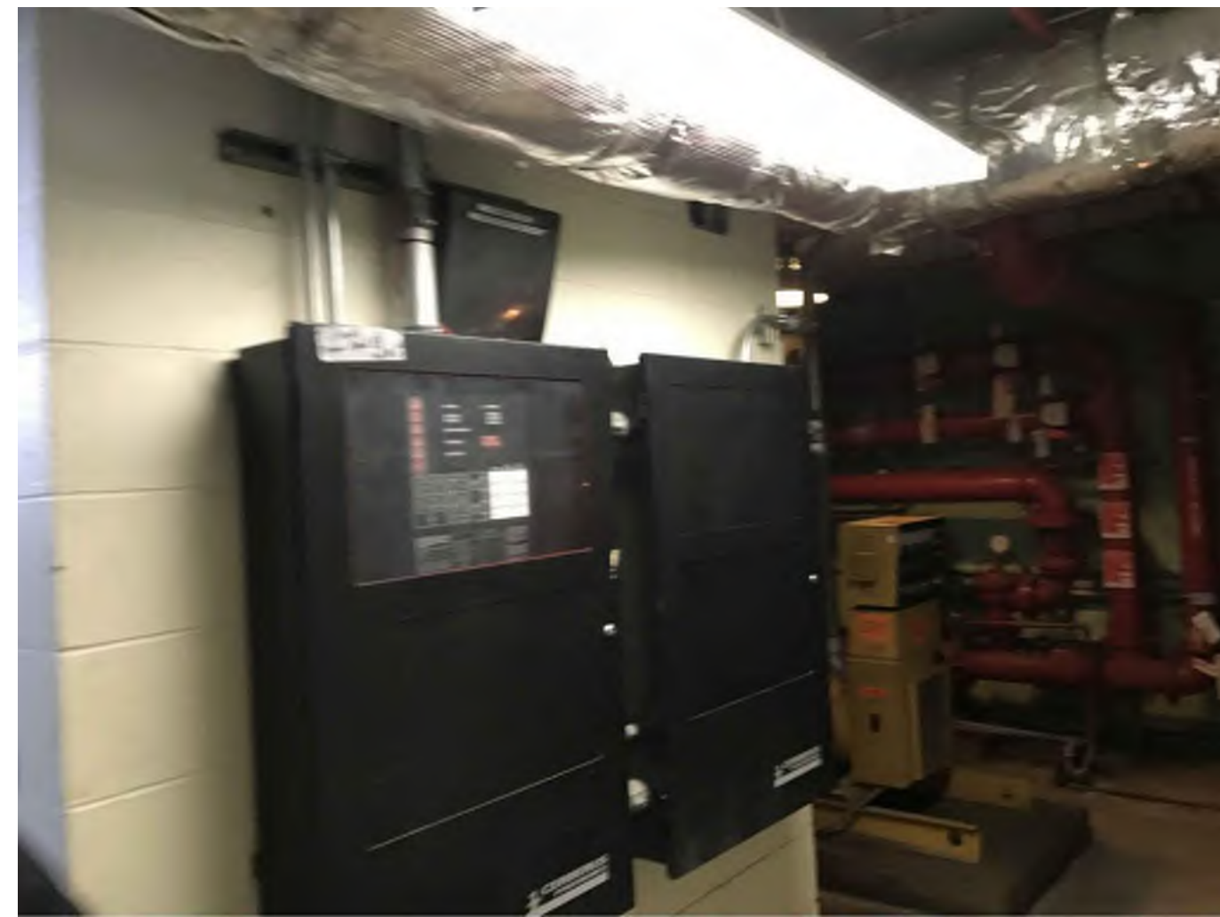
PHOTO B - SIEMENS FIRE ALARM CONTROL PANEL Siemens MXL Addressable Fire Alarm Control Panel With Exposed Conduit Located Within Lower Level Generator Room
