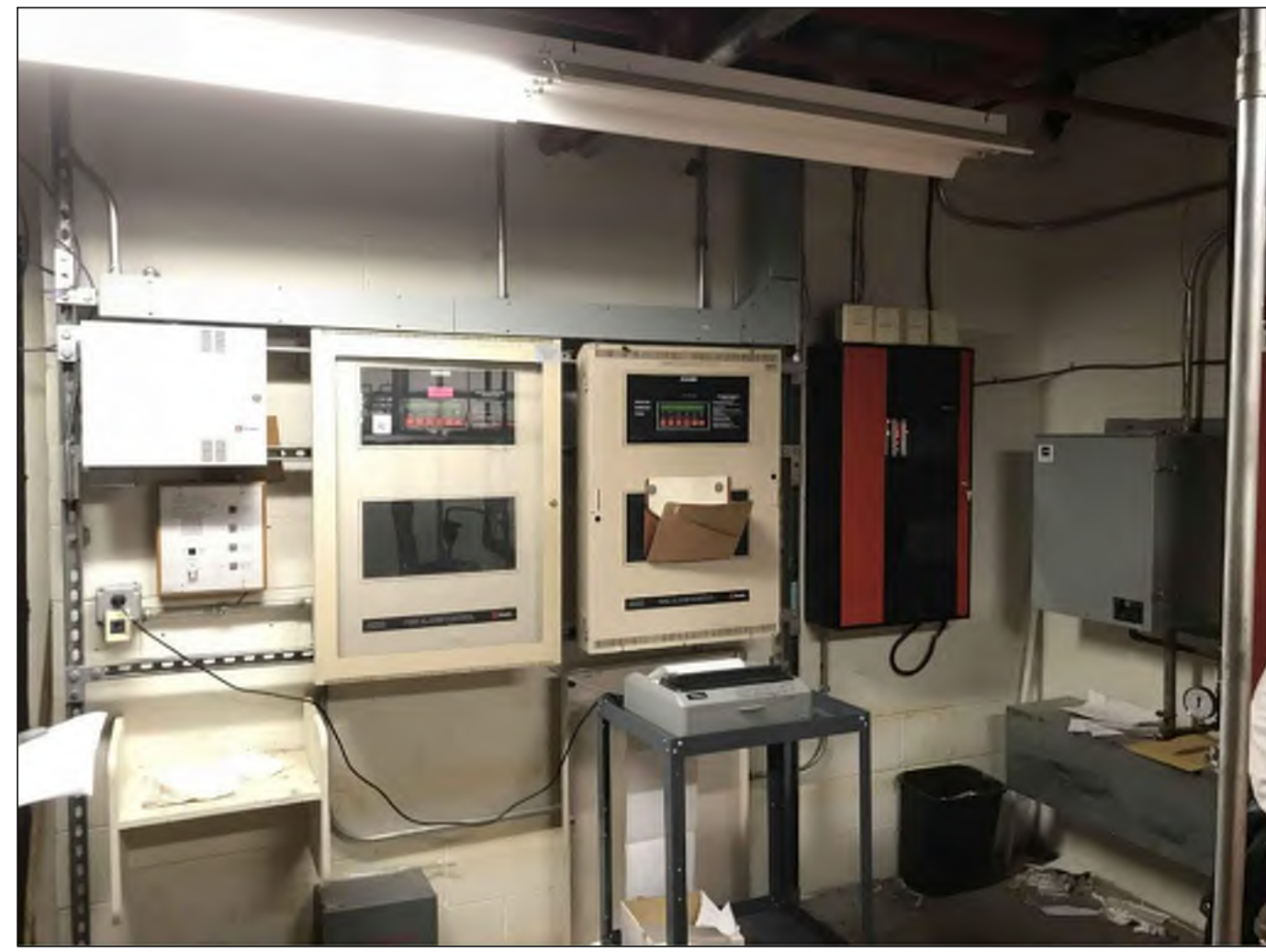
PHOTO A - SIMPLEX FIRE ALARM CONTROL PANEL Simplex 4020 Addressable Fire Alarm Control Panel And Honeywell FS90 Intermediary Fire Alarm Control Panel With Exposed Conduit Located Within Lower Level Fire Pump Room
