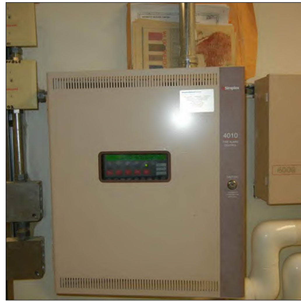
PHOTO A - SIMPLEX FIRE ALARM CONTROL PANEL Simplex 4010 Addressable Fire Alarm Control Panel With Exposed Conduit Located Within Lower Level Electrical Room
