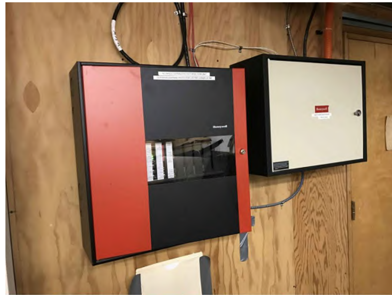
PHOTO A - INTERMEDIARY FIRE ALARM CONTROL PANEL Honeywell FS90 Intermediary Fire Alarm Control Panel With Exposed Conduit Located Within Lower Level Storage Room
