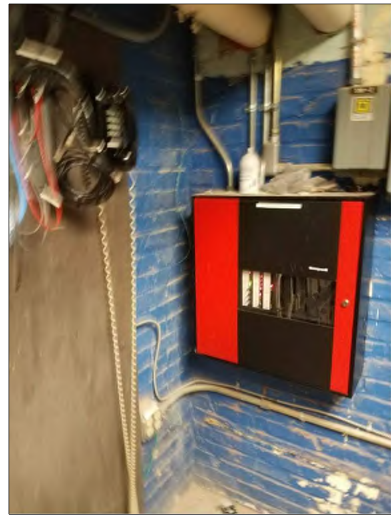
PHOTO A - INTERMEDIARY FIRE ALARM CONTROL PANEL Honeywell FS90 Intermediary Fire Alarm Control Panel With Exposed Conduit Located Within Basement Electrical Room.
