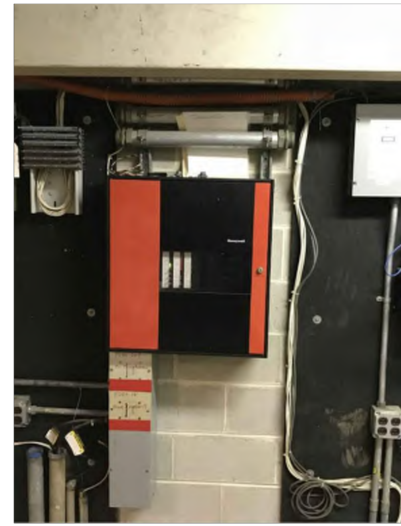
PHOTO B - INTERMEDIARY FIRE ALARM CONTROL PANEL Honeywell FS90 Intermediary Fire Alarm Control Panel And Booster Panel With Exposed Conduit Located Within First Floor Electrical Room
