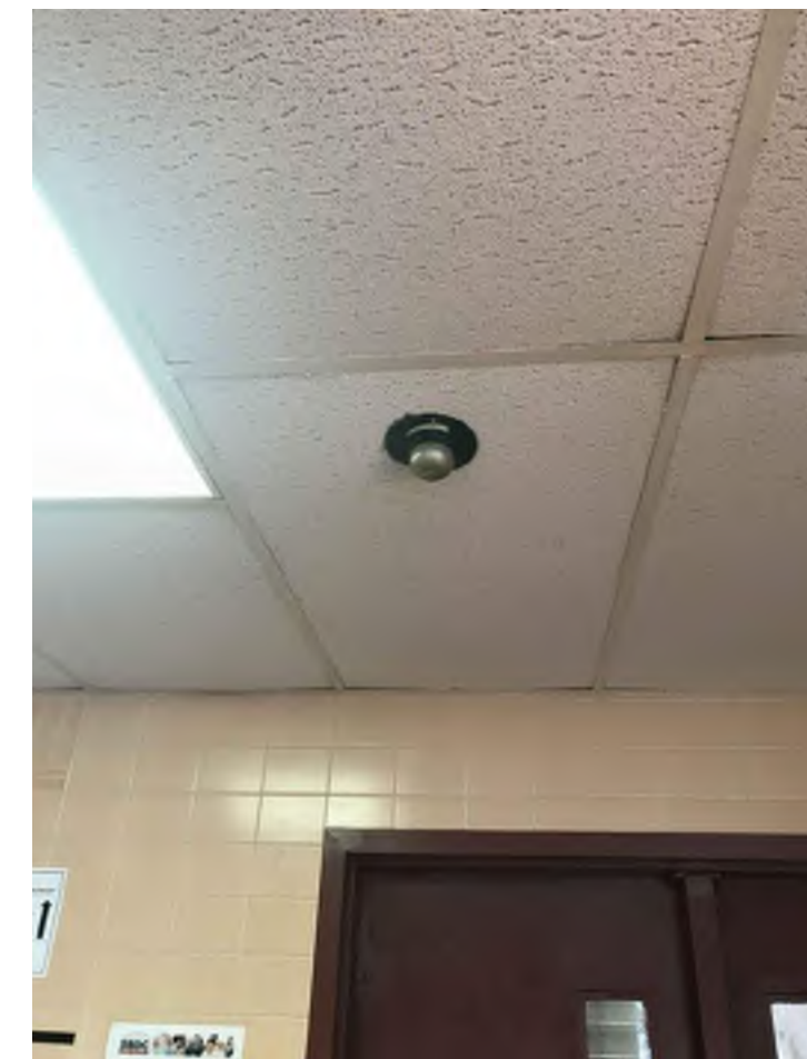
PHOTO F - HEAT DETECTION Typical Ceiling Mounted Heat Detectors Located Throughout Building To Be Demolished
