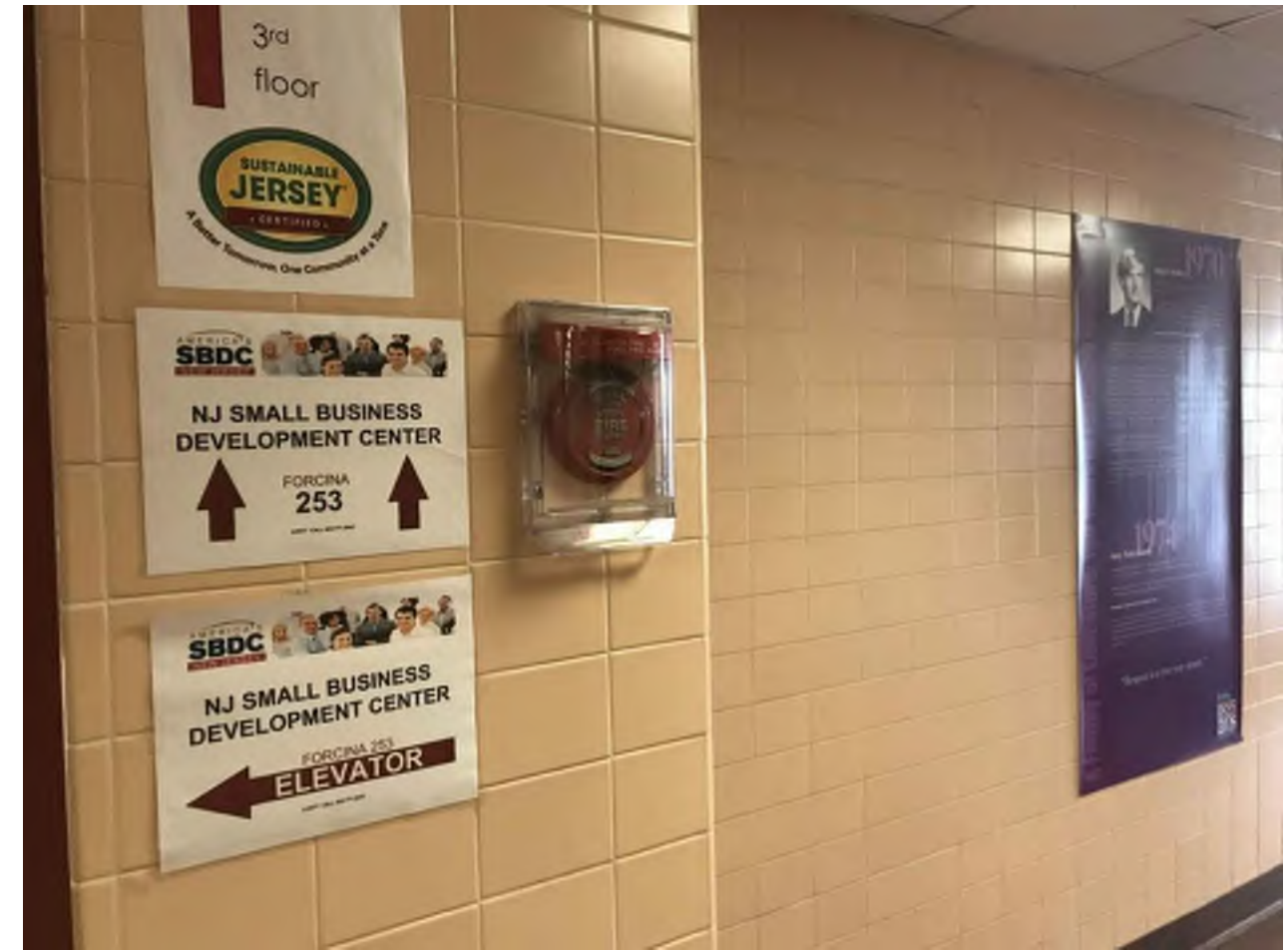
PHOTO C - MANUAL FIRE ALARM INITIATION Typical Pull Stations With Protective Cover Located Within Corridors To Be Demolished
