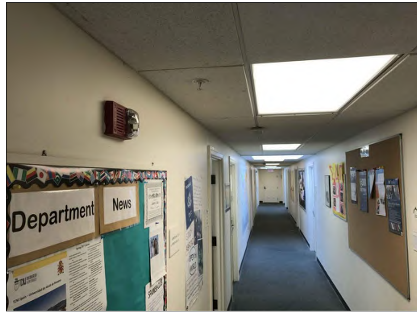
SIMPLEX FIRE ALARM DEVICES Existing Simplex Addressable Fire Alarm Devices Located Throughout The Building
