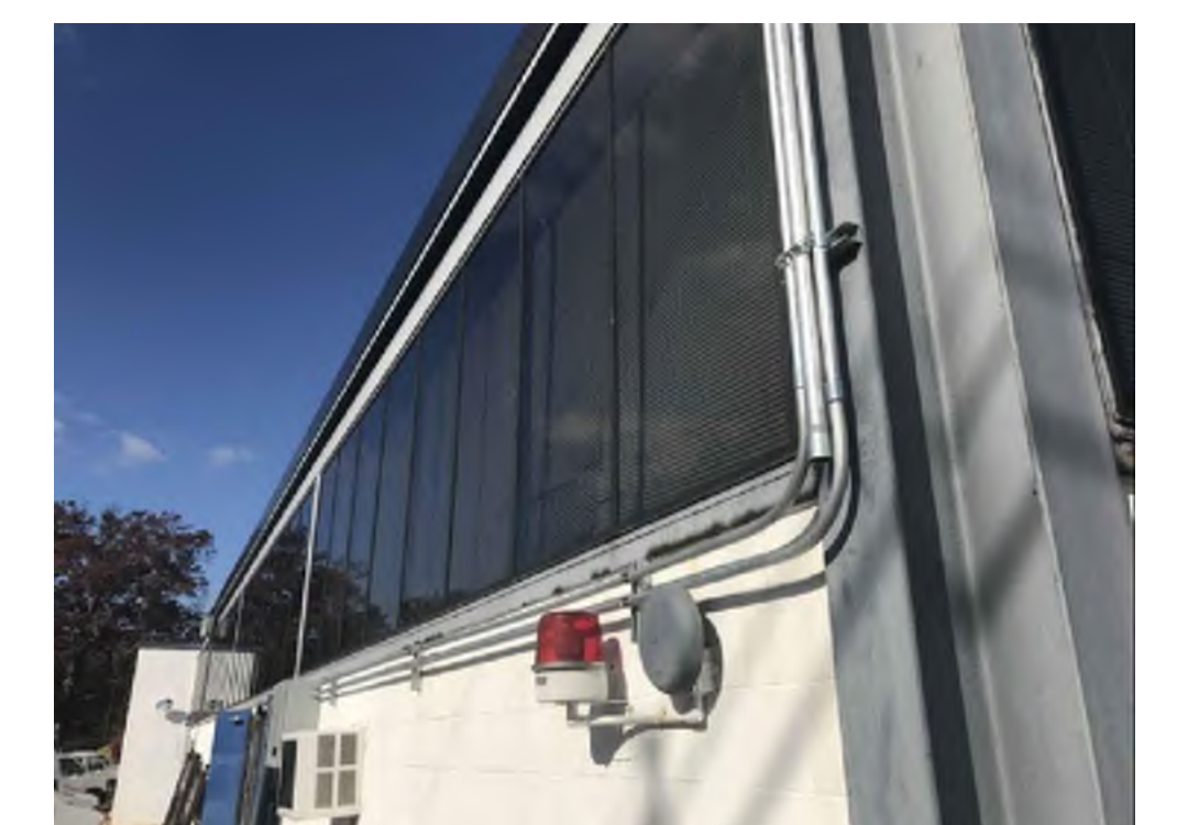
PHOTO H - EXTERIOR Bell And Beacon To Be Demolished
