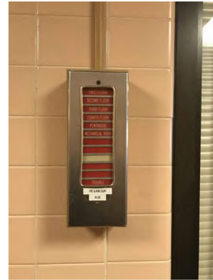
PHOTO A - FIRE ALARM ANNUNCIATOR Fire Alarm Annunciator Located Within Corridor To Be Demolished
