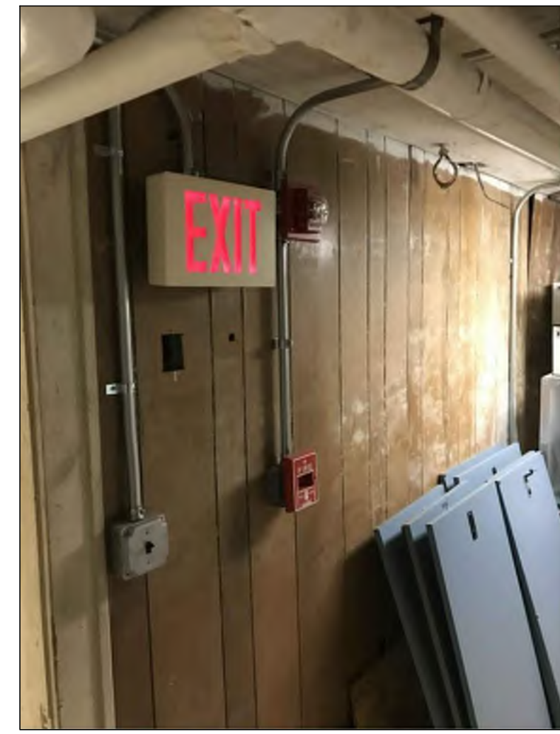
SIEMENS FIRE ALARM DEVICES Existing Siemens Addressable Fire Alarm Devices Located Throughout The Building
