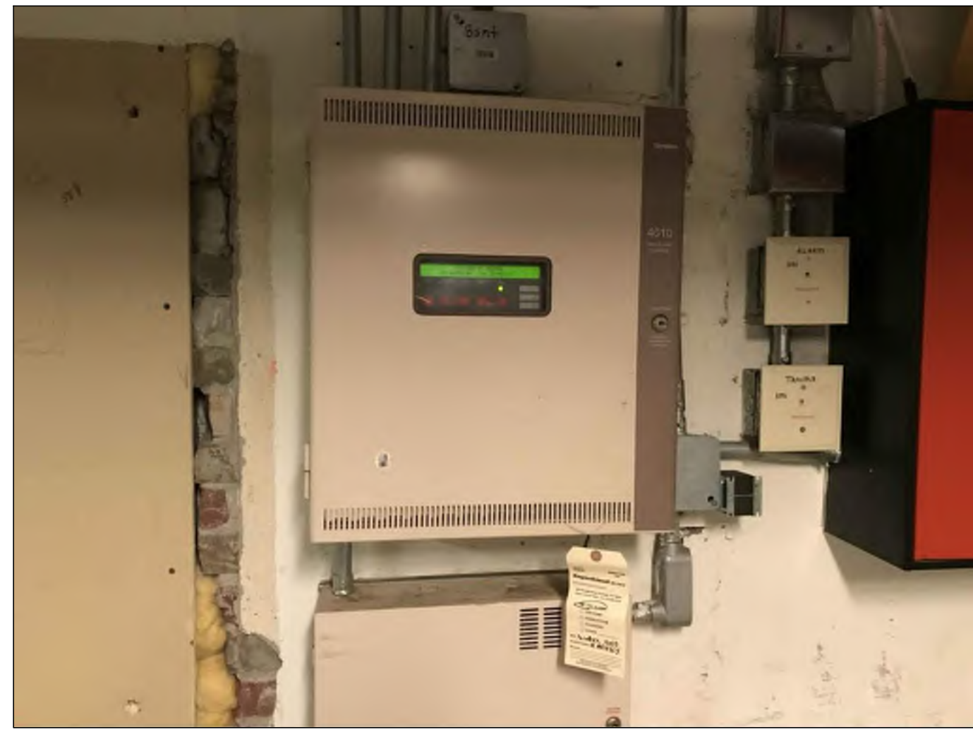
PHOTO A - SIMPLEX FIRE ALARM CONTROL PANEL Simplex 4010 Addressable Fire Alarm Control Panel With Exposed Conduit Located Within Lower Level Electrical Room
