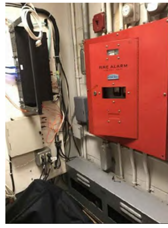
PHOTO A - FIRE ALARM PANEL Standard Time Fire Alarm Control Panel To Be Demolished
