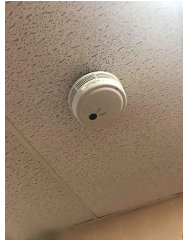
PHOTO B - SMOKE DETECTION Typical Smoke Detectors For Elevator Recall To Be Demolished
