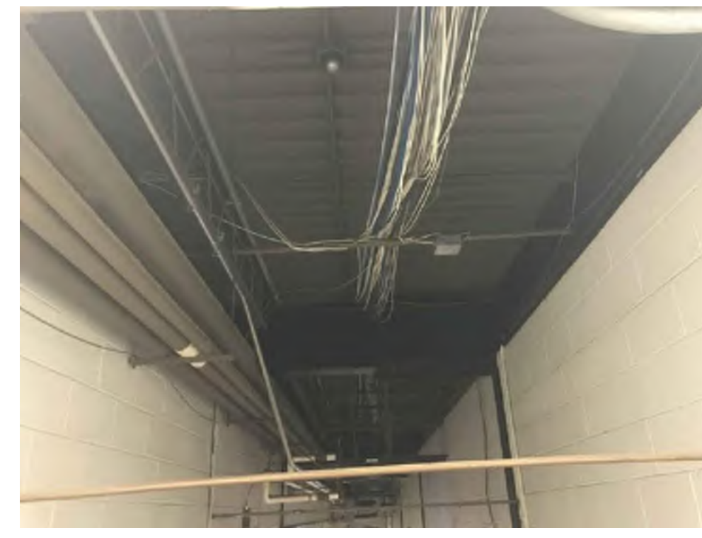
PHOTO C - CORRIDOR Open Ceiling Maintenance Corridor Heat Detectors To Be Demolished
