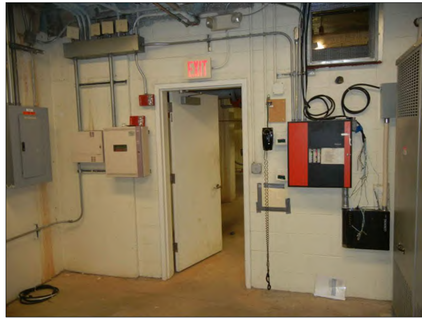
PHOTO A - SIMPLEX FIRE ALARM CONTROL PANEL Simplex 4010 Addressable Fire Alarm Control Panel And Honeywell FS/90 Intermediary Fire Alarm Control Panel With Exposed Conduit Located Within Lower Level Electrical Room
