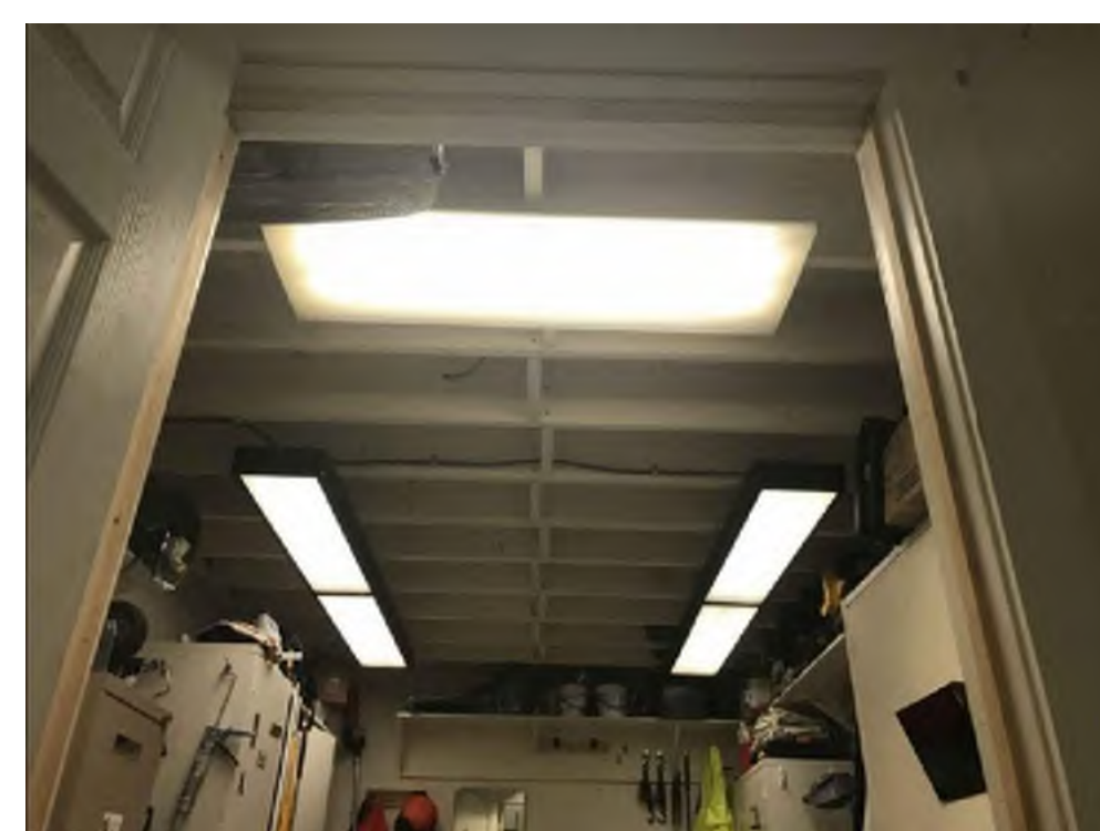
PHOTO F - MEZZANINE AREA Storage Area Below Mezzanine Area To Be Demolished
