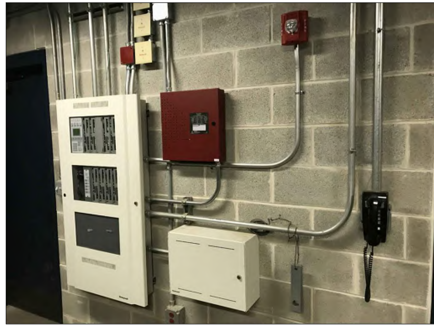
PHOTO A - HONEYWELL FIRE ALARM CONTROL PANEL Honeywell XLS1000 Addressable Fire Alarm Control Panel With Exposed Conduit Located Within Lower Level Electrical Room
