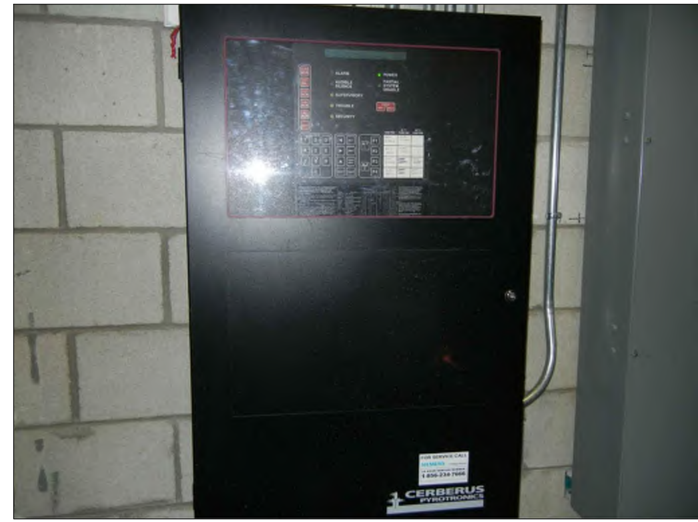
PHOTO A - SIEMENS FIRE ALARM CONTROL PANEL Existing Siemens MXL Addressable Fire Alarm Control Panel With Exposed Conduit Located Within Lower Level Mechanical Room
