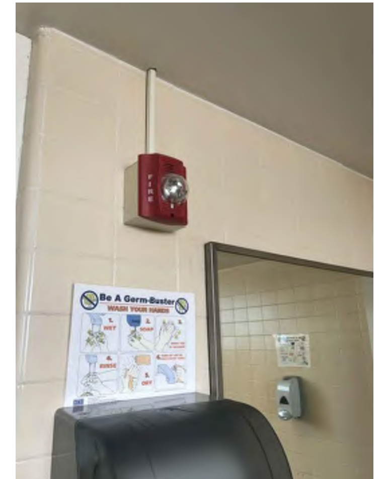
PHOTO E - HORN AND STROBES Typical Horns / Strobe Located Throughout Building To Be Demolished
