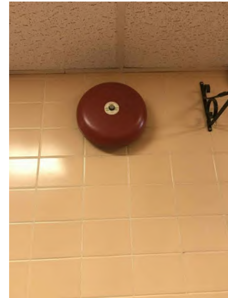
PHOTO D - NOTIFICATION Typical Wall Mounted Bells Located Throughout Building To Be Demolished
