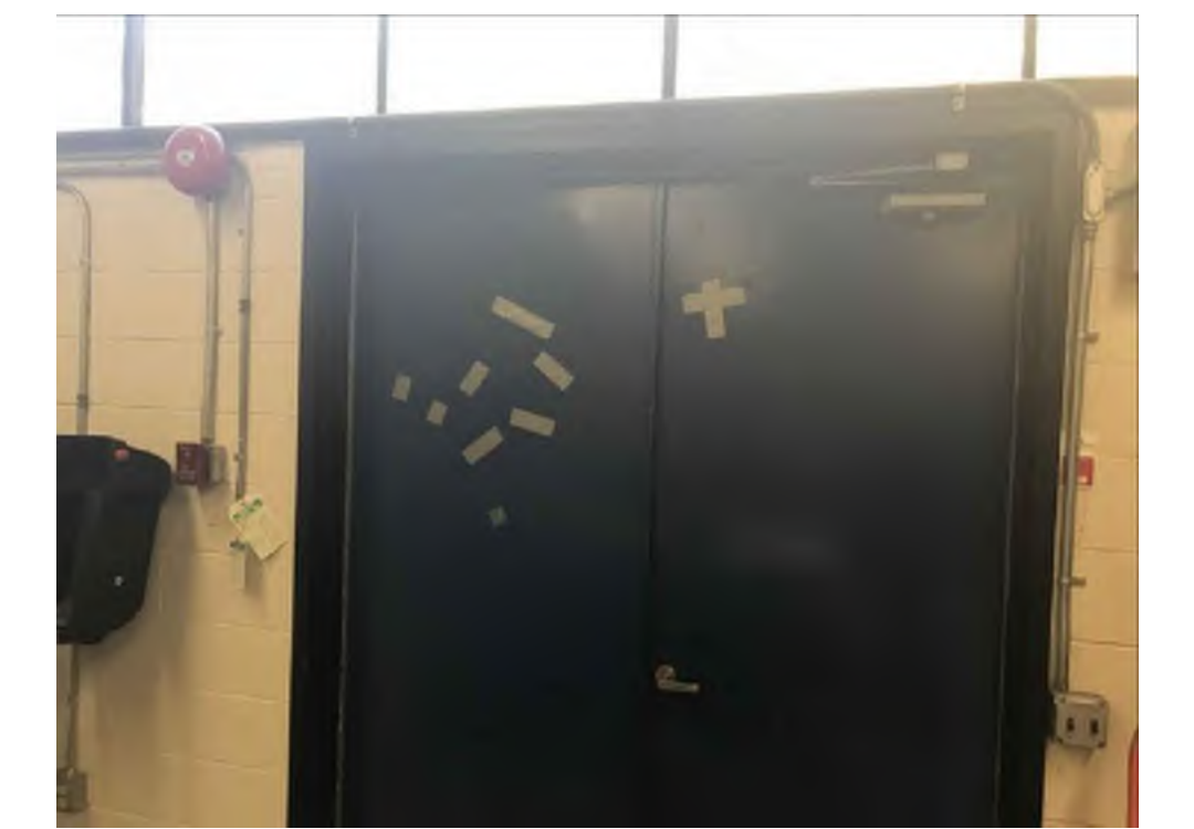
PHOTO D - SHOP Shop Area Pull Stations And Bell Notification To Be Demolished
