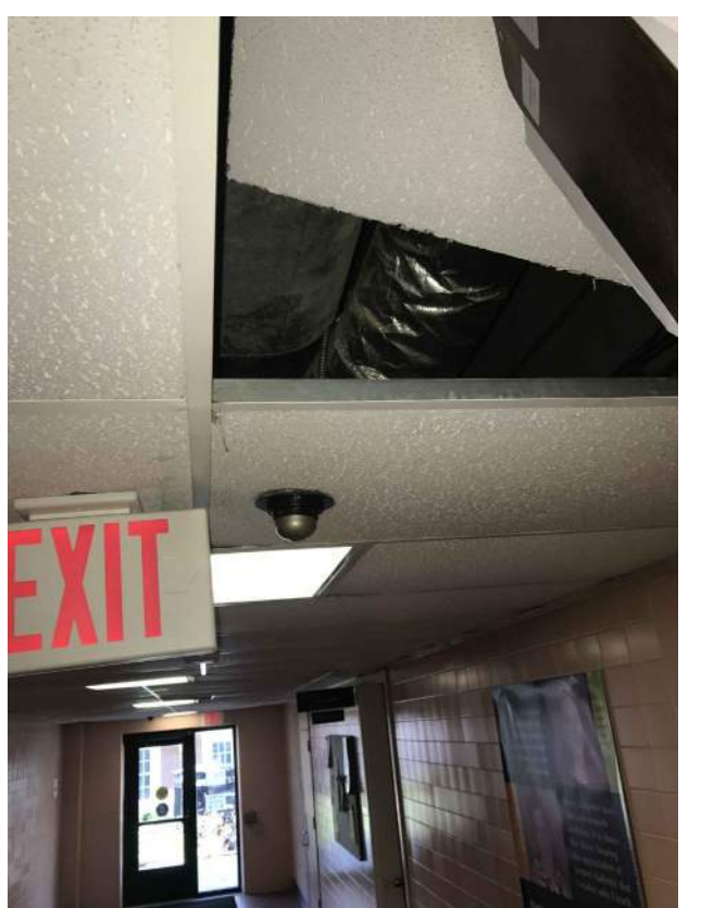
PHOTO B - EXISTING CORRIDOR CEILING Route Fiber Pathway Above Existing Drop Ceilings Within Corridor
