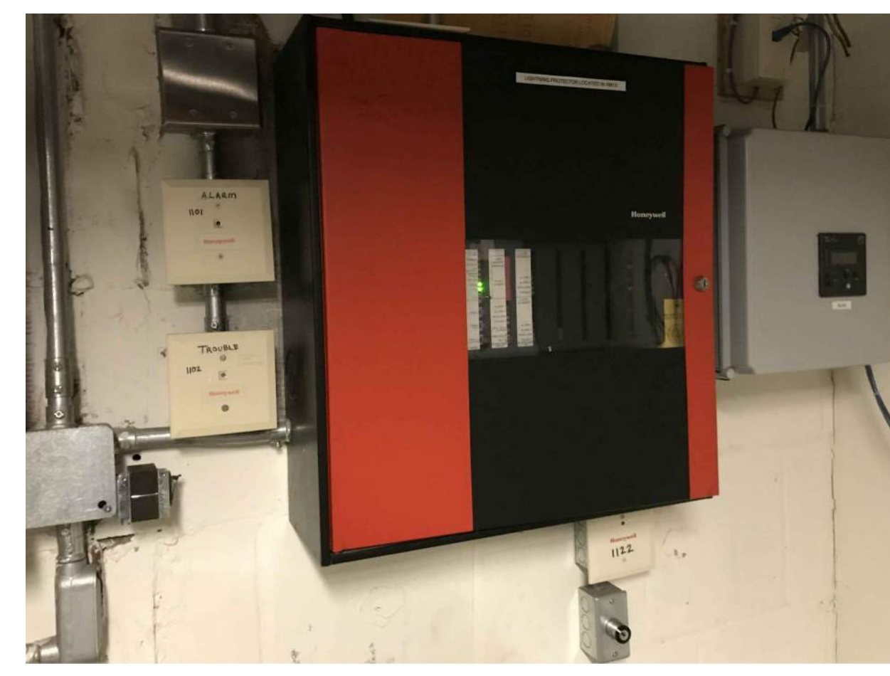
PHOTO A - EXISTING FIRE ALARM PANEL Existing Fire Alarm Control Panel
