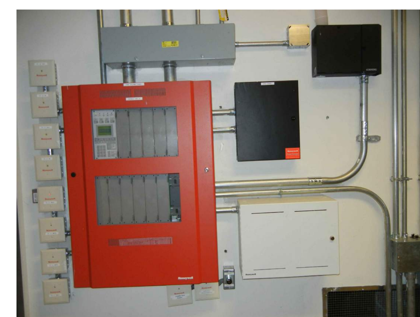
PHOTO C - FIRE ALARM CONTROL PANEL Fire Alarm Control Panel With Exposed Conduit Located Within First Floor Electrical Room
