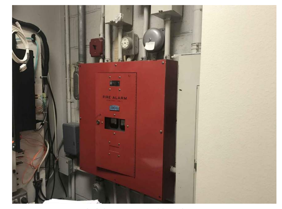
PHOTO C - FIRE ALARM CONTROL PANEL Existing Fire Alarm Control Panel With Exposed Conduit Located Within Electrical Room
