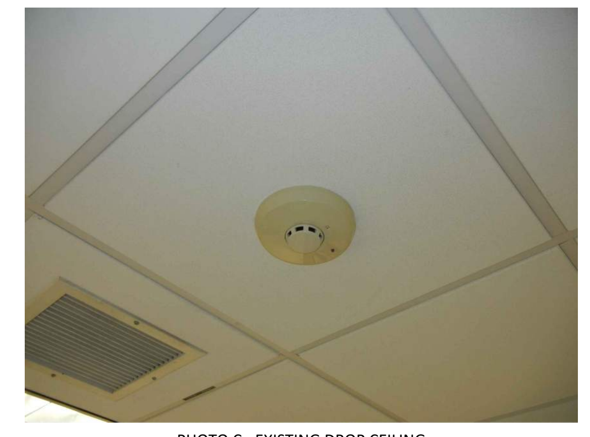
PHOTO C - EXISTING DROP CEILING Route Fiber Pathway Above Existing Drop Ceilings With The Corridor
