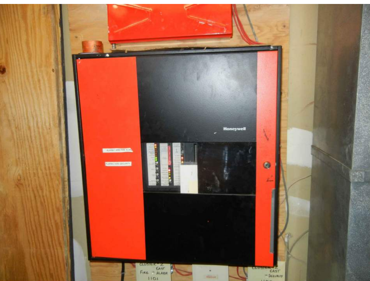
PHOTO D - EXISTING FIRE ALARM PANEL Existing Fire Alarm Control Panel Location
