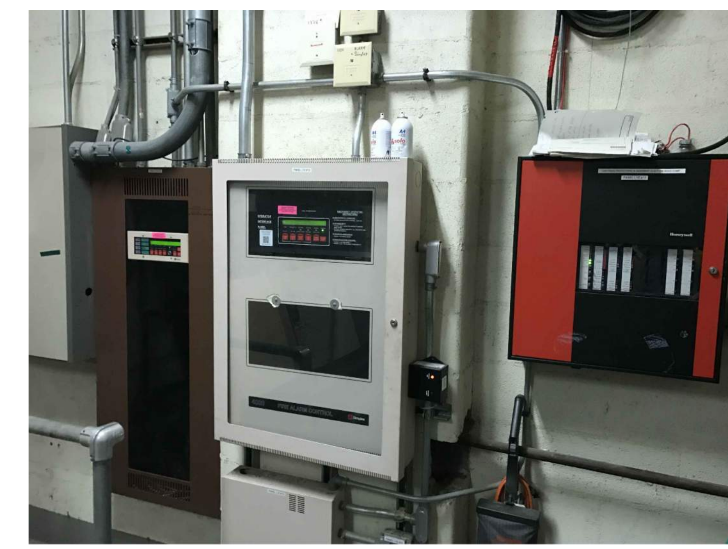
PHOTO A - FIRE ALARM CONTROL PANELS Fire Alarm Control Panels And Fire Alarm Remote Annunciator With Exposed Conduit Located Within First Floor Electrical Room
