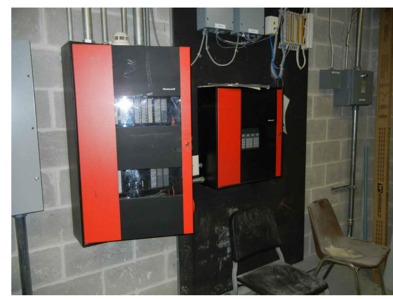
PHOTO B - EXISTING FIRE ALARM PANEL Existing Fire Alarm Control Panel Location
