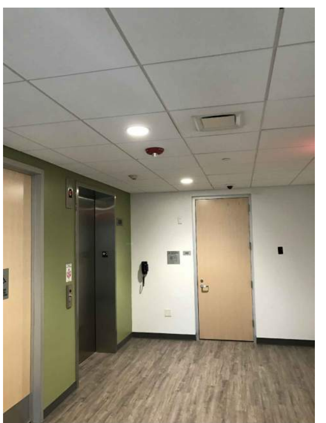
PHOTO C - EXISTING CONDITIONS Fiber Routing Location And Existing Drop Ceiling Conditions
