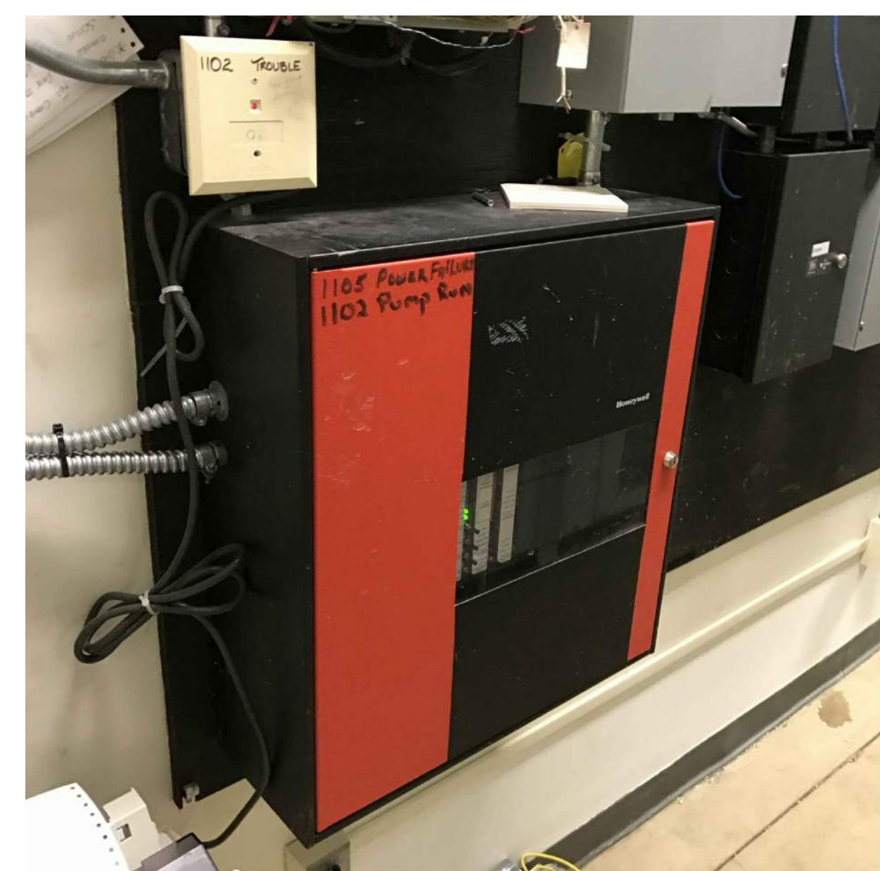
PHOTO B - FIRE ALARM CONTROL PANEL Existing Fire Alarm Control Panel
