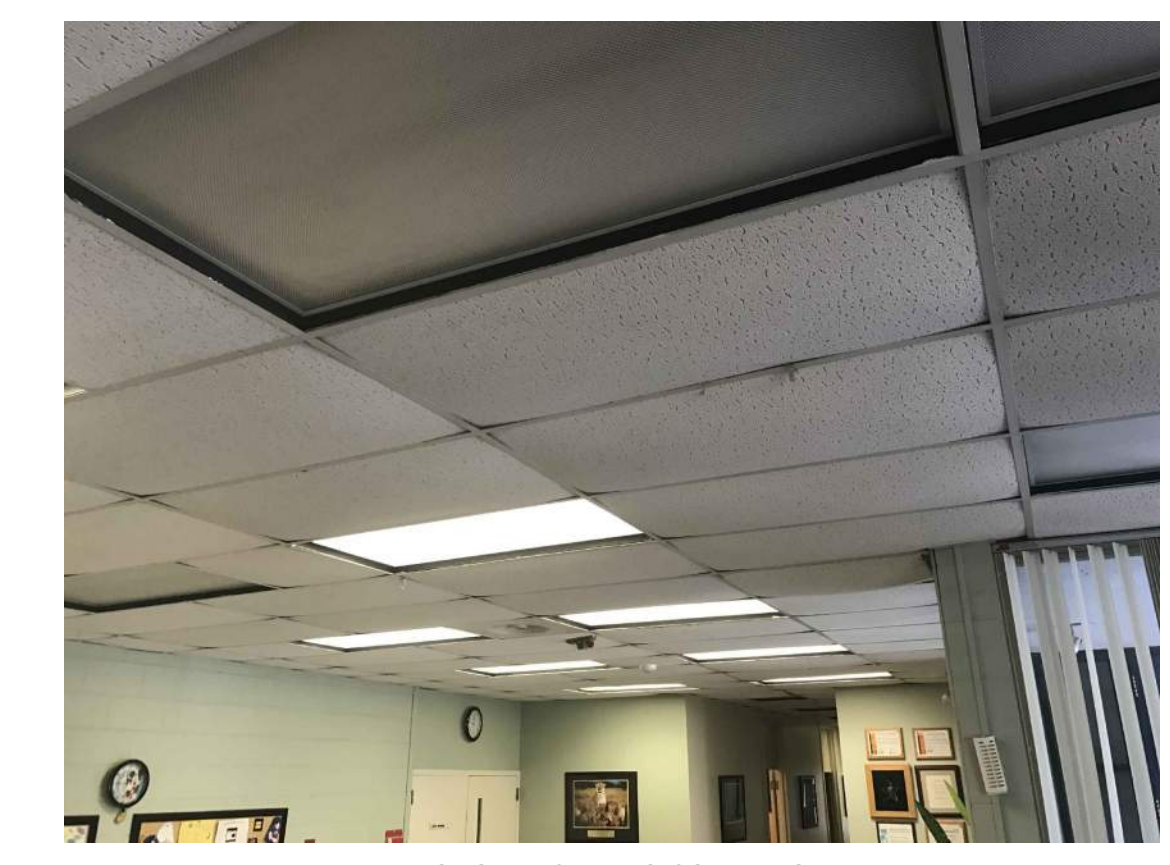
PHOTO D - CEILING CONDITION Drop Ceiling Located Throughout The Office Area And Corridor
