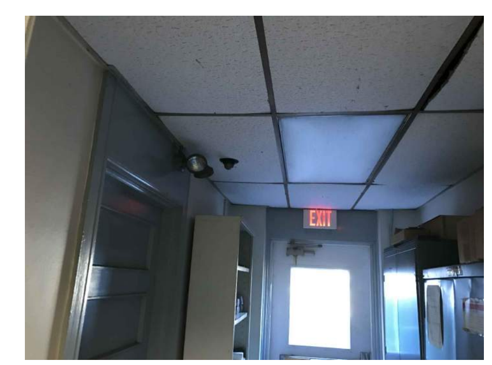
PHOTO B - EXISTING CEILING CONDITIONS Route Fiber Pathway Above Drop Ceiling Located Throughout First Floor
