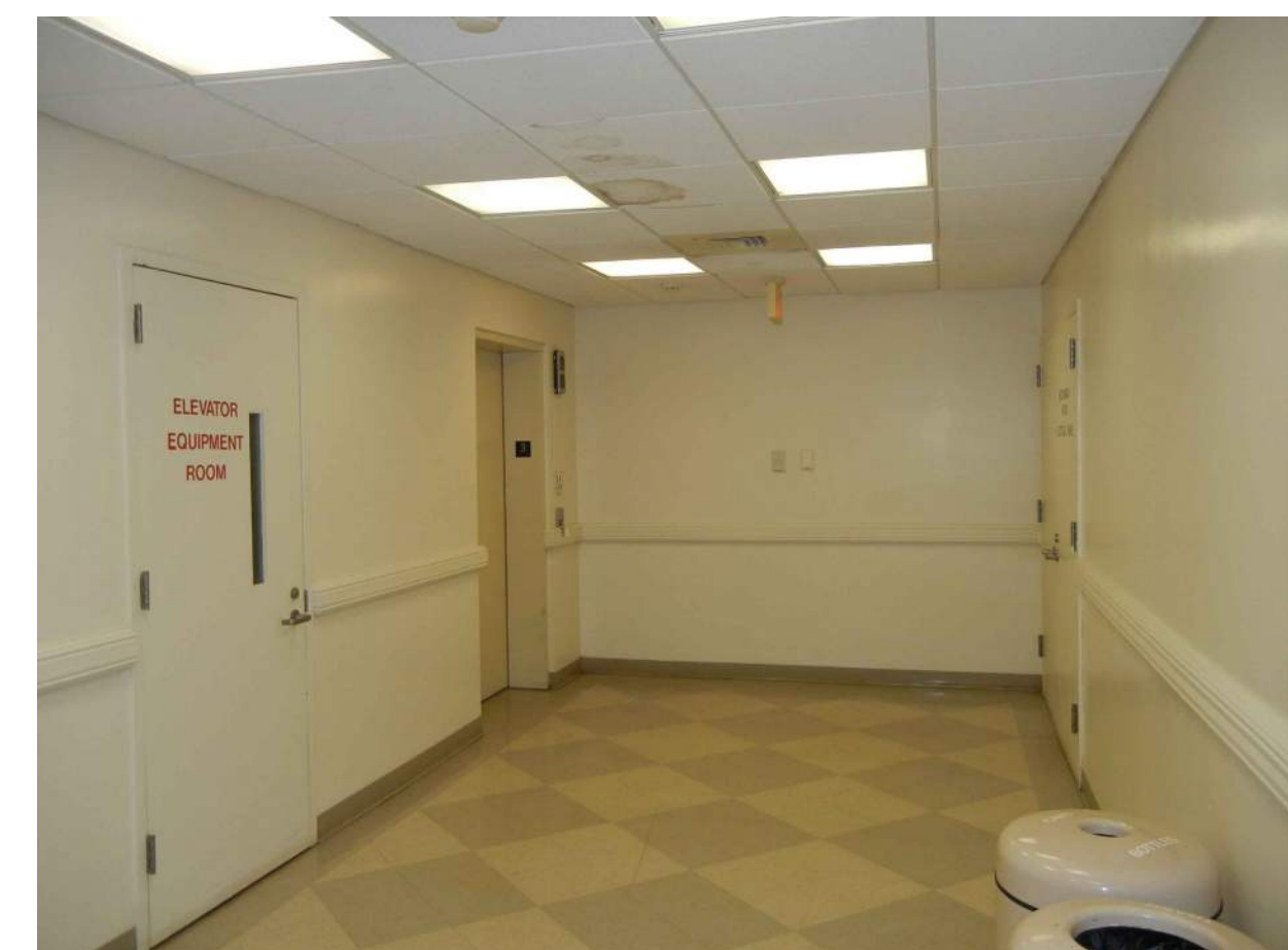
BUILDING CEILINGS Drop Ceilings Located Throughout The Building. Route Fiber Pathway Above Existing Drop Ceilings
