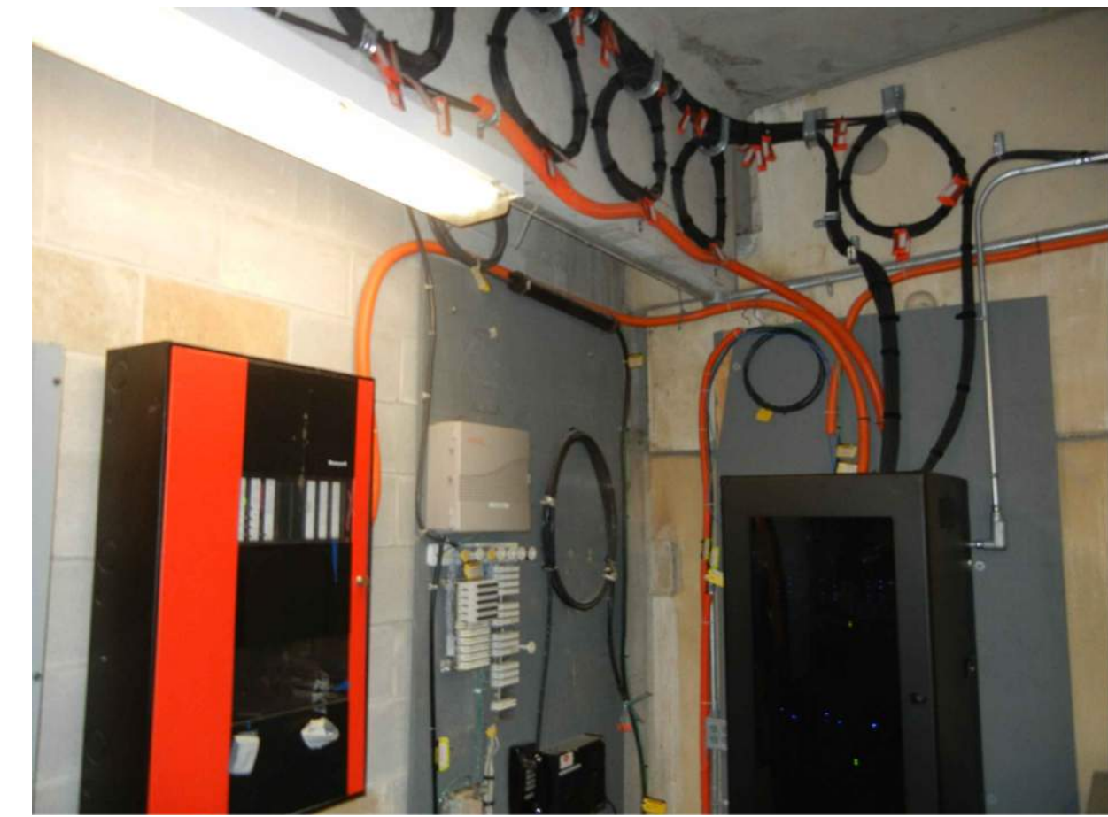
PHOTO A - EXISTING FIRE ALARM PANEL Existing Fire Alarm Control Panel Location
