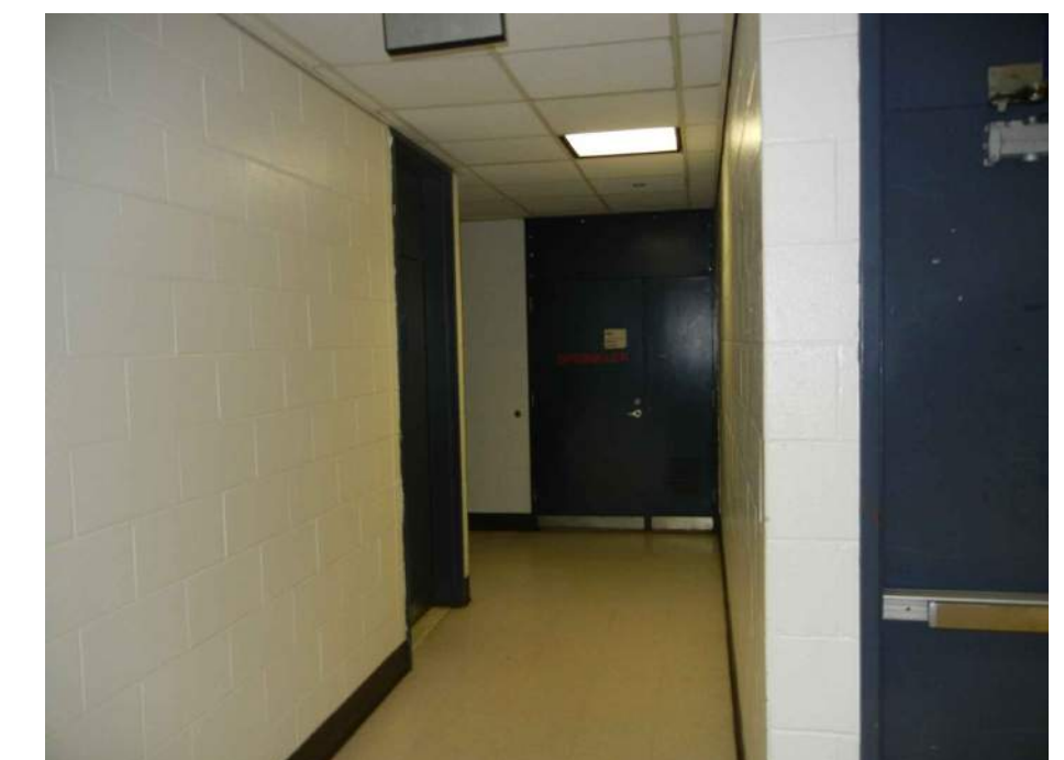
PHOTO D - BASEMENT CEILING Route Fiber Pathway Above Existing Basement Drop Ceiling
