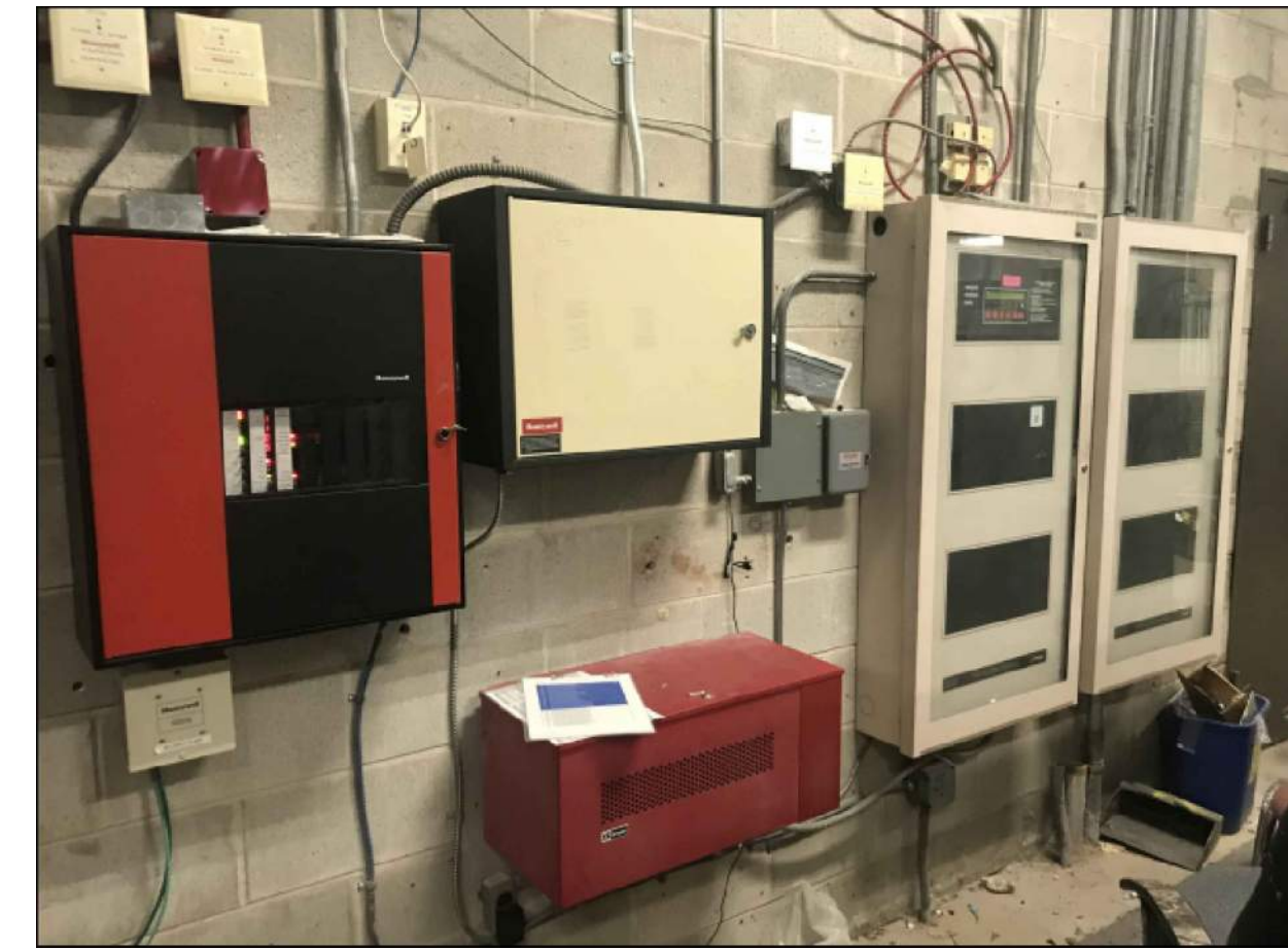
PHOTO A - FIRE ALARM CONTROL PANEL Existing Fire Alarm Control Panel
