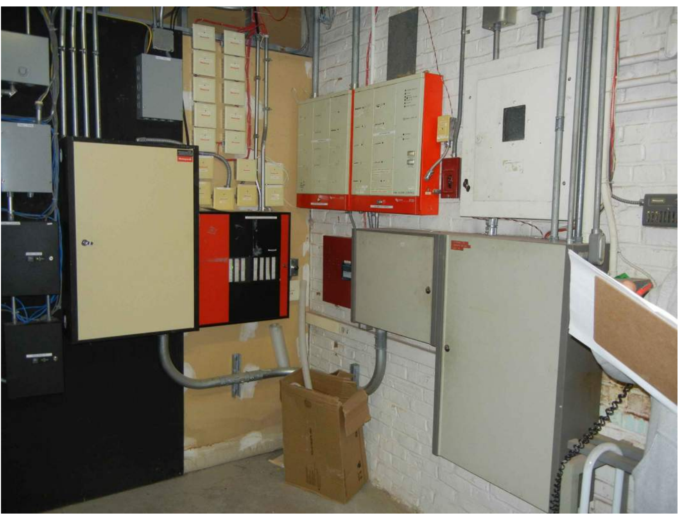
PHOTO D - FIRE ALARM CONTROL PANEL Existing Fire Alarm Control Panel With Exposed Conduit Located Within Lower Level Electrical Room
