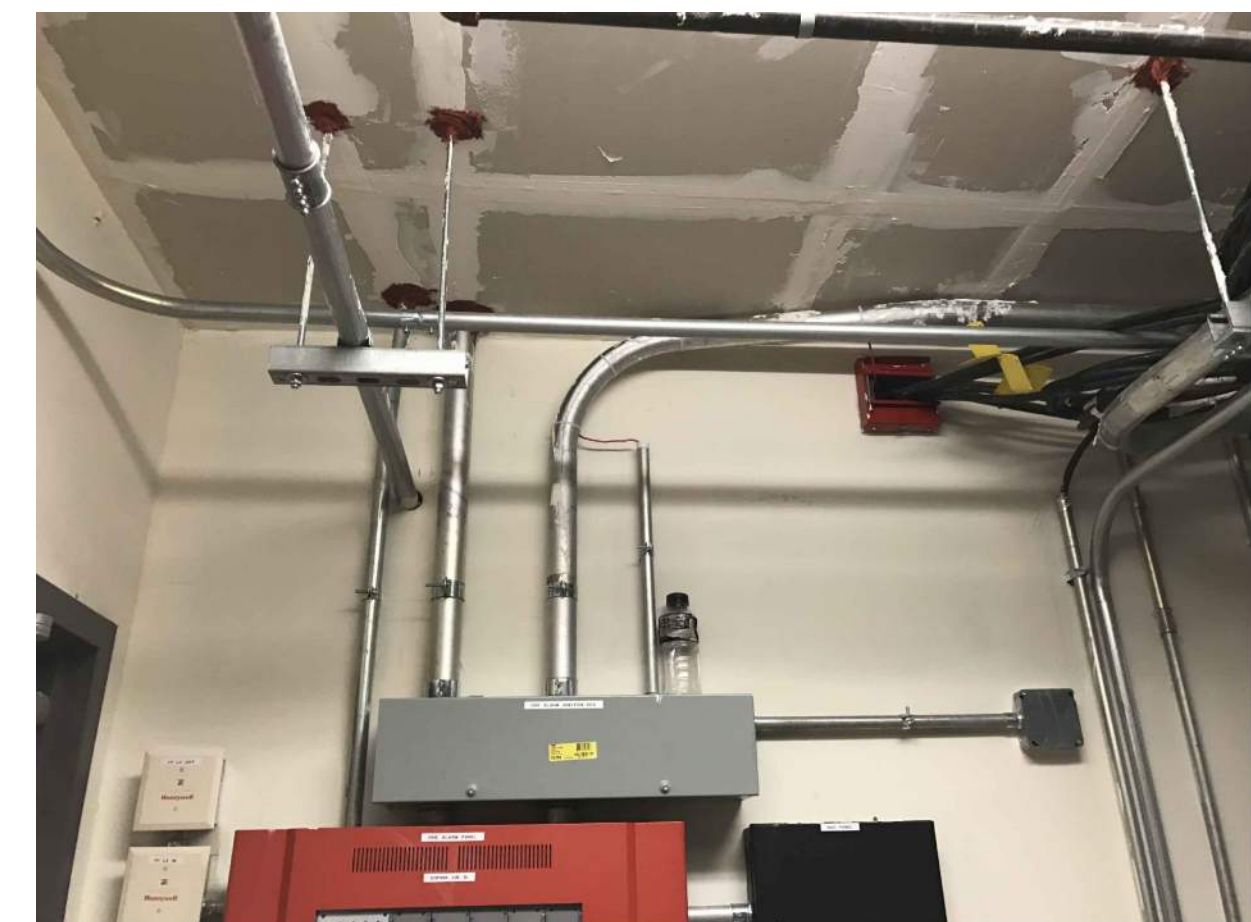
PHOTO B - BASEMENT CEILING Open Ceiling In Basement Room 108 And 110
