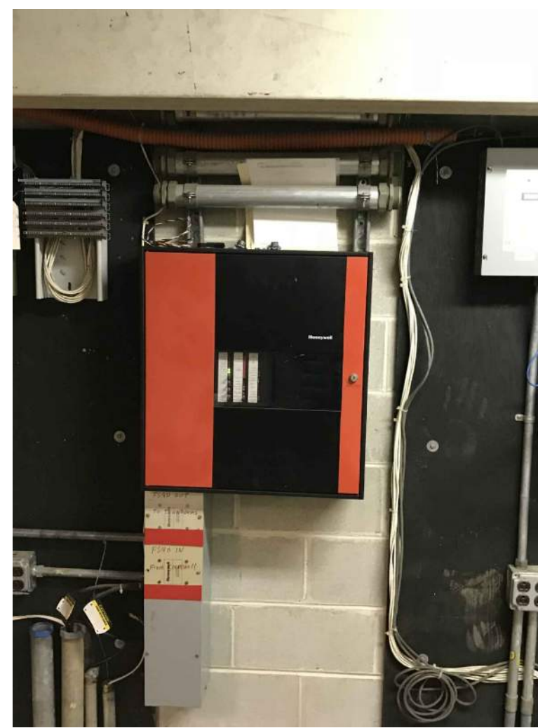
PHOTO C - EXISTING FIRE ALARM CONTROL PANEL Honeywell FS90 Addressable Fire Alarm Control Panel And Booster Panel With Exposed Conduit Located Within First Floor Electrical Room
