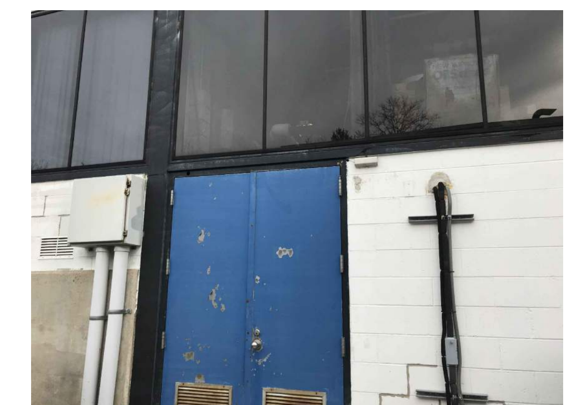
PHOTO F - EXISTING POINT OF ENTRY Location Of Existing Point Of Entry For Maintenance Building Pull Box Mounted On Building Exterior With Empty Conduit.
