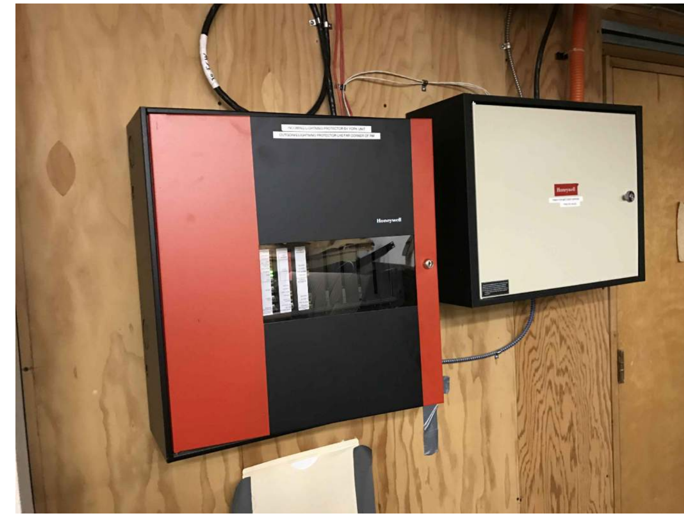
PHOTO A - EXISTING FIRE ALARM CONTROL PANEL Honeywell FS90 Addressable Fire Alarm Control Panel With Exposed Conduit Located Within Lower Level Storage Room
