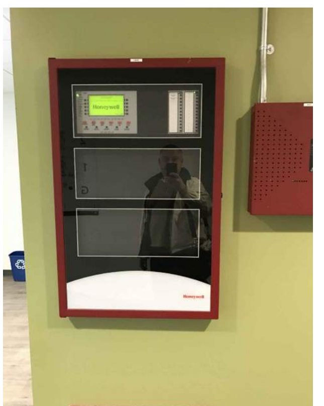
PHOTO A - EXISTING FIRE ALARM PANEL Existing Fire Alarm Control Panel Location
