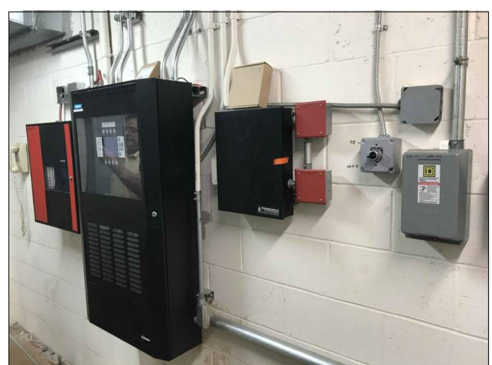
SCIENCE COMPLEX FACP Fiber Installed In The Science Complex Building Installed Per TCNJ Standards
