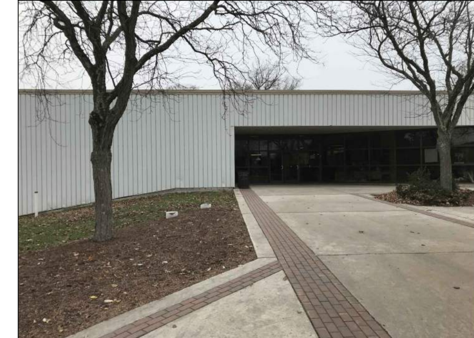
PHOTO A - RECREATION CENTER POE Area For New Recreation Center Point Of Entry And New Duct Bank. Route Includes Hardscapes Such As Brick And Concrete.
