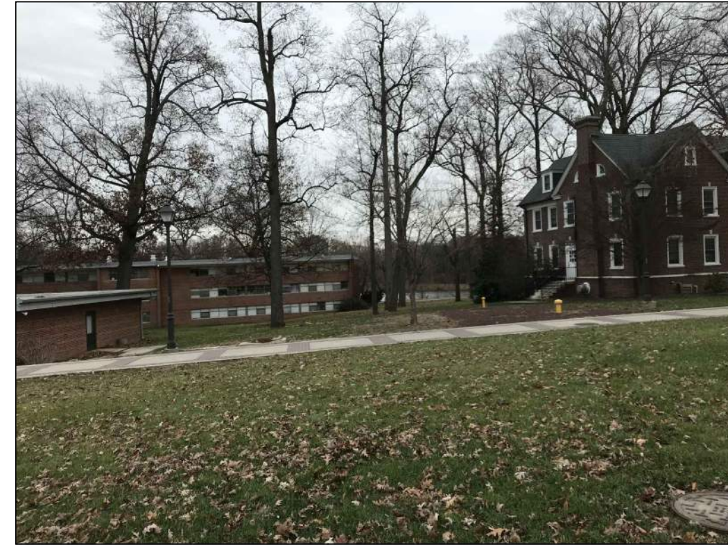
PHOTO E - NORTH EAB Location For New Manhole And Duct Bank Routing From New Manhole North Of EAB To Manhole 12C. Route Includes Hardscapes Such As Brick And Concrete.
