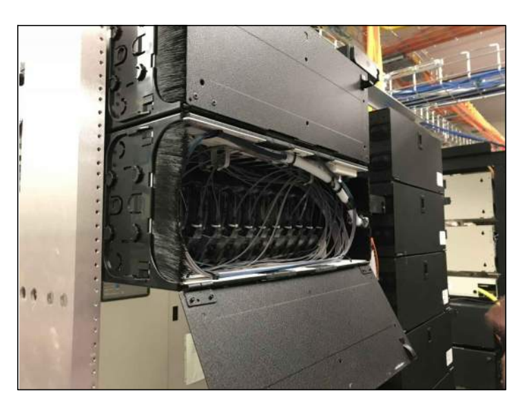
RACK MOUNTED CABINET
