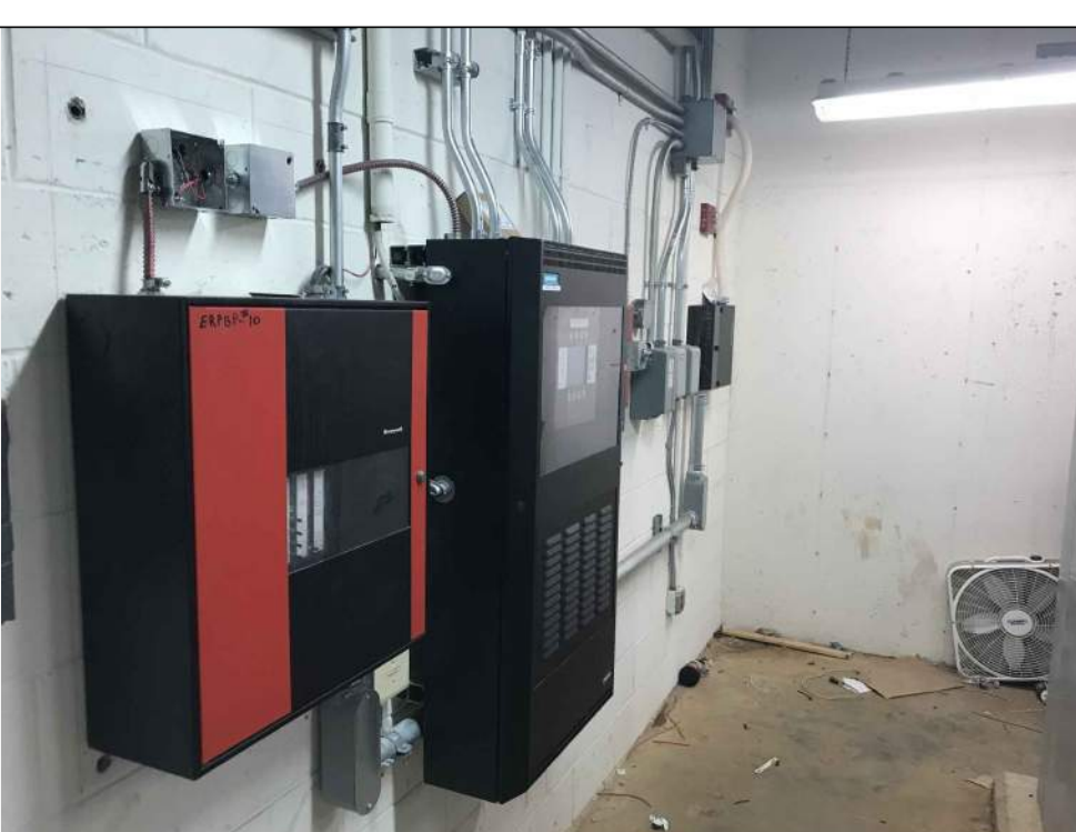
SCIENCE COMPLEX FACP Fiber Installed In The Science Complex Building Installed Per TCNJ Standards
