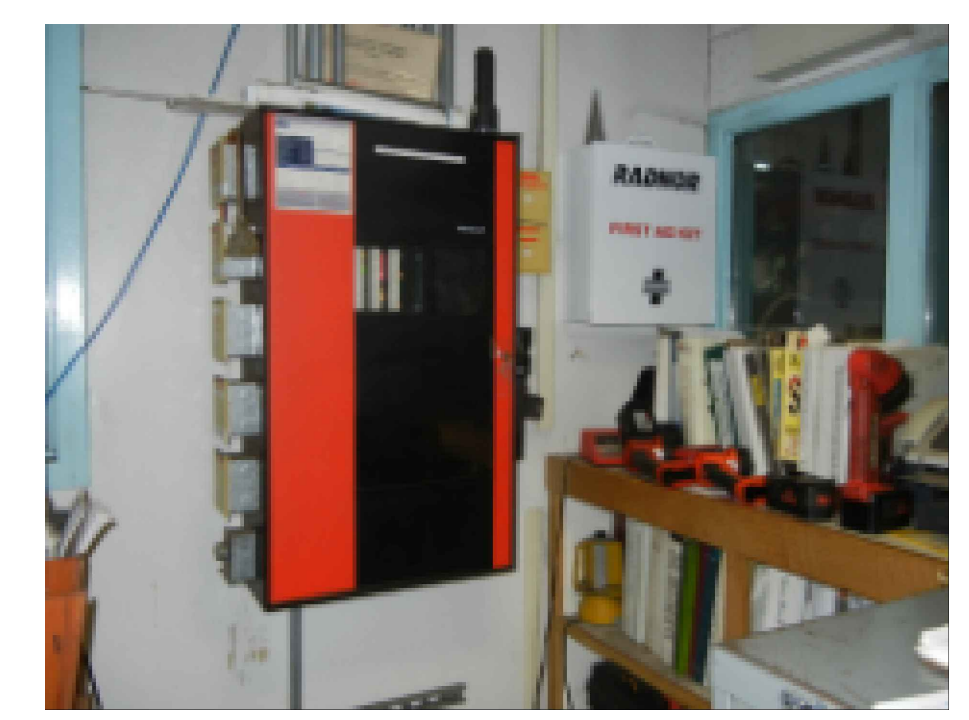
PHOTO A - EXISTING FIRE ALARM PANEL Existing Fire Alarm Control Panel Location On Control Room Wall.
