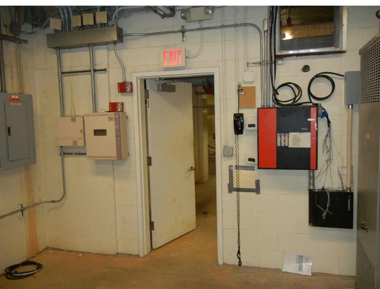
PHOTO D - EXISTING FIRE ALARM PANEL Existing Fire Alarm Control Panel
