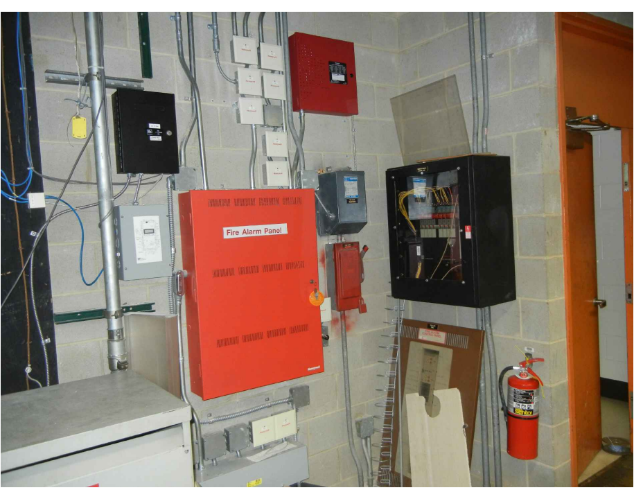
PHOTO C - EXISTING FIRE ALARM PANEL Existing Fire Alarm Control Panel Location In Electrical Room.
