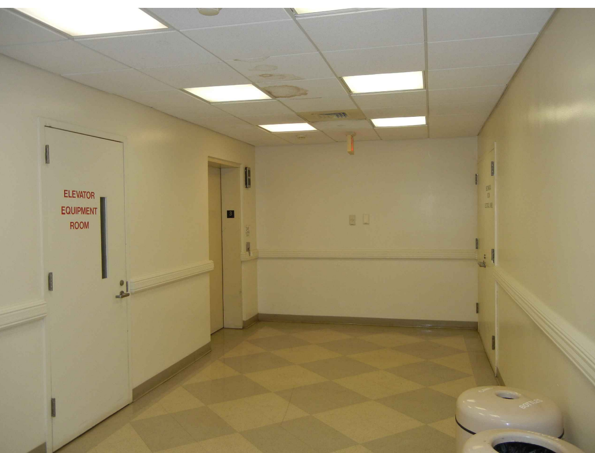
BUILDING CEILINGS Drop Ceilings Located Throughout The Building. Route Fiber Pathway Above Existing Drop Ceilings
