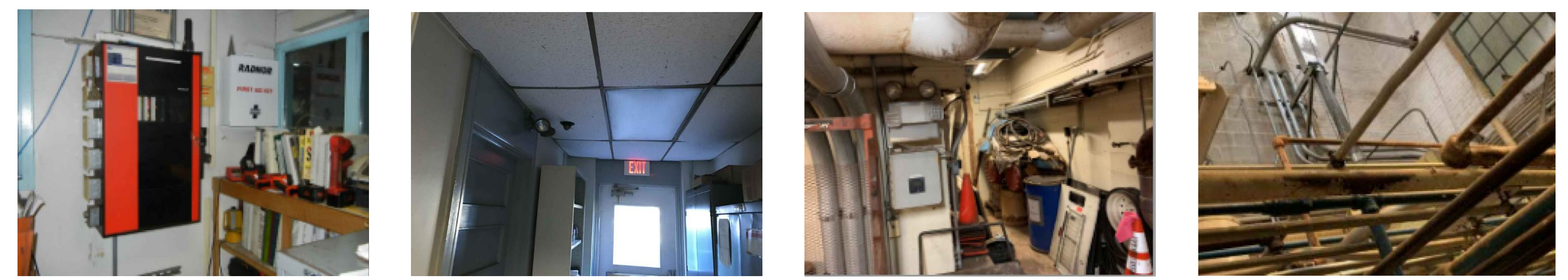
PHOTO A - EXISTING FIRE ALARM PANEL Existing Fire Alarm Control Panel Location On Control Room Wall. PHOTO B - EXISTING CEILING CONDITIONS Route Fiber Pathway Above Drop Ceiling Located Throughout First Floor PHOTO C - BASEMENT CEILING AND POE Route Fiber Pathway As High As Possible Amongst The Other Mechanical Infrastructure In Basement Area. PHOTO D - BOILER ROOM VAULTED CEILING Route Fiber Pathway Along Wall Entering From Corridor Ceiling And Exiting Above Control Room Ceiling ( Photo Above Shows Existing Conduits Entering Control Room Ceiling Area ). New Fiber Pathway To Be Routed Similar To Existing Routing
