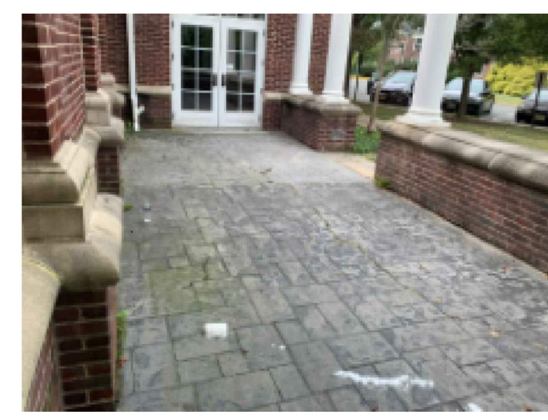
PHOTO B - PATIO AREA Install New Exterior Fiber Pathway Below Existing Stamped Concrete Patio. Existing Sidewalk And Entire Stamped Concrete Patio To Be Replaced To Match Existing.
