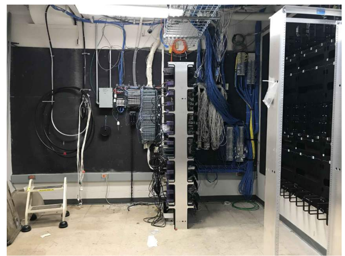
PHOTO B - EXISTING MDF ROOM Existing MDF in First Floor Electrical Room
