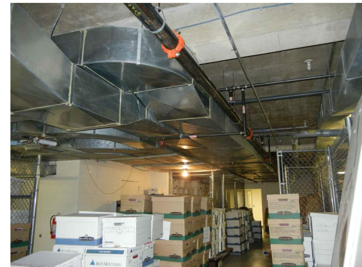
PHOTO B - BASEMENT EXPOSED CEILING Exposed Ceiling In The Basement
