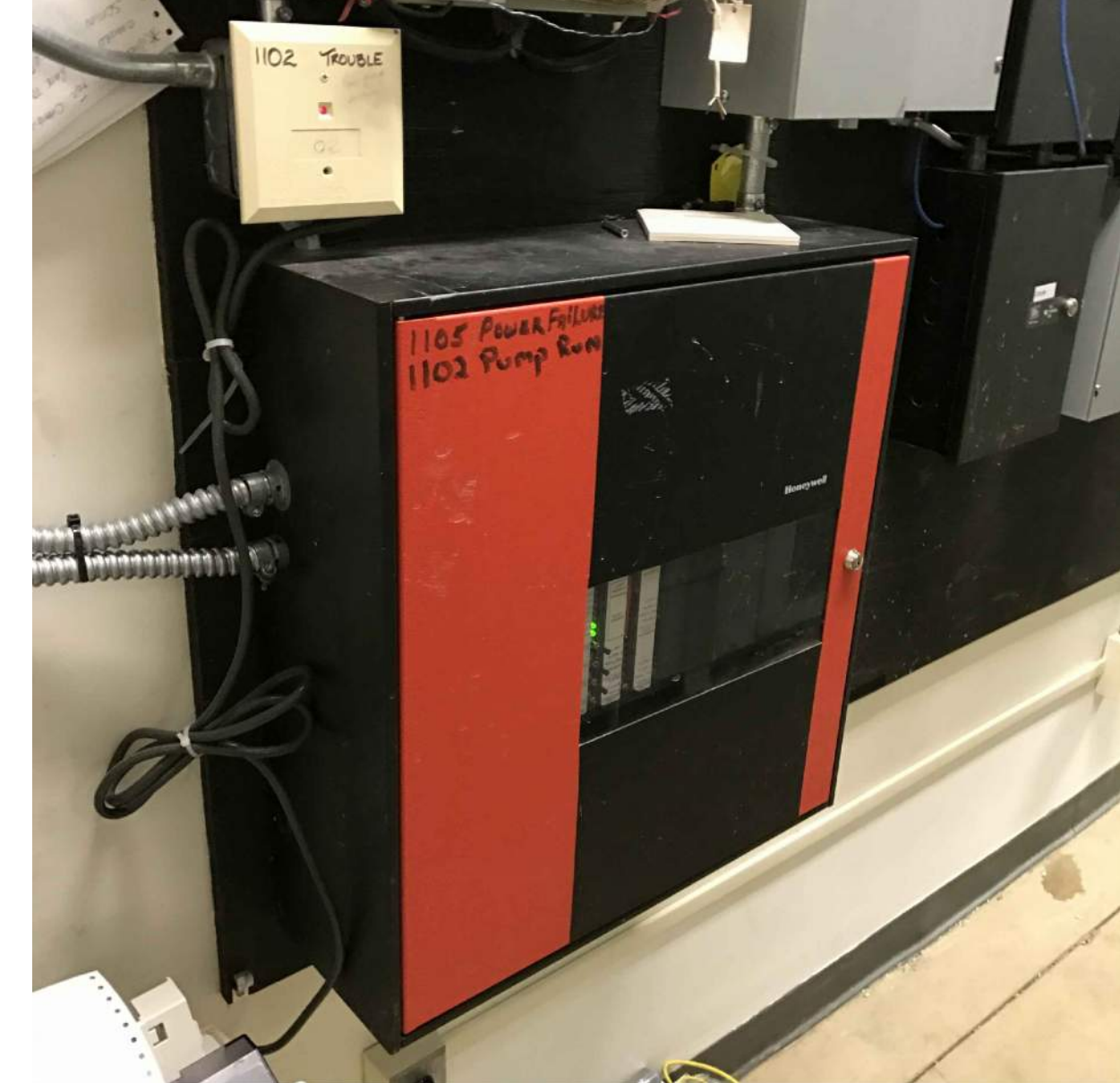
PHOTO B - FIRE ALARM CONTROL PANEL Existing Fire Alarm Control Panel
