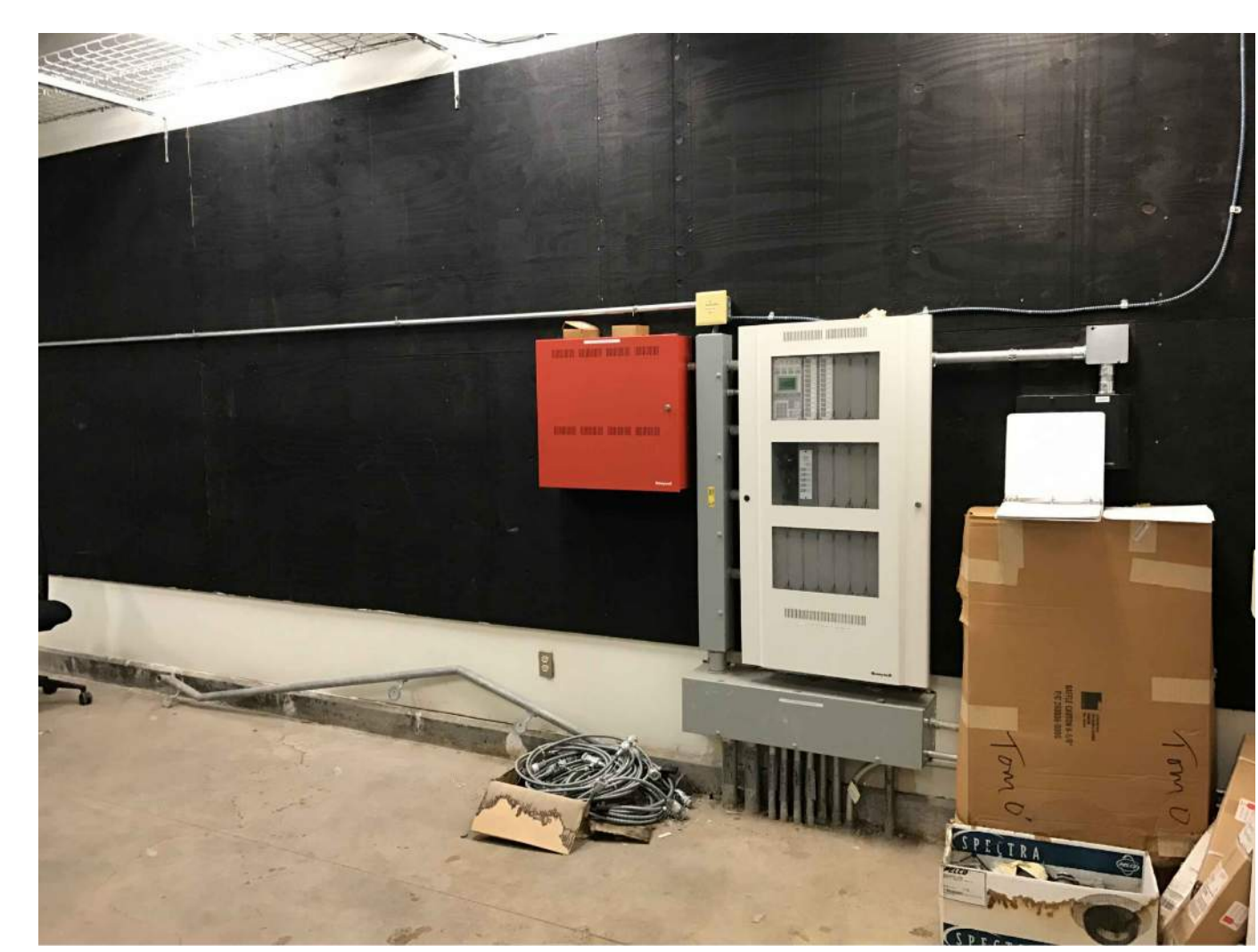
PHOTO A - FIRE ALARM CONTROL PANEL Fire Alarm Control Panel And Booster Panel With Exposed Conduit Located Within Lower Level Electrical Room
