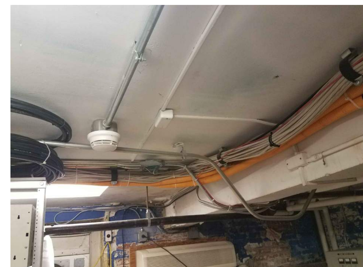
PHOTO D - BASEMENT CEILING Existing Ceiling Space In Basement MDF.
