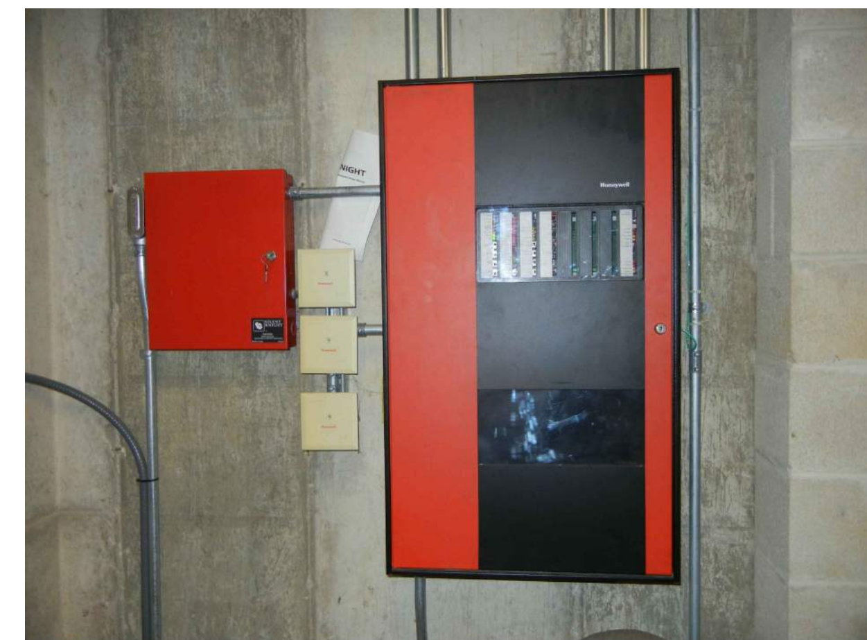
PHOTO C - EXISTING FIRE ALARM PANEL Existing Fire Alarm Control Panel Location
