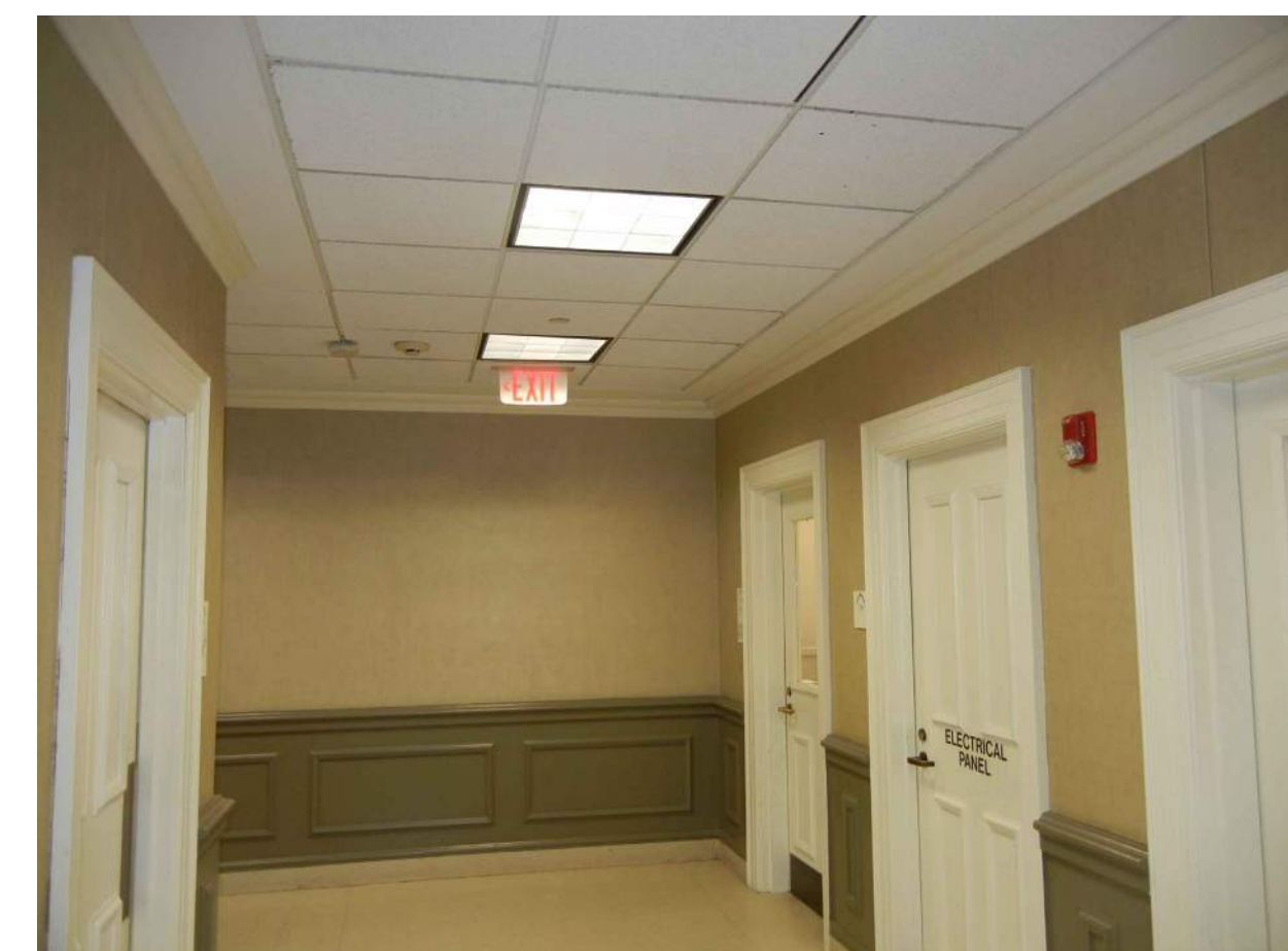
PHOTO D - LOWER LEVEL CEILING Route Above Existing Lower Level Drop Ceiling
