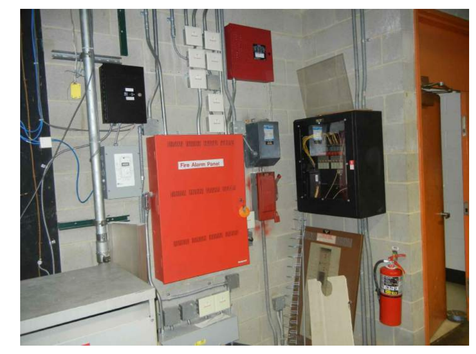
PHOTO C - EXISTING FIRE ALARM PANEL Existing Fire Alarm Control Panel Location In Electrical Room.
