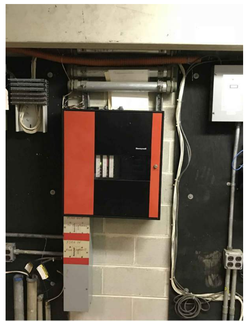
PHOTO C - EXISTING FIRE ALARM CONTROL PANEL Honeywell FS90 Addressable Fire Alarm Control Panel And Booster Panel With Exposed Conduit Located Within First Floor Electrical Room
