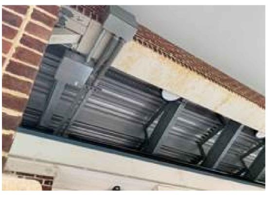
PHOTO D - CONDUIT ROUTING Route New Fiber Pathway Similar To The Existing Conduit Runs That Are Routed Under The Second Floor Press Box And Up Into The Mechanical Room.
