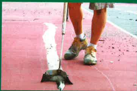
STEP 1: Fill cracks up to 4 inches wide
