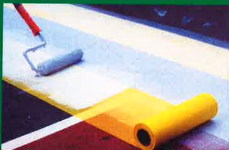
STEP 7: Install yellow ARMOR ® mesh
