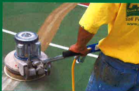
STEP 2: Sand flush to surface
