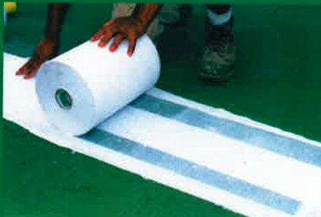
STEP 5: Install narrow ARMOR ® fabric
