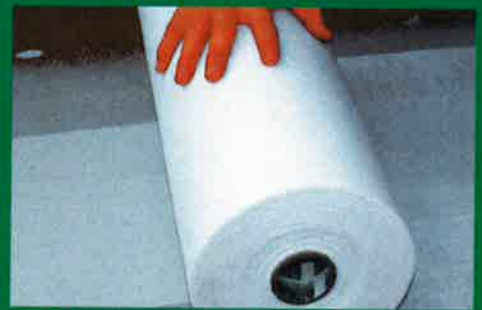
STEP 6: Install wide ARMOR ® fabric
