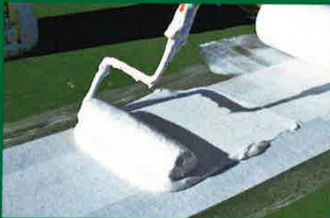
STEP 4: Apply liquid adhesive
