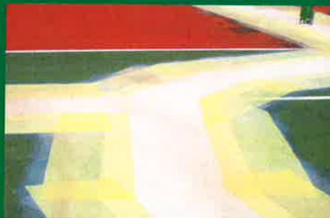
STEP 8: Finished...ready to color coat!
