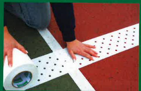
STEP 3: Apply ARMOR ® release tape
